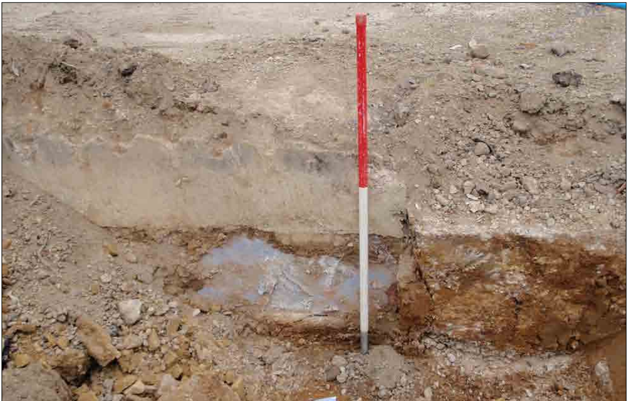
Plate 4: Trench 11 looking north showing reinforced concrete rafts and concrete pillar
