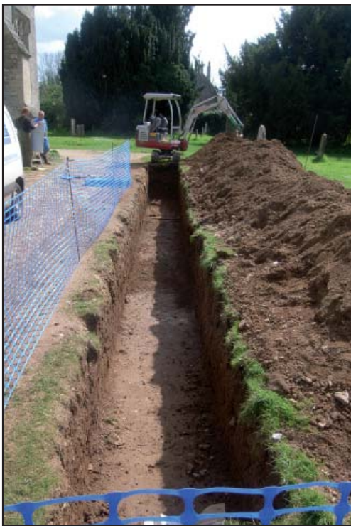
Plate 2: North-south trench, (looking towards the south)
