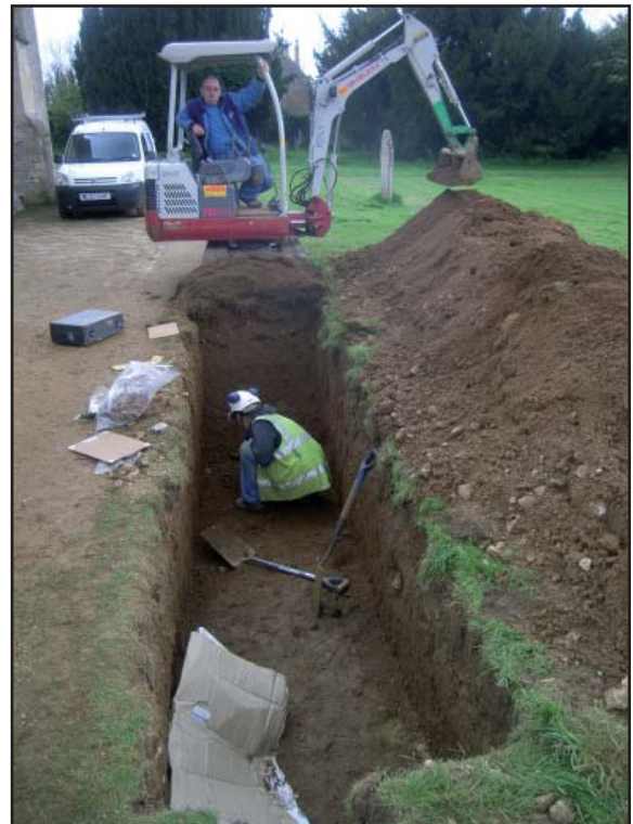
Plate 3: Working shot of north-south trench, (looking towards the south)
