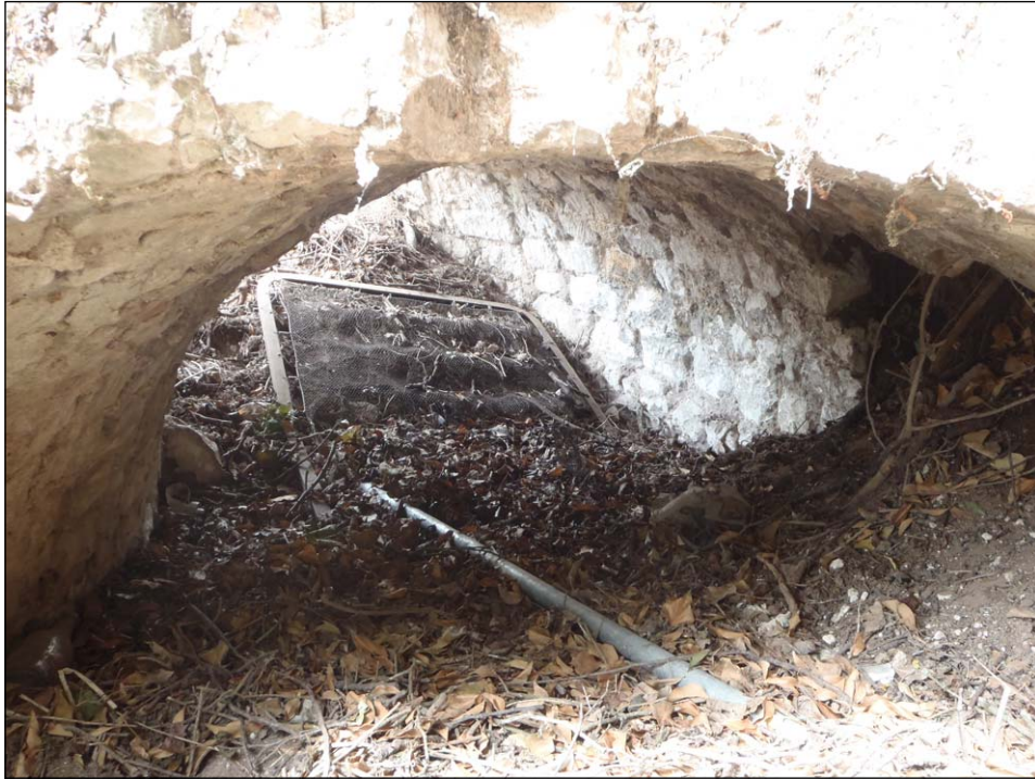
Plate 5: Internal view of kiln structure (from south)
