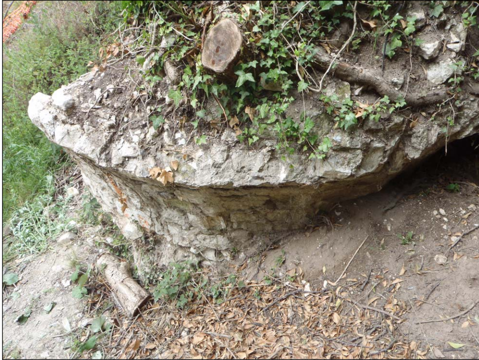
Plate 7: Detail of arch on southern side of kiln structure (from south)
