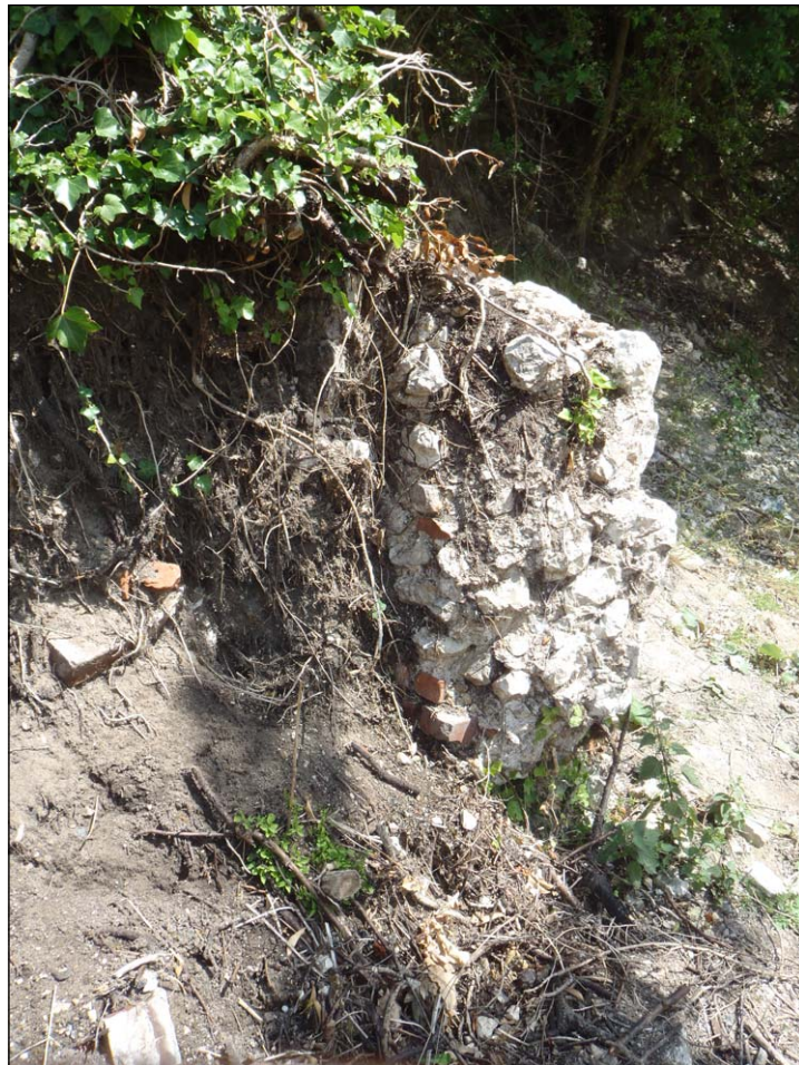
Plate 8: Detail of arch on southern side of kiln structure (from north west)
