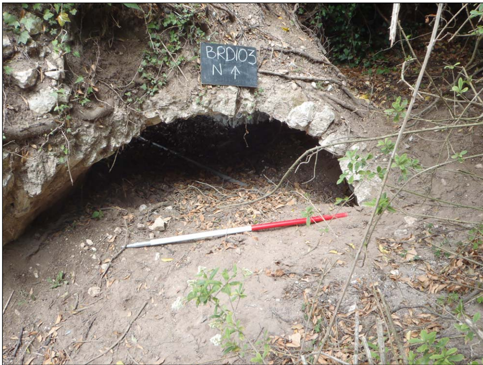
Plate 4: Detail shot of kiln opening (from south)
