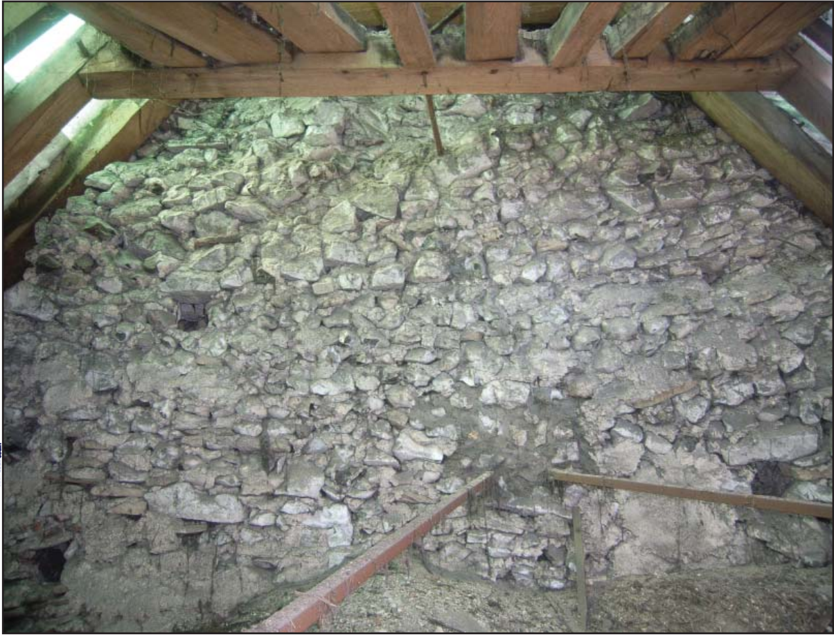
Plate 25: East face of wall between semi-circular end and main roof
