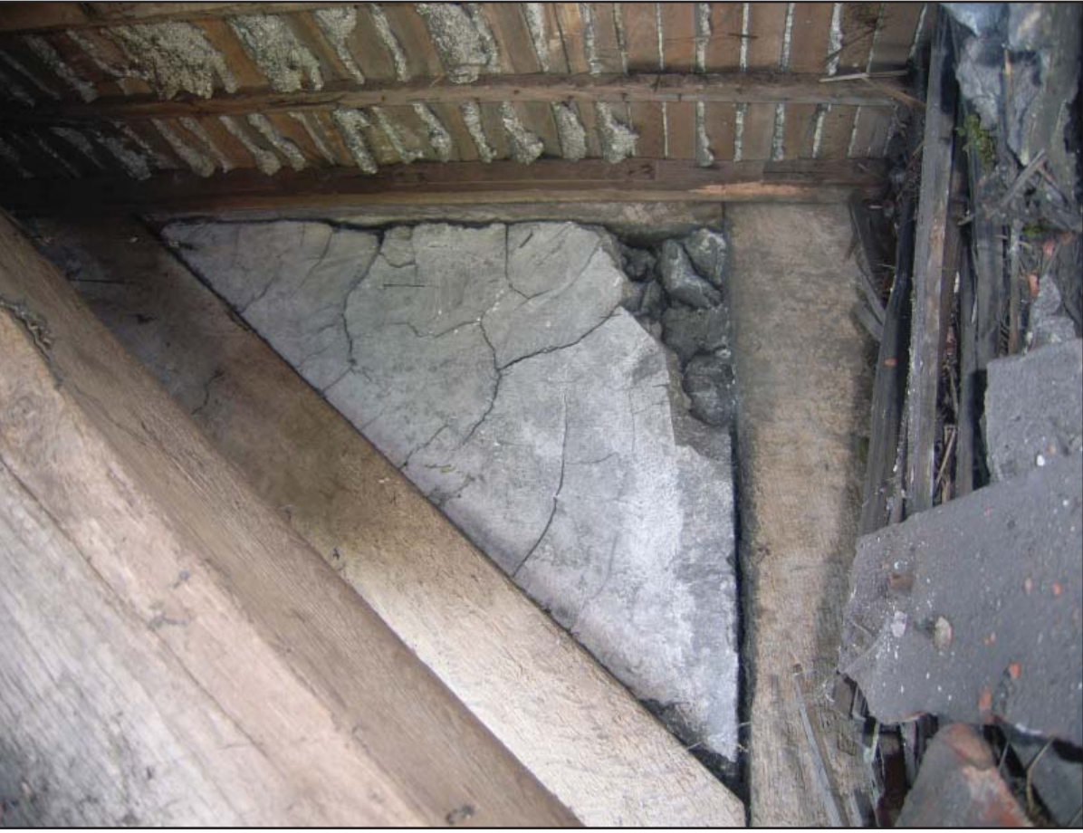
Plate 17: Plastered wall at east end of main roof
