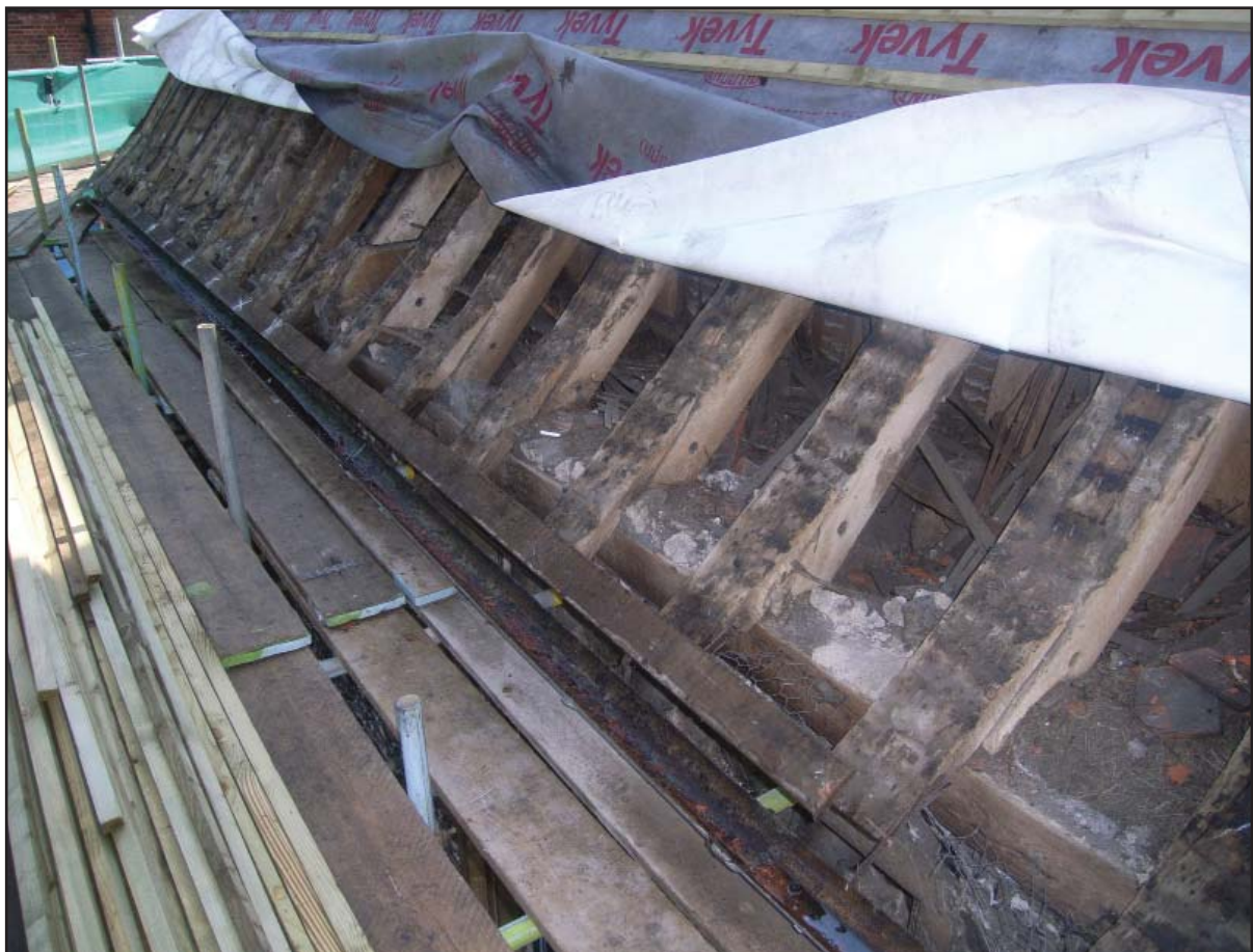
Plate 10: Rafter feet exposed on north side of roof
