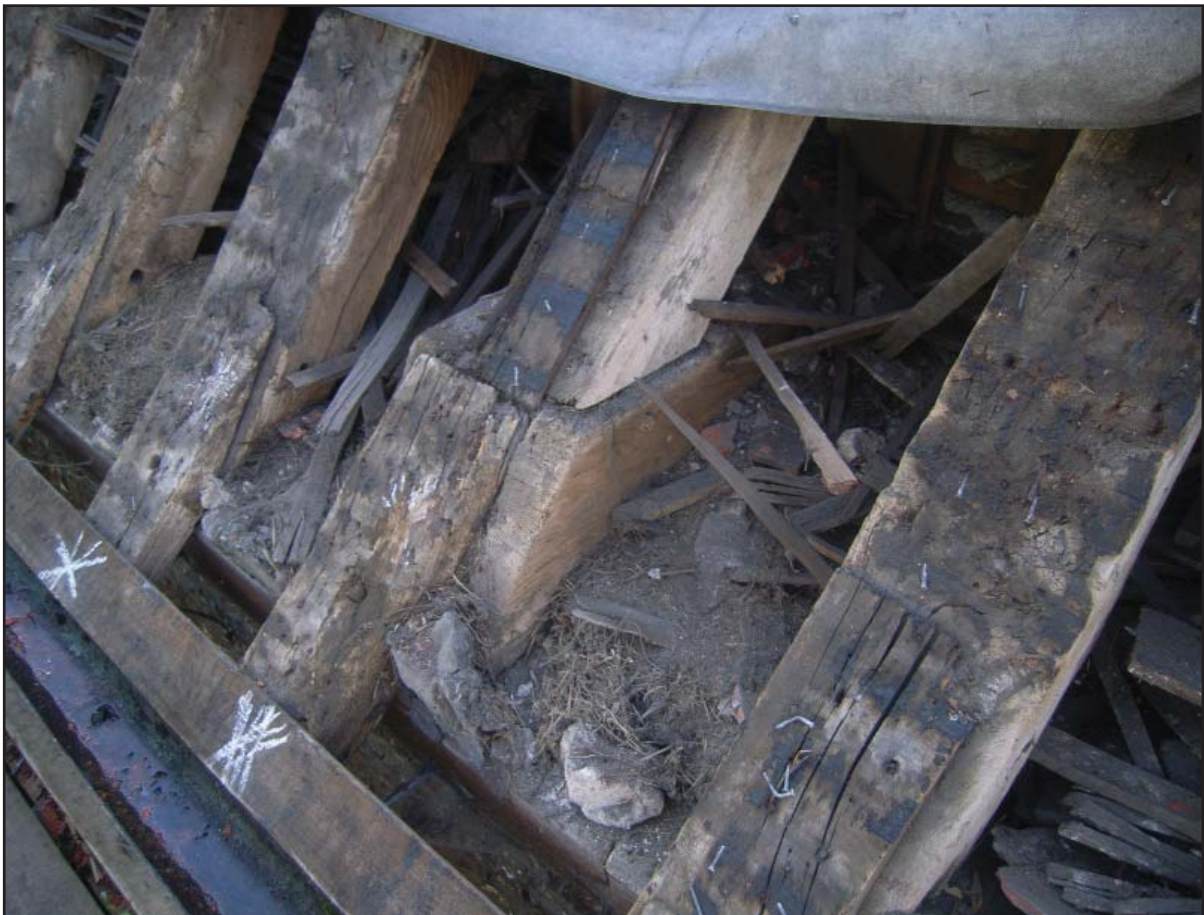
Plate 12: Tie-beam towards centre of chapel roof
