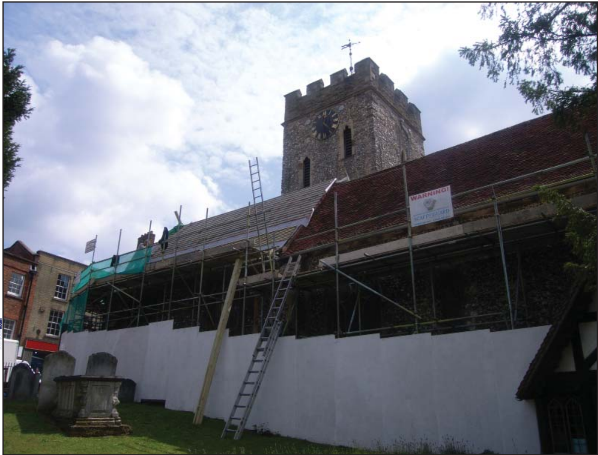
Plate 9: St Marys from the NW during works
