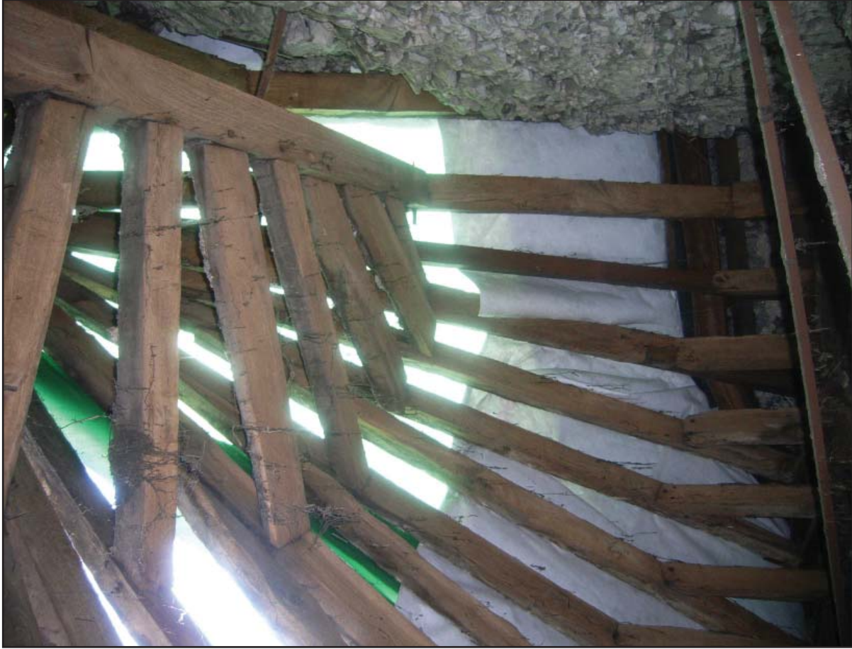
Plate 20: Roof at semi-circular east end
