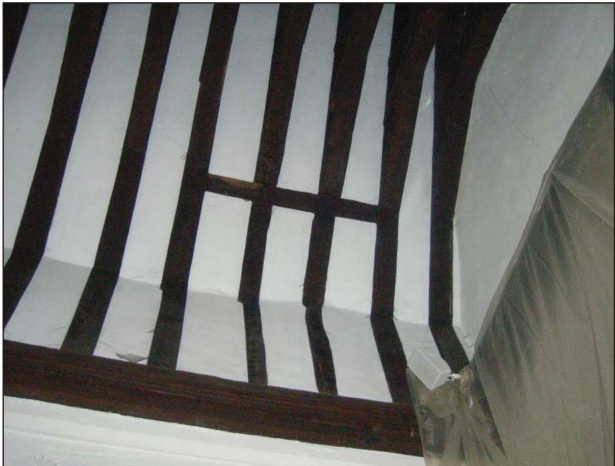
Plate 28: Trimmer visible from beneath in chapel
