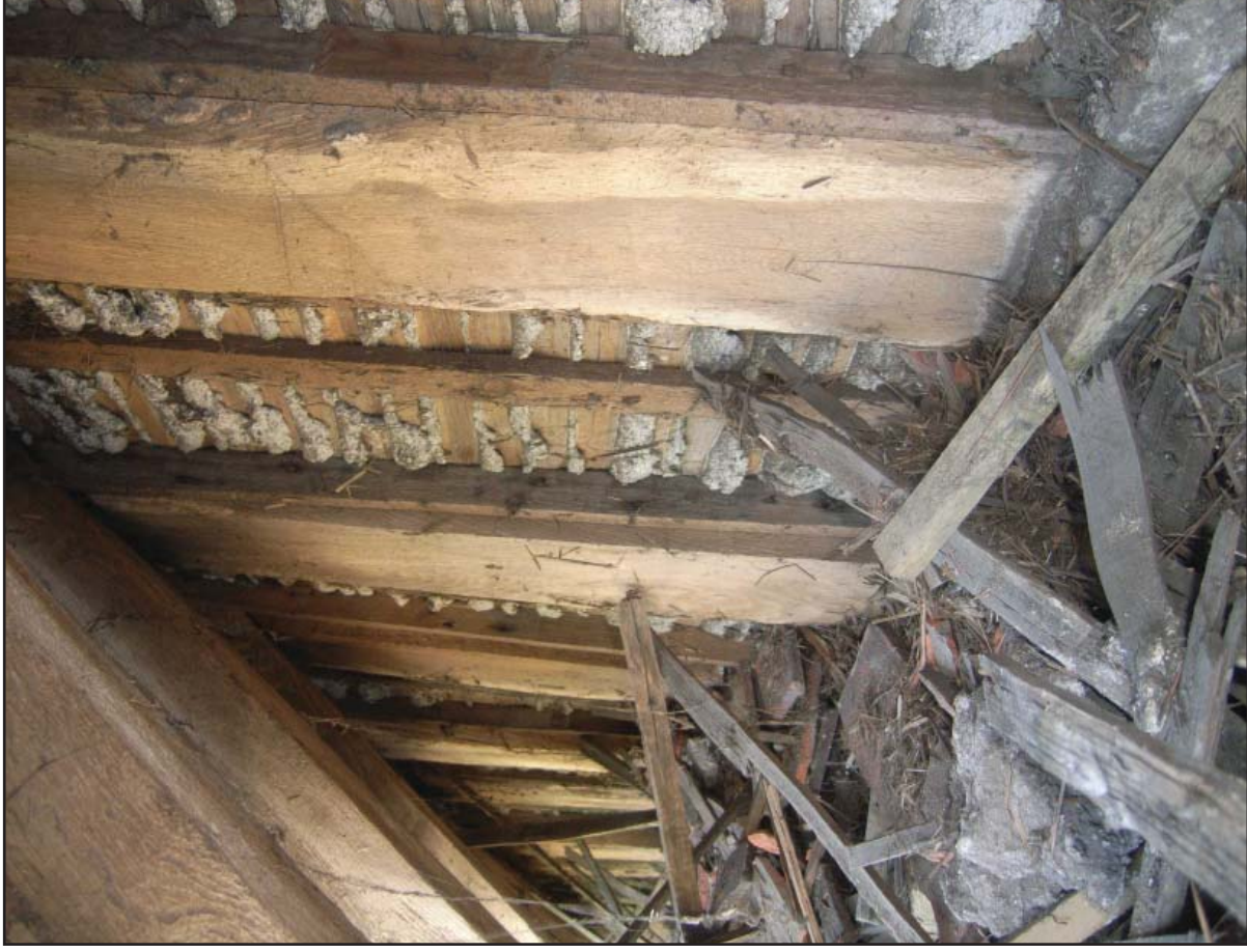
Plate 19: Ashlar studs along main part of roof
