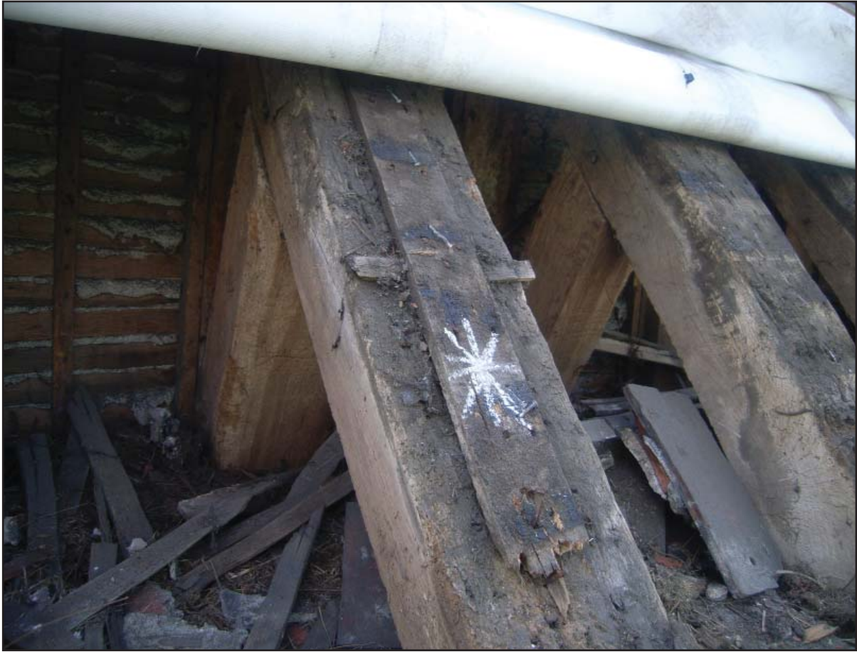
Plate 15: Rafter feed towards east end of main roof
