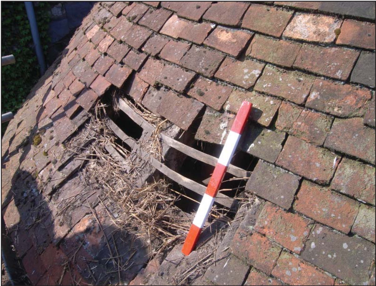
Plate 3: St. Mary's Church roof, showing straw packing
