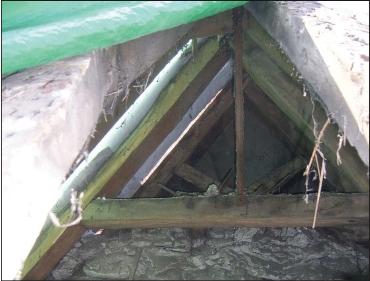
Plate 23: Roof apex at east end
