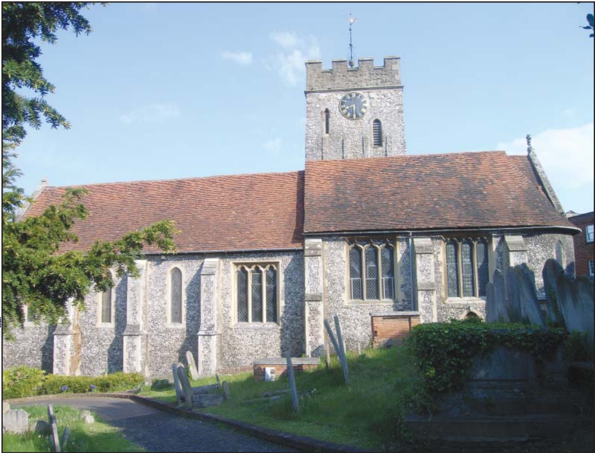
Plate 1: St. Mary's Church, general view
