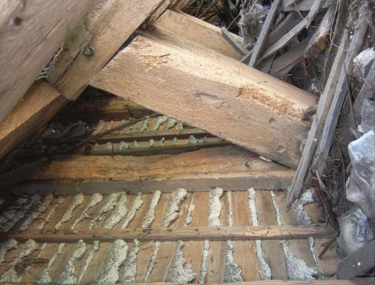
Plate 18: Strut supporting trimmer from former light
