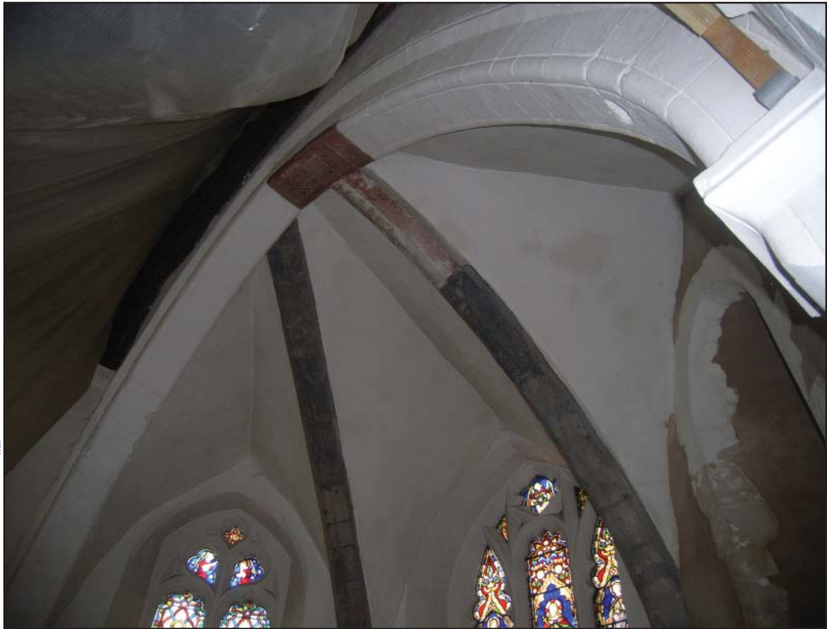
Plate 27: Vaulting in St John's Chapel
