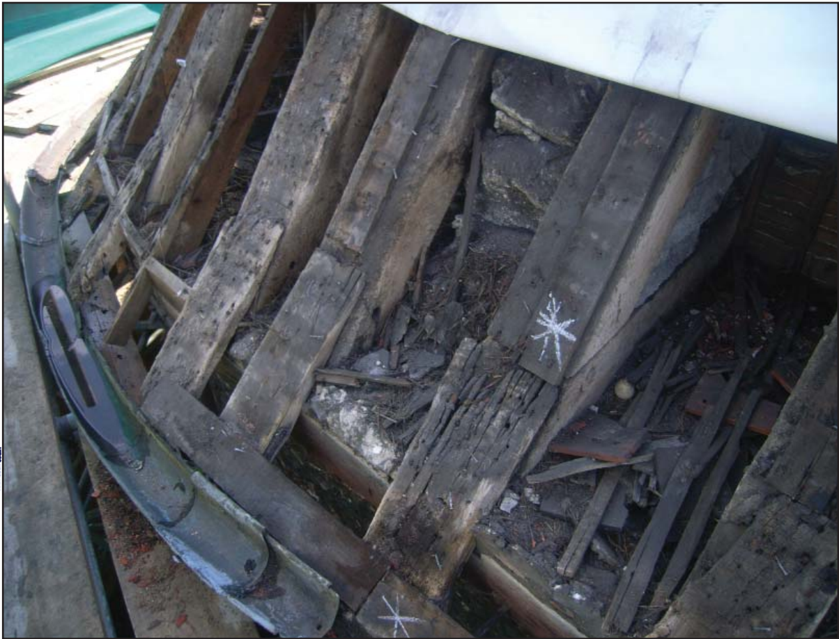
Plate 13: Rafter feet at semi-circular east end
