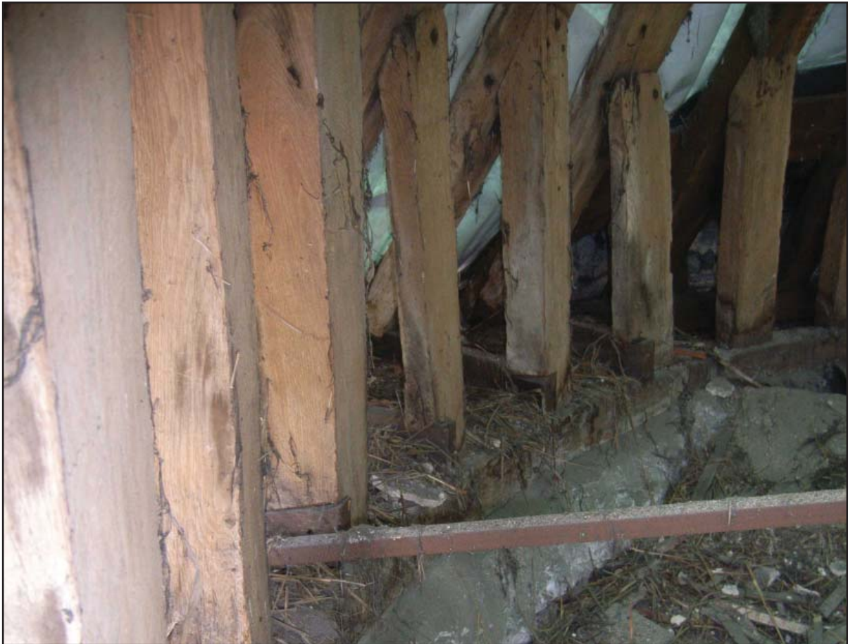
Plate 24: Detail of studs in semi circular east part of roof
