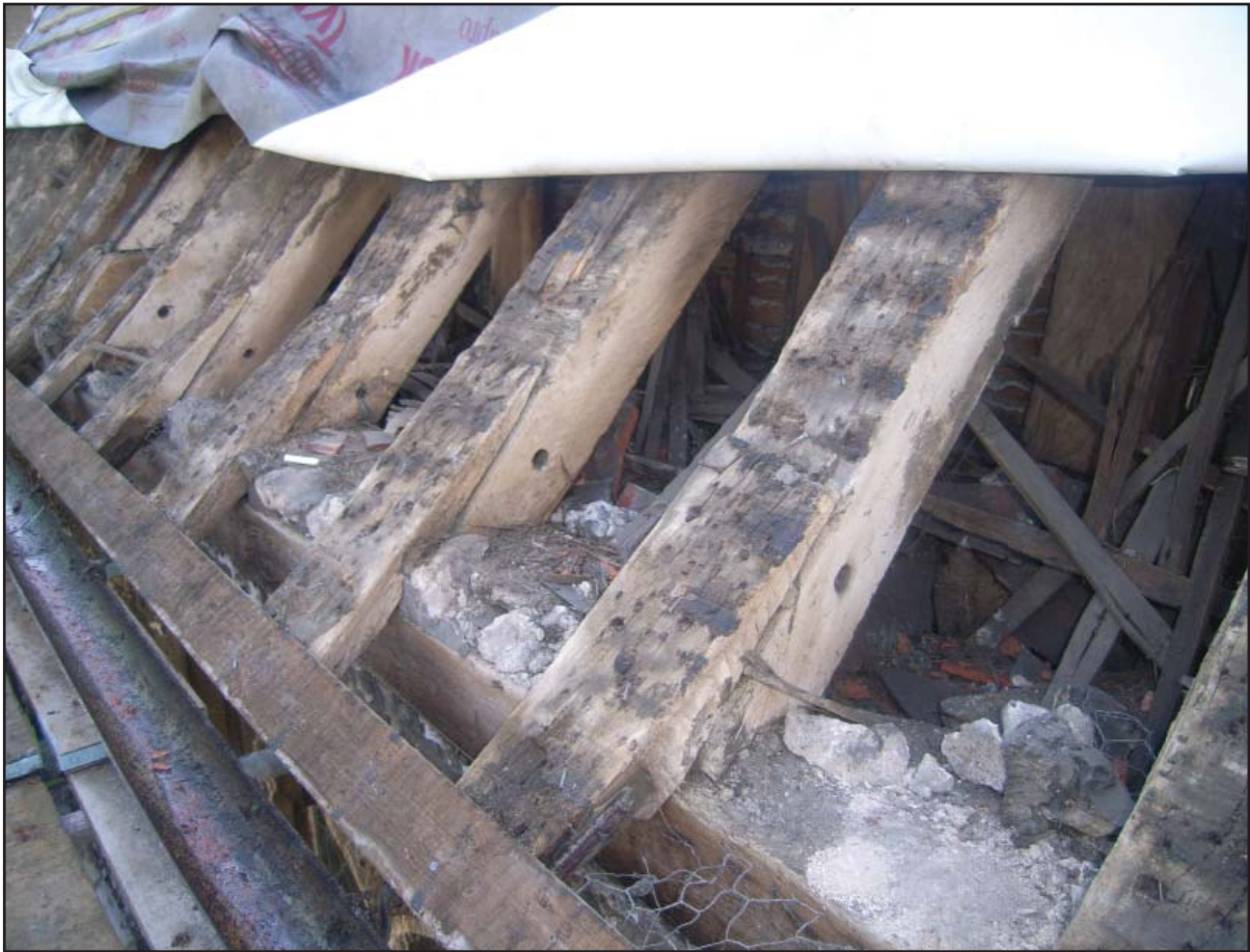
Plate 11: Rafter feet exposed on north side of roof
