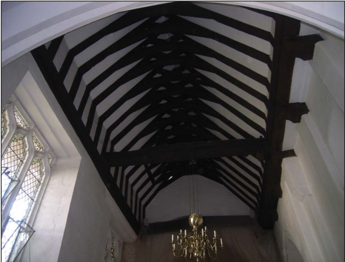
Plate 26: Underside of roof
