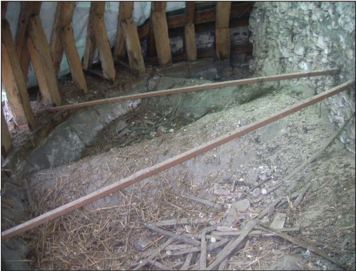
Plate 21: Tie rods in roof at east end
