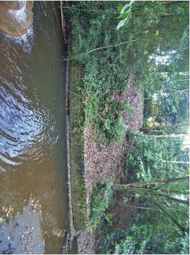
Plate 2: West wall of Southern inlet, showing subsidence
