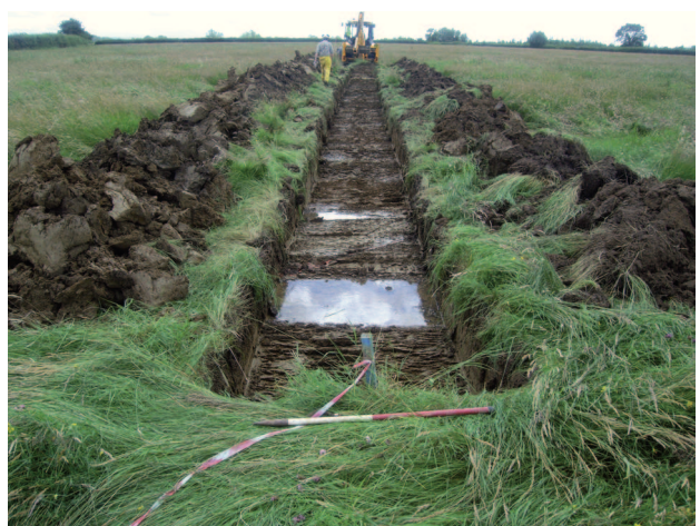
South-West facing photograph of Trench 6
