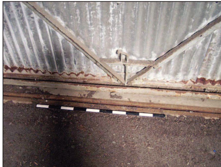
Plate 14: Detail of wall in south shed
