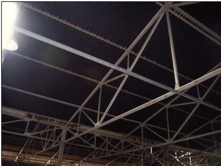
Plate 11: Roof trusses in south shed
