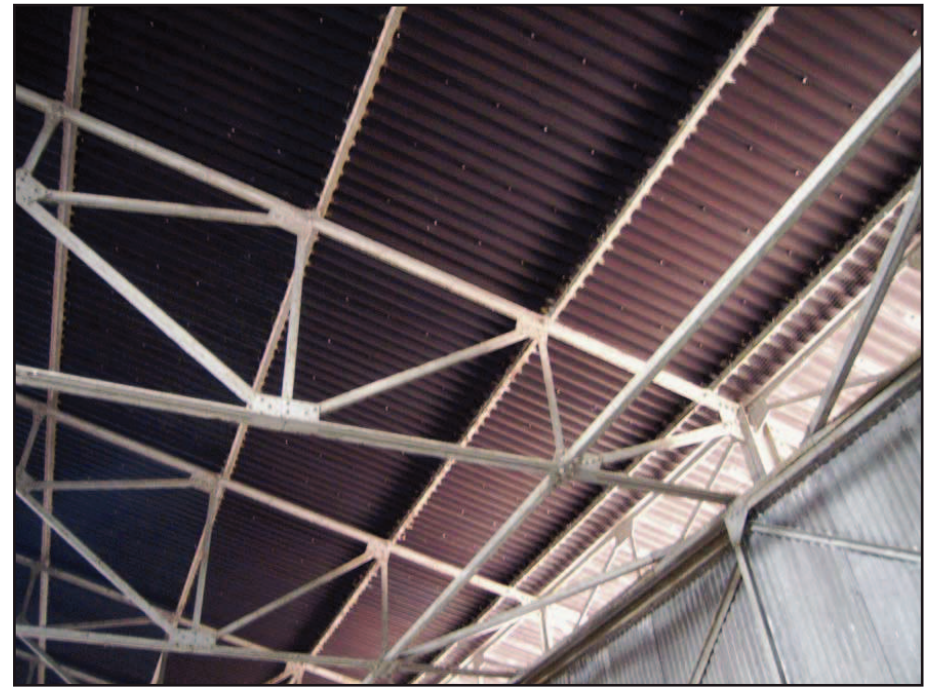
Plate 16: Detail of truss in south shed
