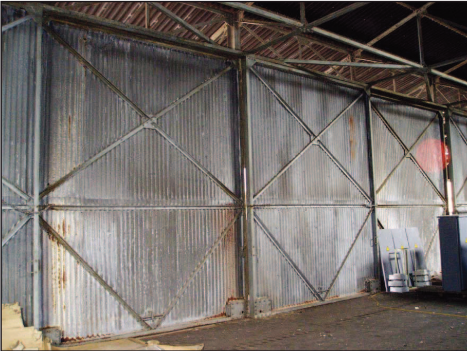
Plate 7: Wall frame in south shed
