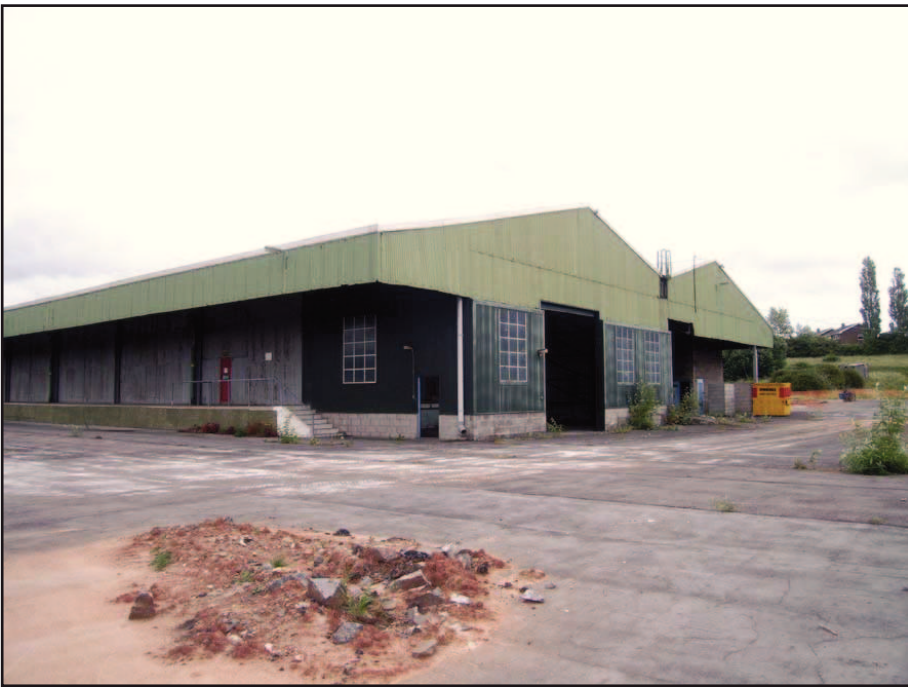
Plate 5: South end of north shed
