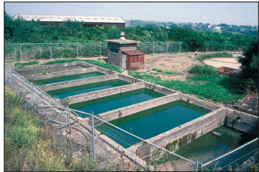
Plate 6: Settling tanks in the sewerage works
