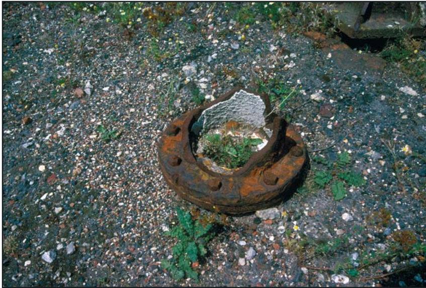
Plate 11: Section of pipe
