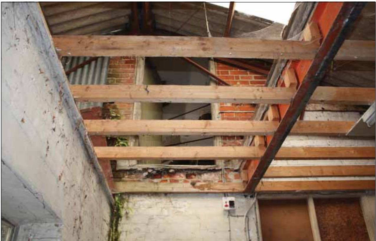
Plate 18: First floor loading door on former external wall of bakehouse, as viewed from “office”/G4
