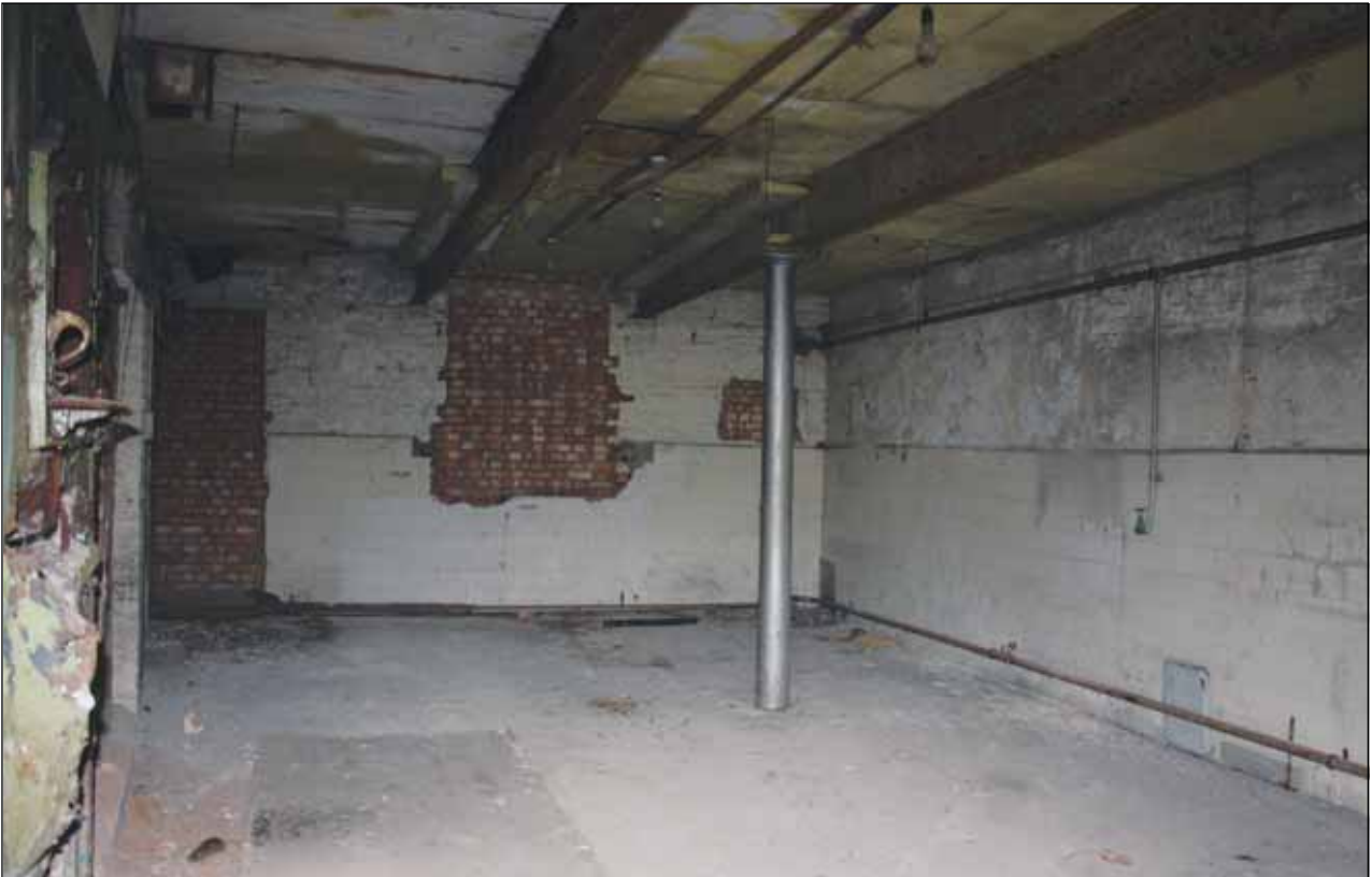
Plate 21: General room view of ground floor of bakehouse
