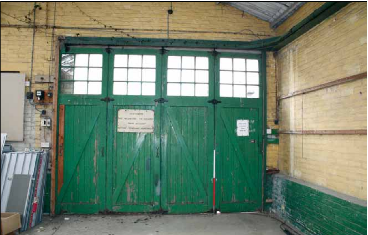
Plate 6: Internal view of main entrance doors to auction house
