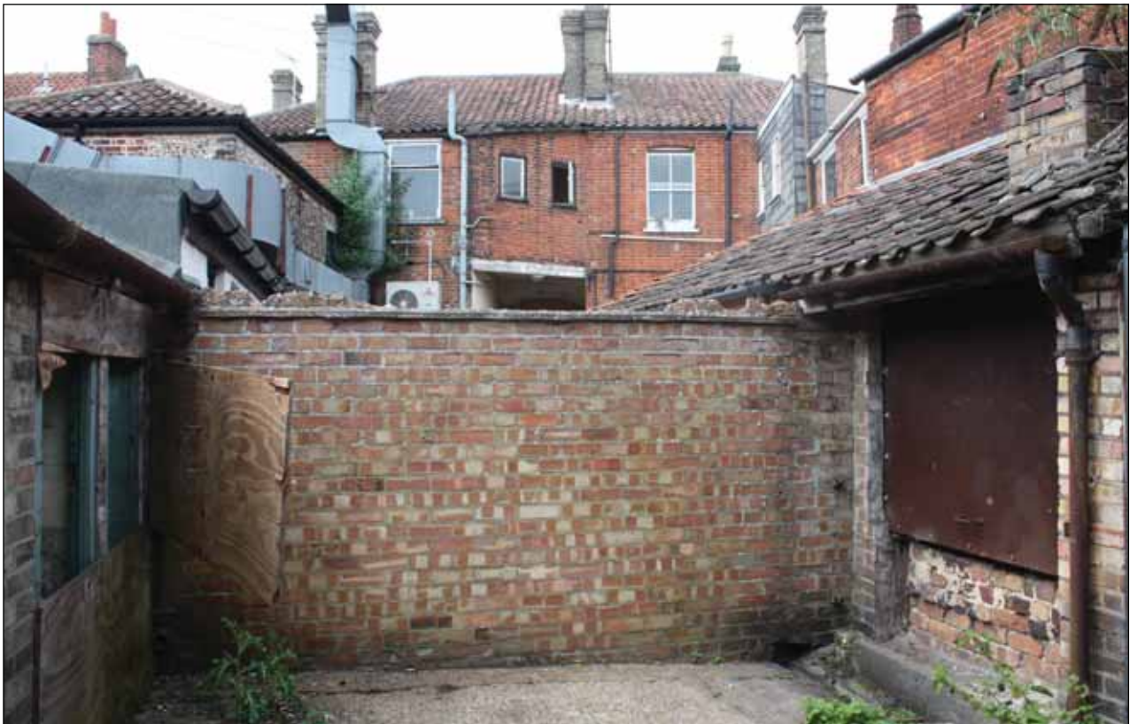
Plate 37: Boundary wall in external courtyard
