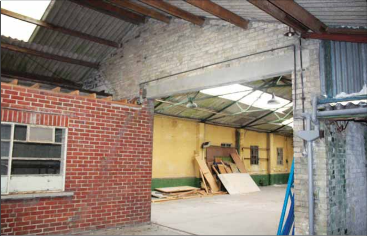
Plate 19: Western elevation of auction house as viewed from inner courtyard
