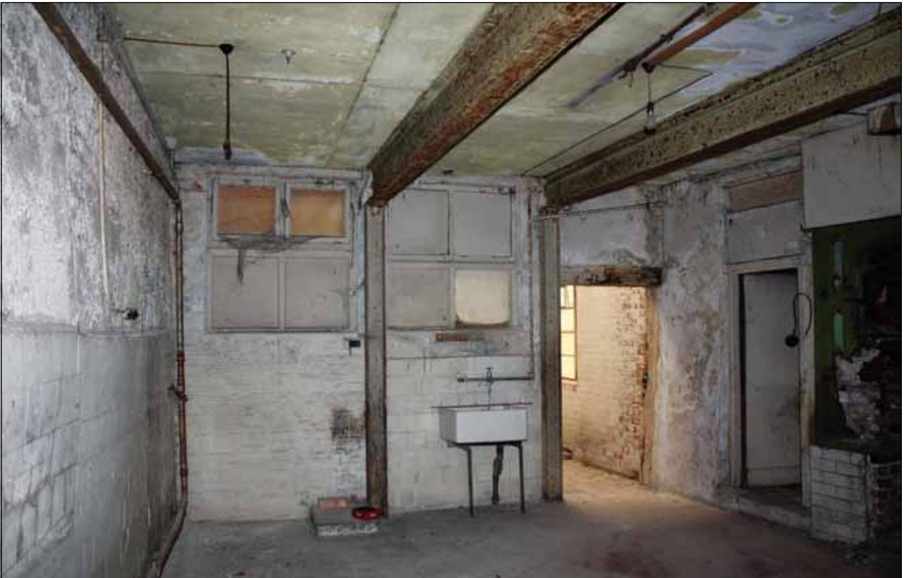
Plate 20: General room view of ground floor of bakehouse
