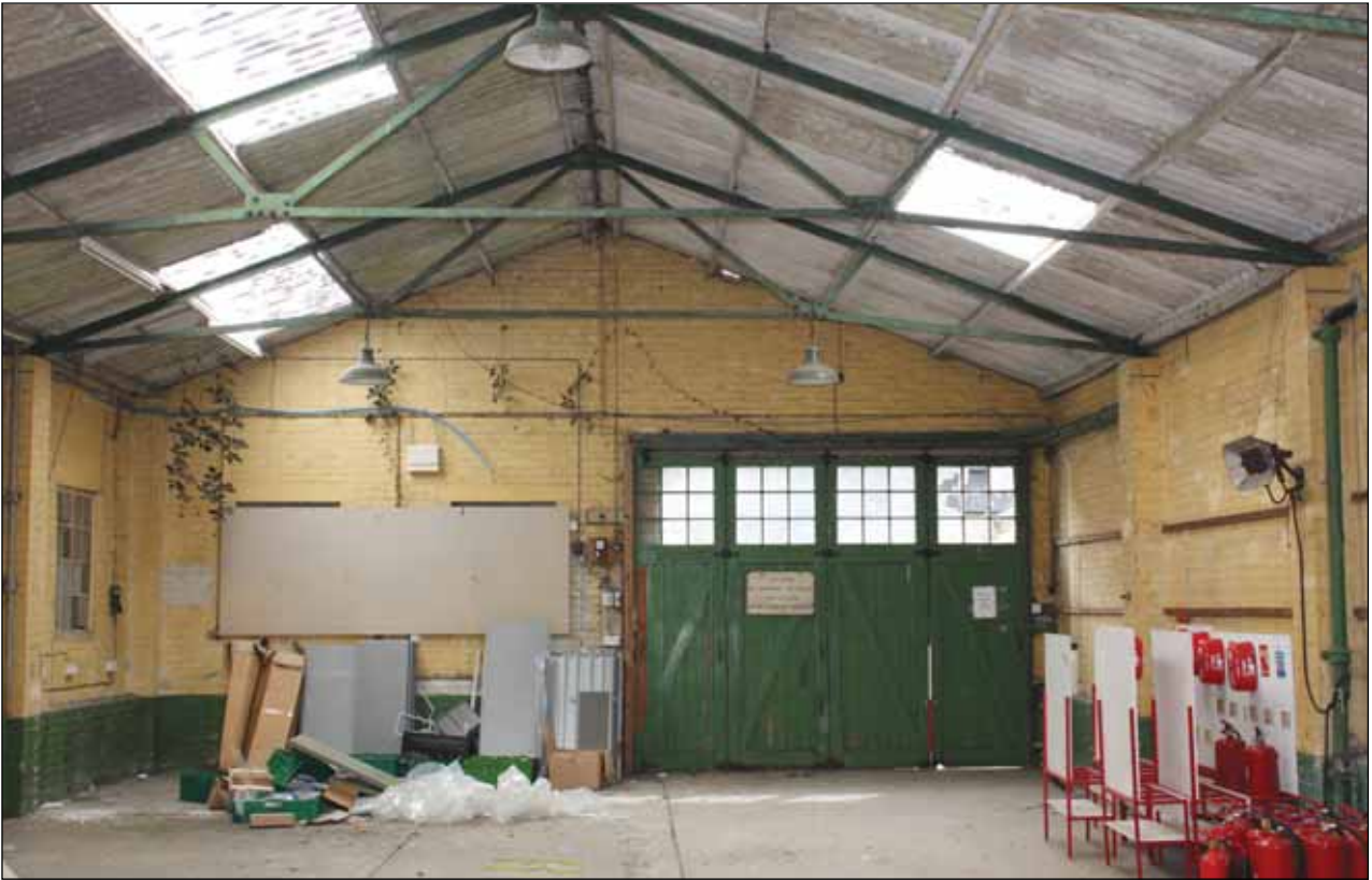
Plate 5: Internal view of auction house
