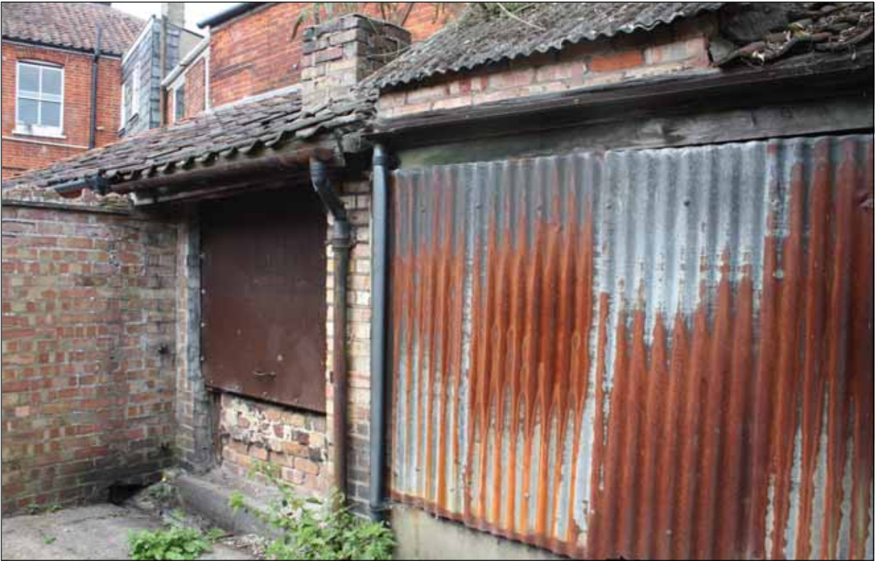
Plate 27: External view of Building 3
