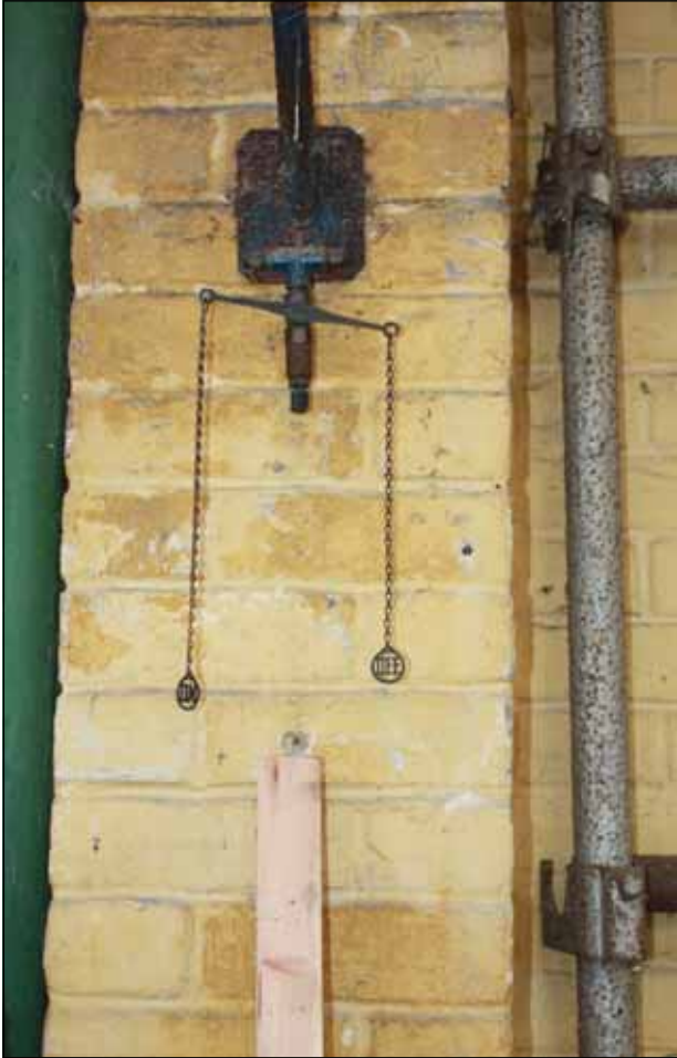
Plate 11: Detail of former gas lamp
