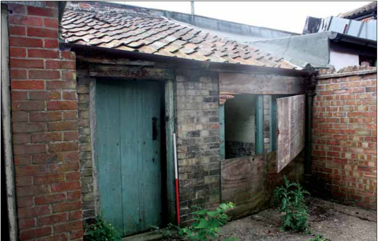
Plate 33: Building 5 as viewed from external courtyard
