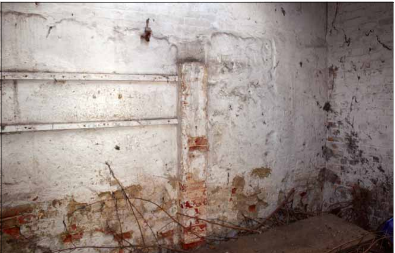
Plate 36: Detail of Brick buttress and possible blocked-up door, Building 5
