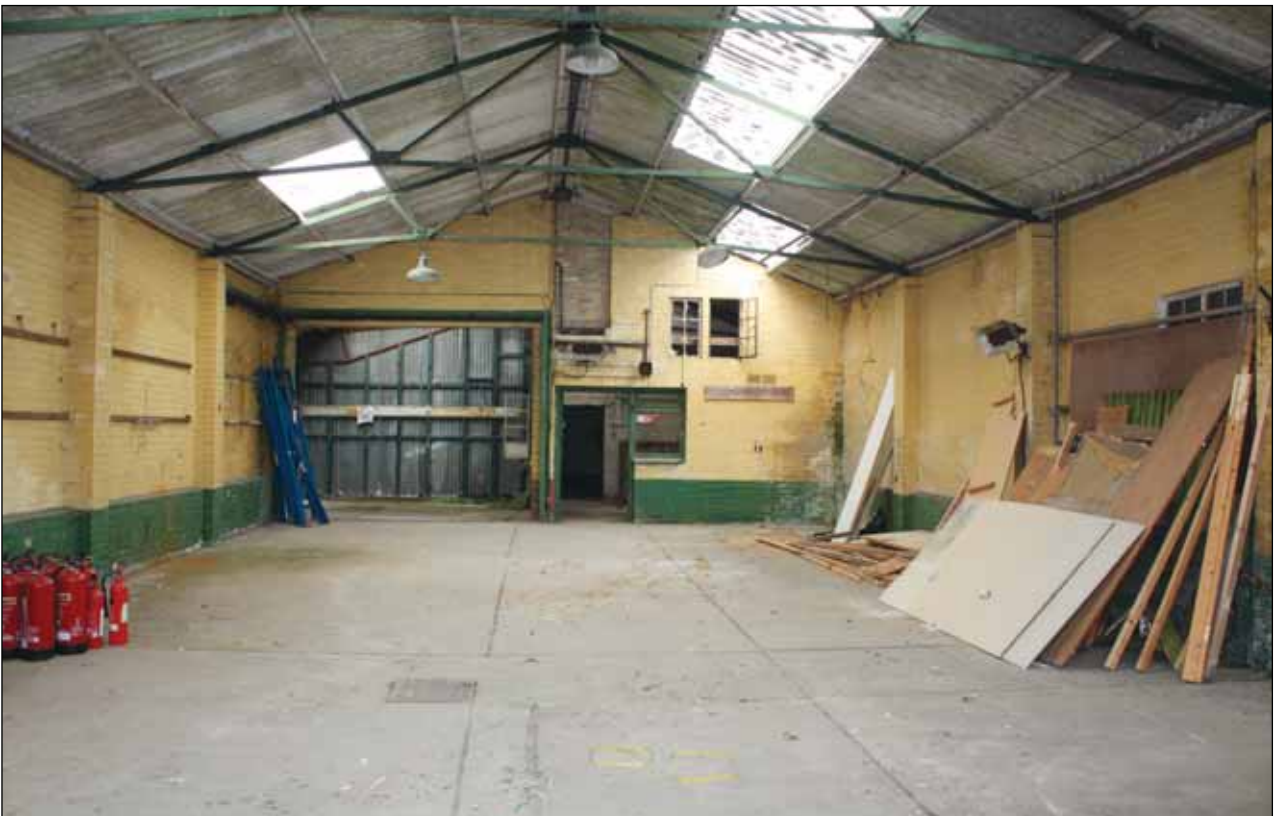
Plate 4: Internal view of auction house
