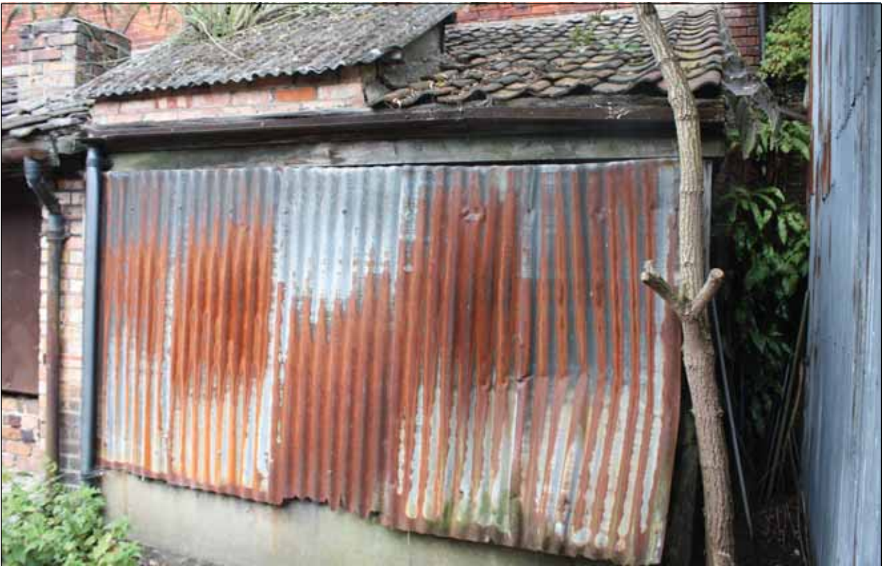
Plate 28: External view of Building 3
