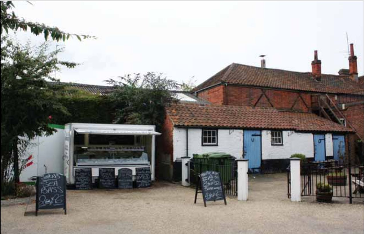
Plate 3: North-facing elevation of outbuildings at rear of the White Hart with first floor of bakehouse behind
