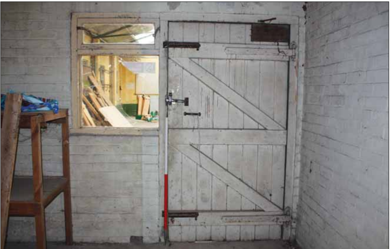
Plate 16: Detail of door as viewed from inside of "office"/G4
