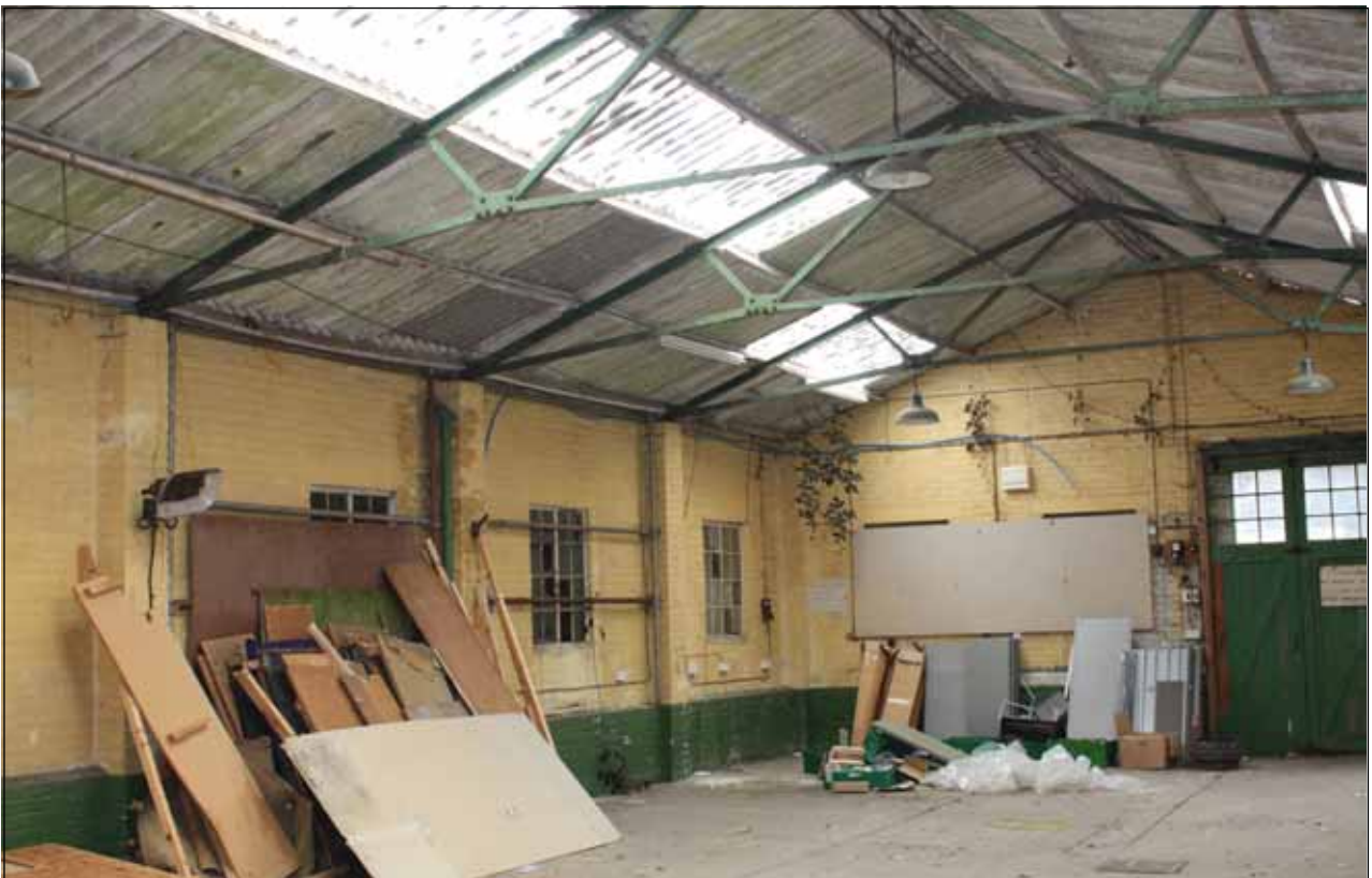
Plate 8: Internal view of windows on the north elevation of auction house
