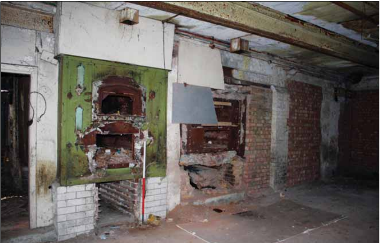
Plate 22: Ovens in ground floor room of bakehouse
