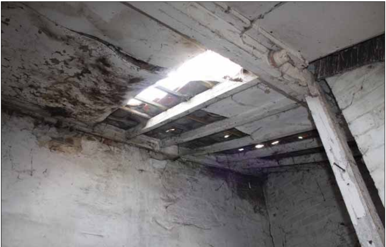
Plate 35: Detail of roof structure, Building 5
