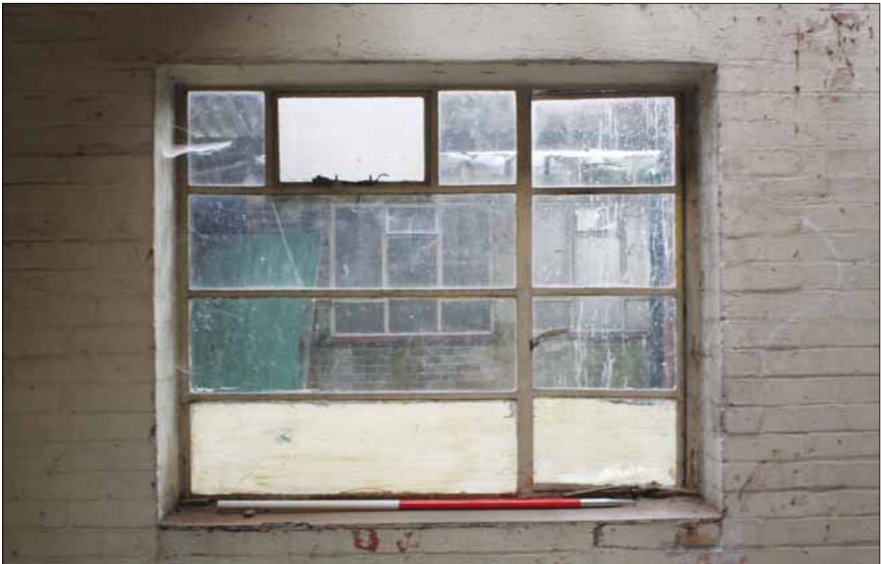
Plate 17: Detail of window on southern elevation of “office”/G4
