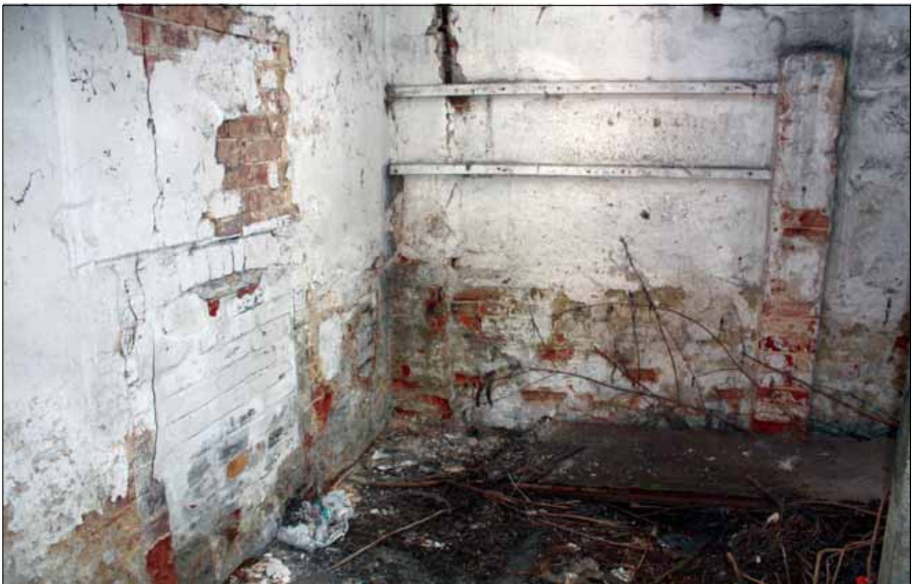
Plate 34: Interior of Building 5 showing blocked-up fireplace and wall support buttress
