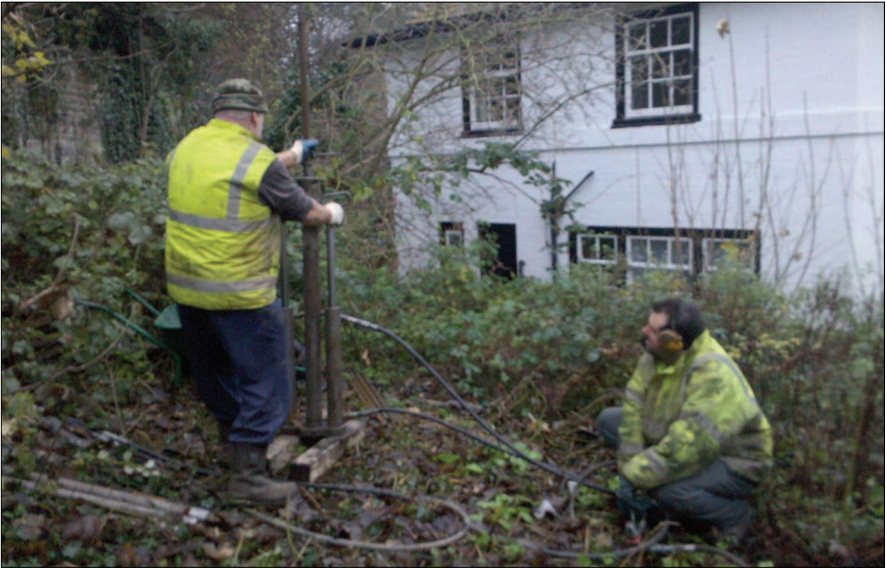
Plate 5: Bore hole sampling
