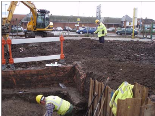
Plate 6: Working shot showing trench with location of Lidl site (MNF31393) in background
