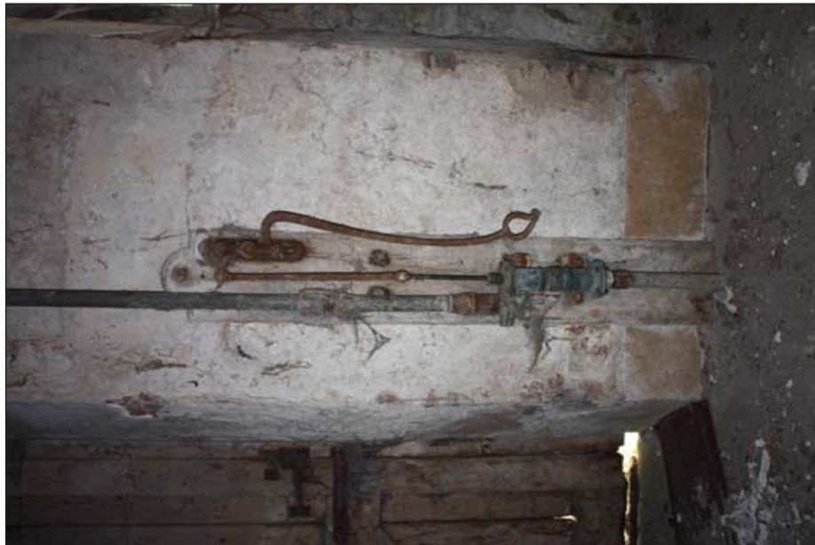
Plate 19: Water Pump, G1
