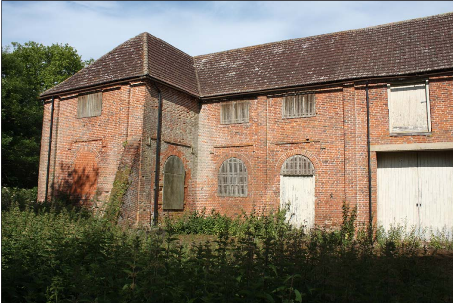
Plate 5: South-East facing elevation
