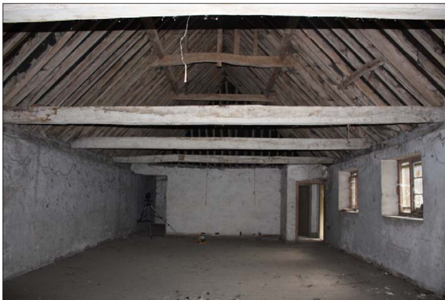
Plate 34: View of F1 showing exposed roof detail
