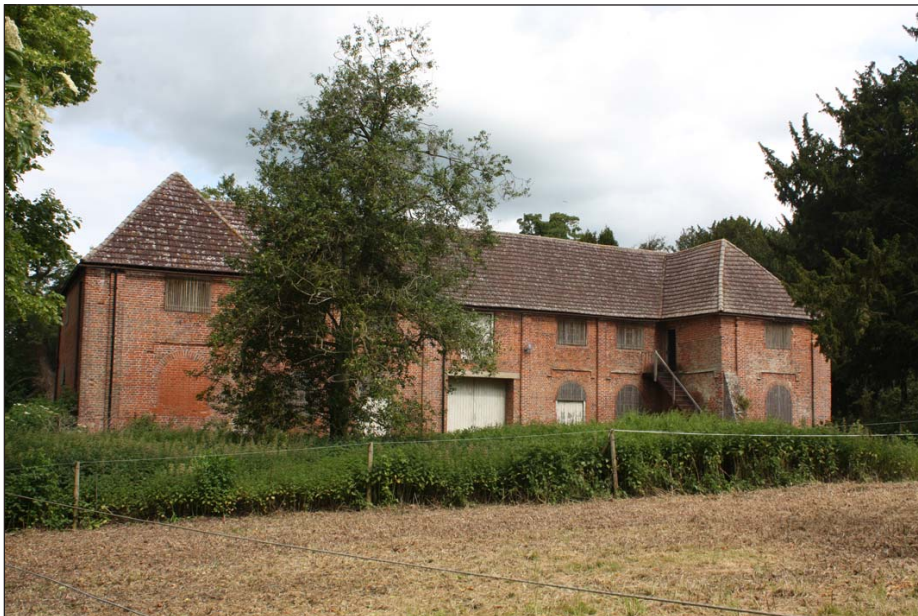
Plate 4: South-East facing elevation
