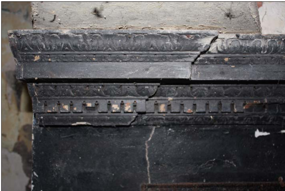
Plate 54: Detail of fire surround, F8
