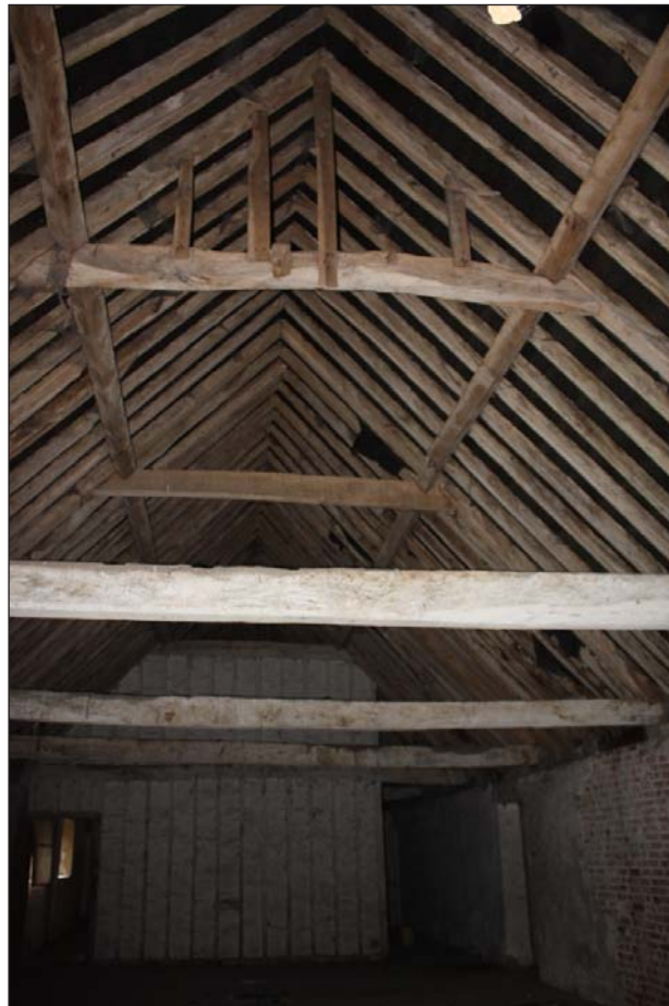
Plate 33: View of F1 showing exposed roof detail
