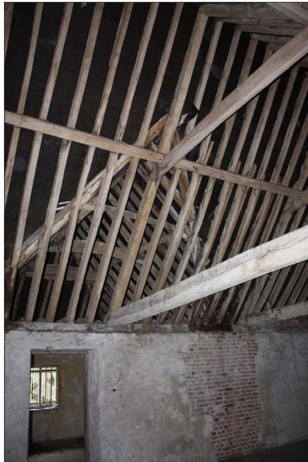
Plate 37: Detail of roof covering over F1 and F10
