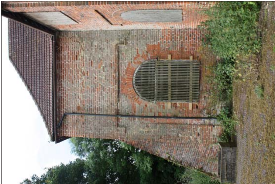
Plate 7: Detail of "wing" on South-East facing elevation
