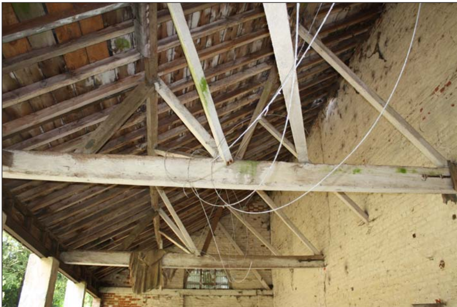
Plate 24: Detail of roof supports, G2
