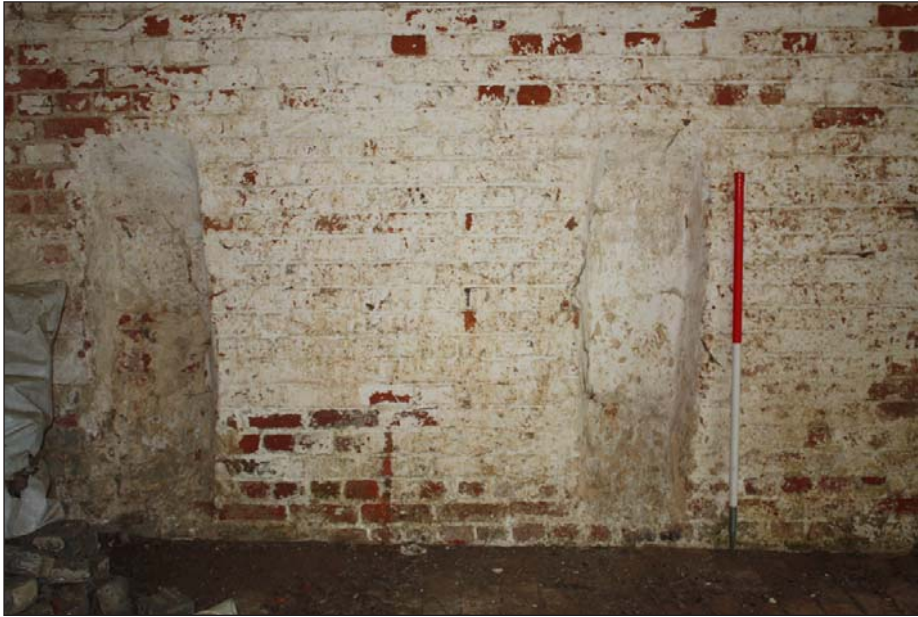
Plate 21: Detail of brickwork, G2, showing Cart Wheel “supports”
