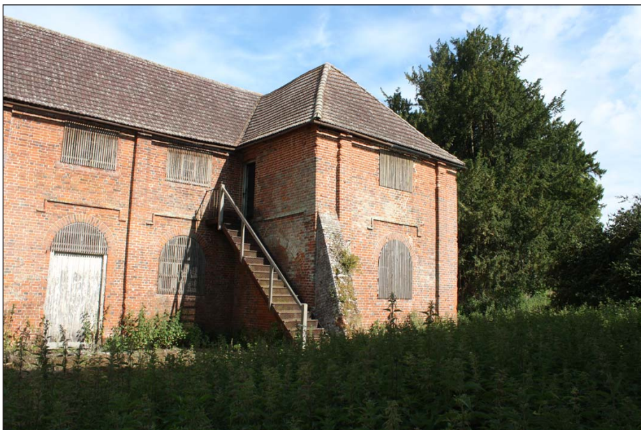
Plate 6: South-East facing elevation
