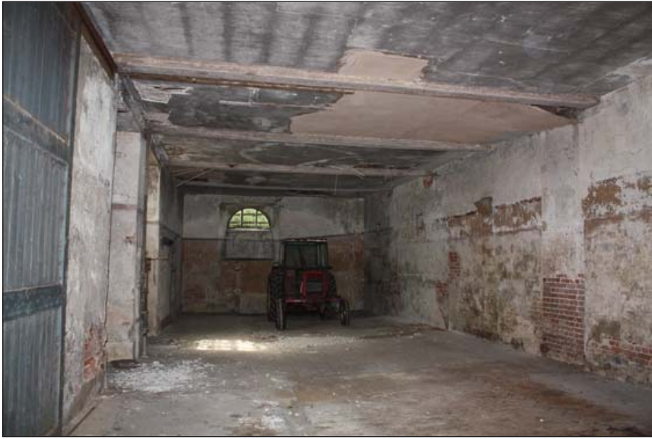
Plate 15: Internal view of G1
