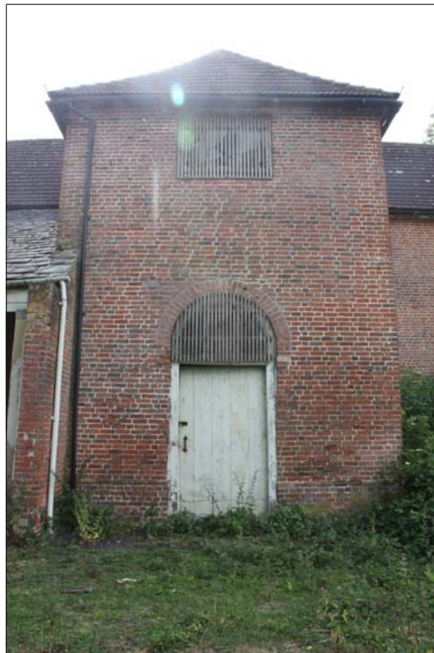
Plate 2: North-West facing elevation
