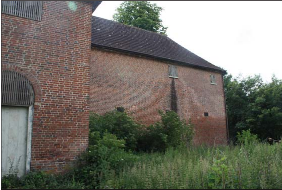
Plate 3: North-West facing elevation
