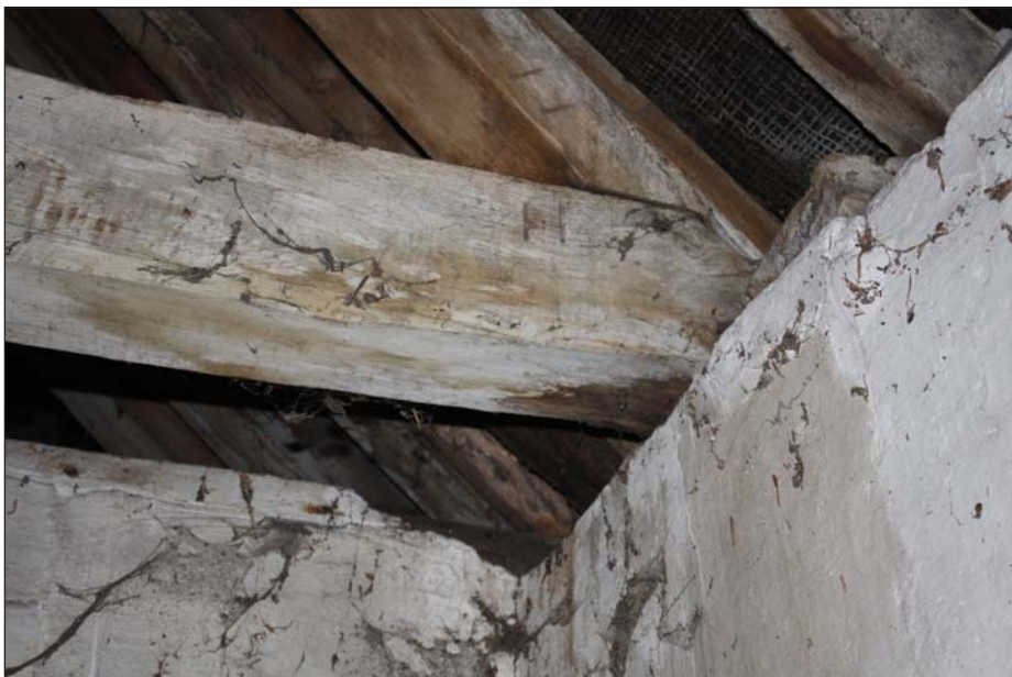
Plate 36: Detail of carpenters marks, F1
