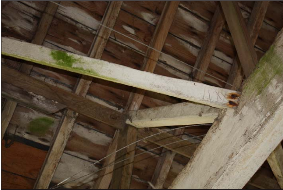
Plate 25: Carpenters Marks, G2
