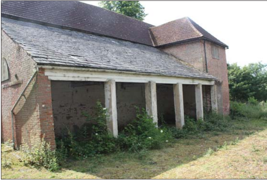
Plate 1: North-West facing elevation
