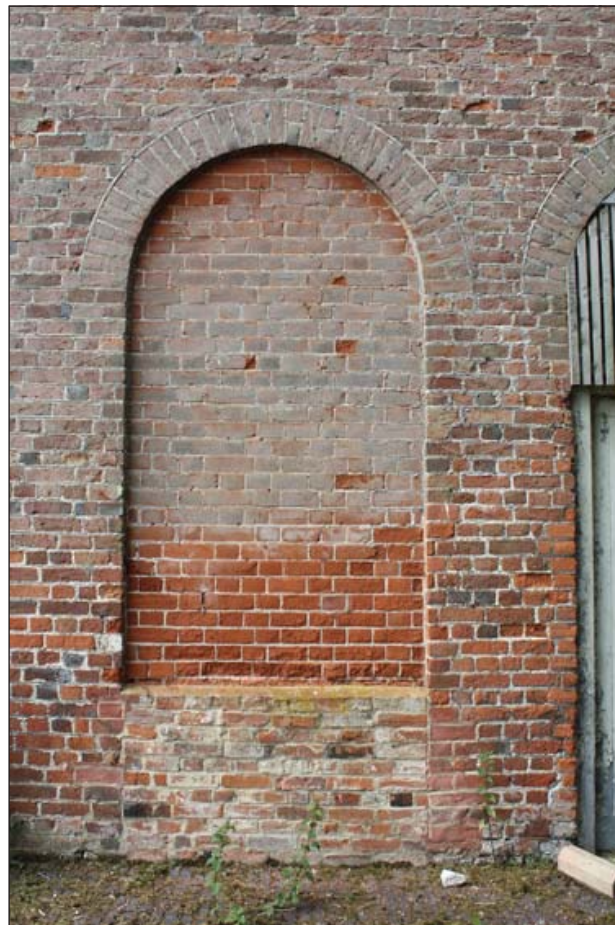
Plate 12: Detail of blocked-up doorway on North-East facing elevation
