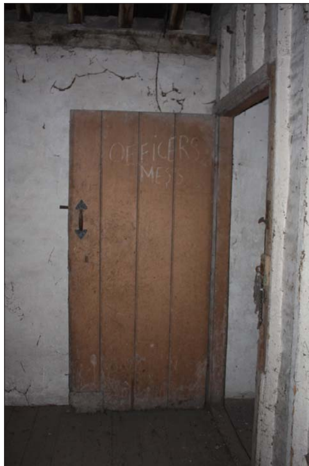
Plate 40: Internal door between F1 and F5
