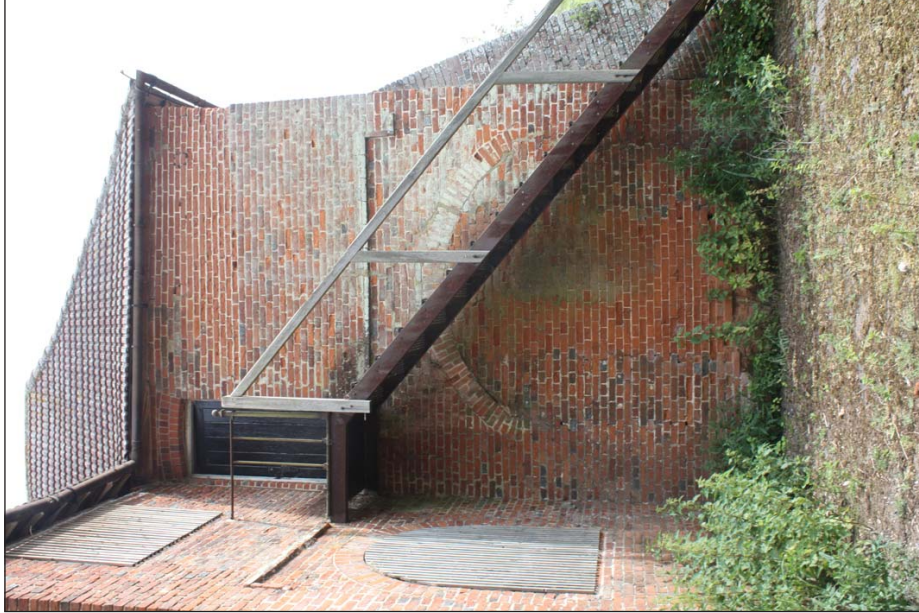
Plate 8: Detail of blocked-up archway and external staircase on south-east facing elevation
