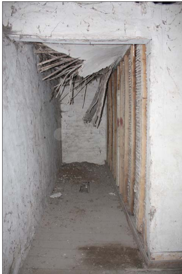
Plate 42: Area rear of F3, showing continuation of hatches
