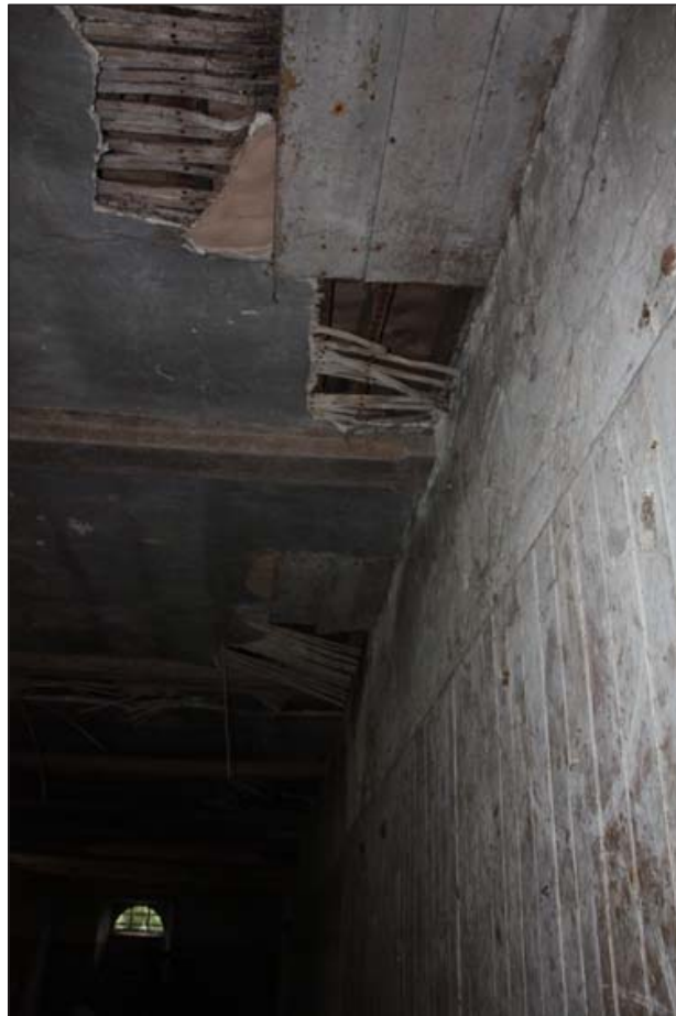
Plate 16: Detail of "hatches" in ceiling of G1
