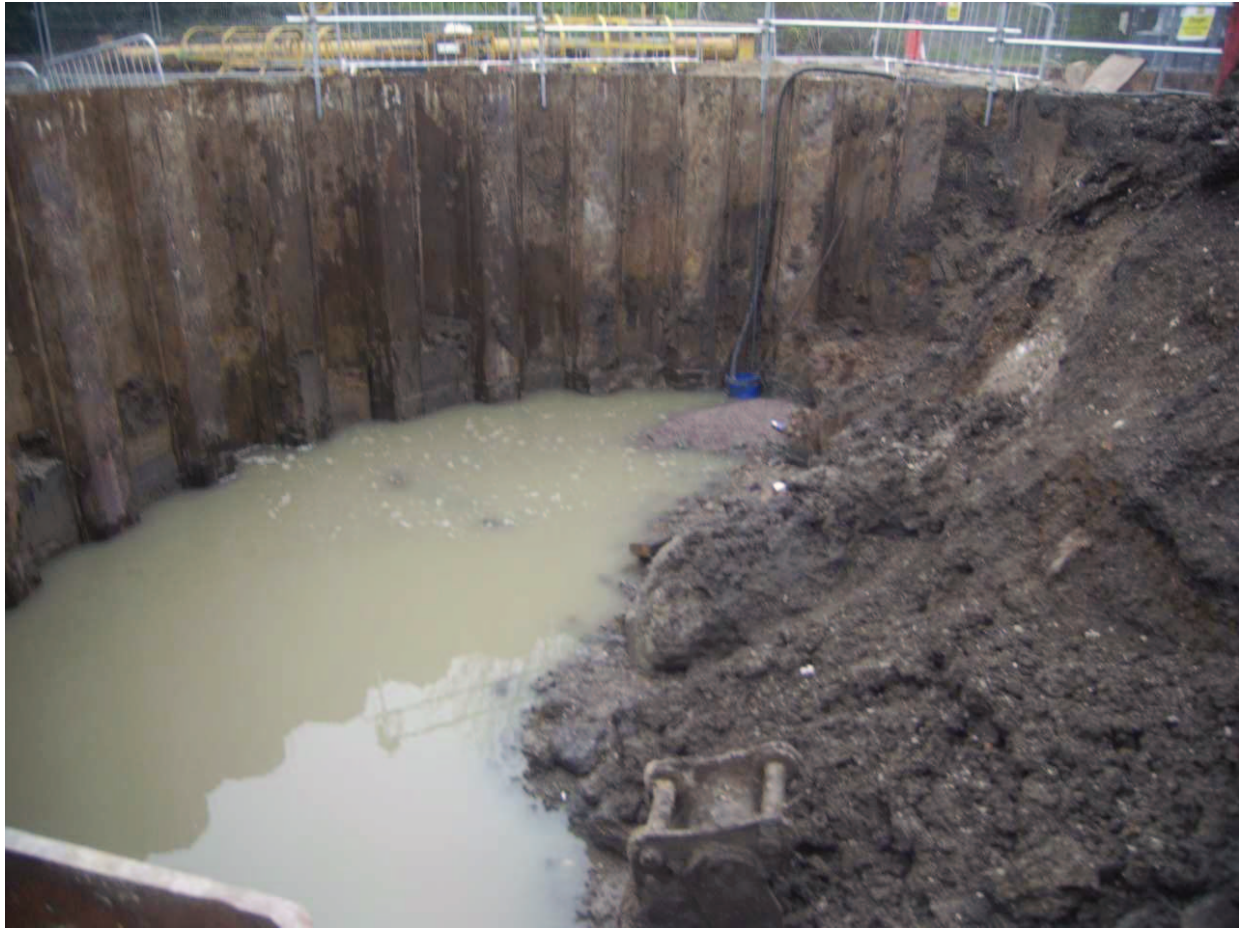
Plate 5: Site conditions within Area A
