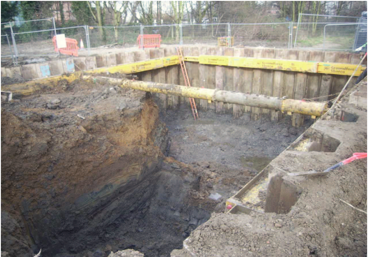
Plate 3: Excavation and section through Areas B
