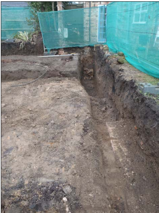
Plate 2: Showing foundation extraction from the west
