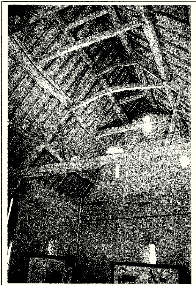
Plate 3: barn roof looking north
