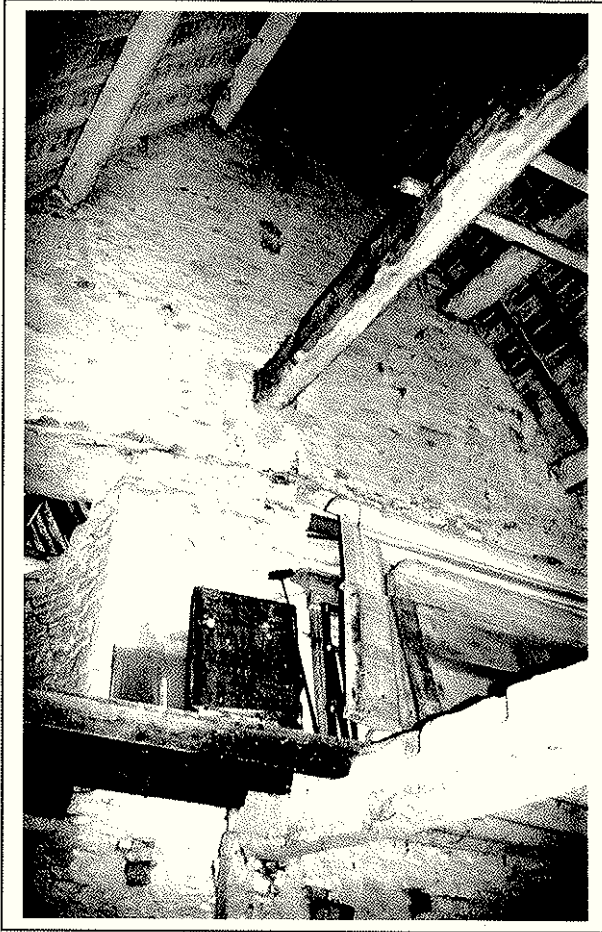
Plate 9: View of upper part of Area 2 looking north showing primary principal joist and later landing
