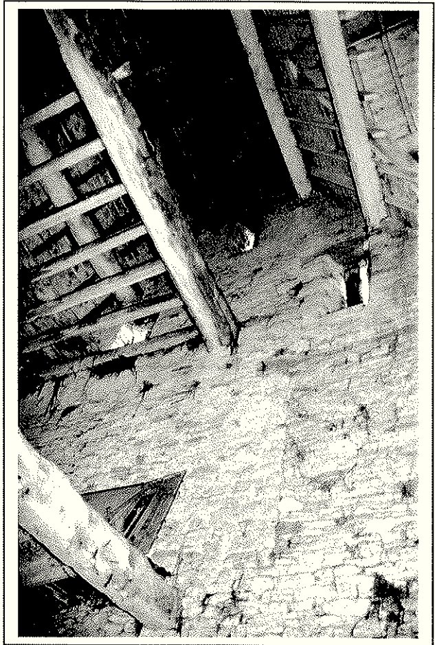
Plate 10: South gable of Area 2 showing partially surviving second floor
