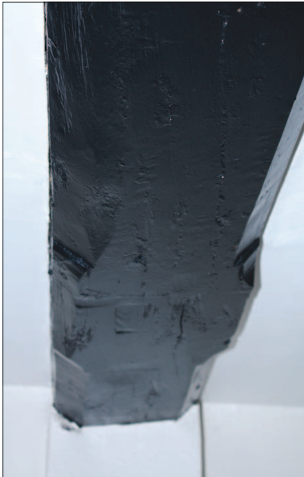
Plate 41: Detail of stops on chamfered beam, F2
