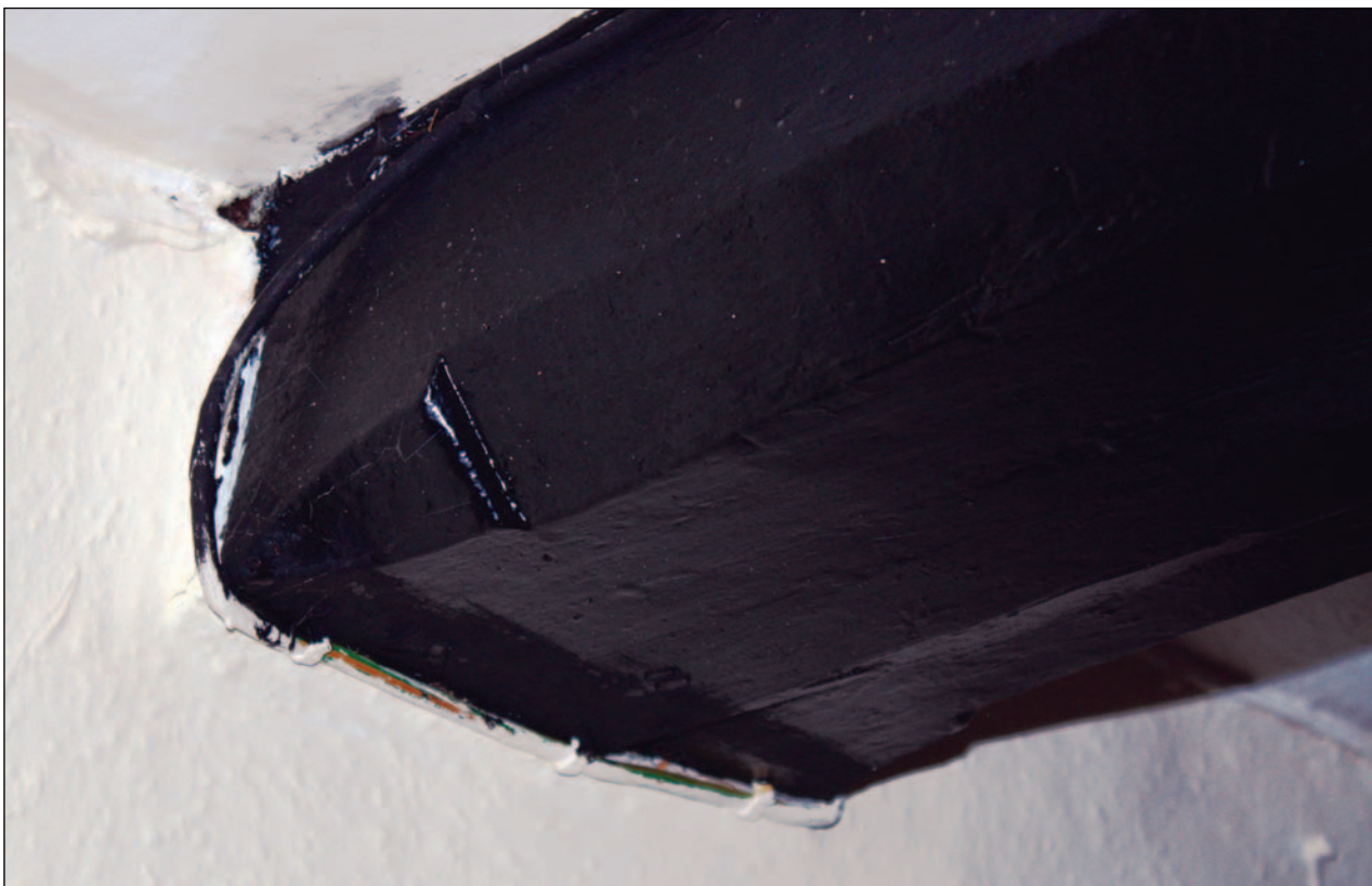
Plate 14: Detail of stop-chamfered beam, G1
