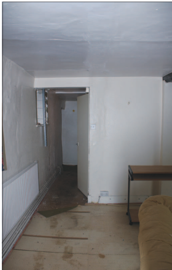
Plate 43: Ghost-lines of removed internal partition, F2
