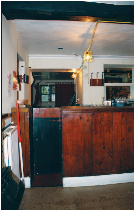
Plate 18: Bar, stop-chamfered beam, G2
