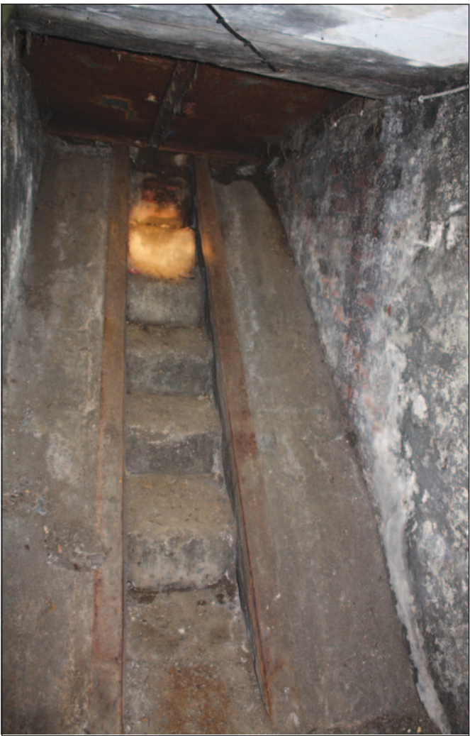
Plate 56: Barrel chute in cellar
