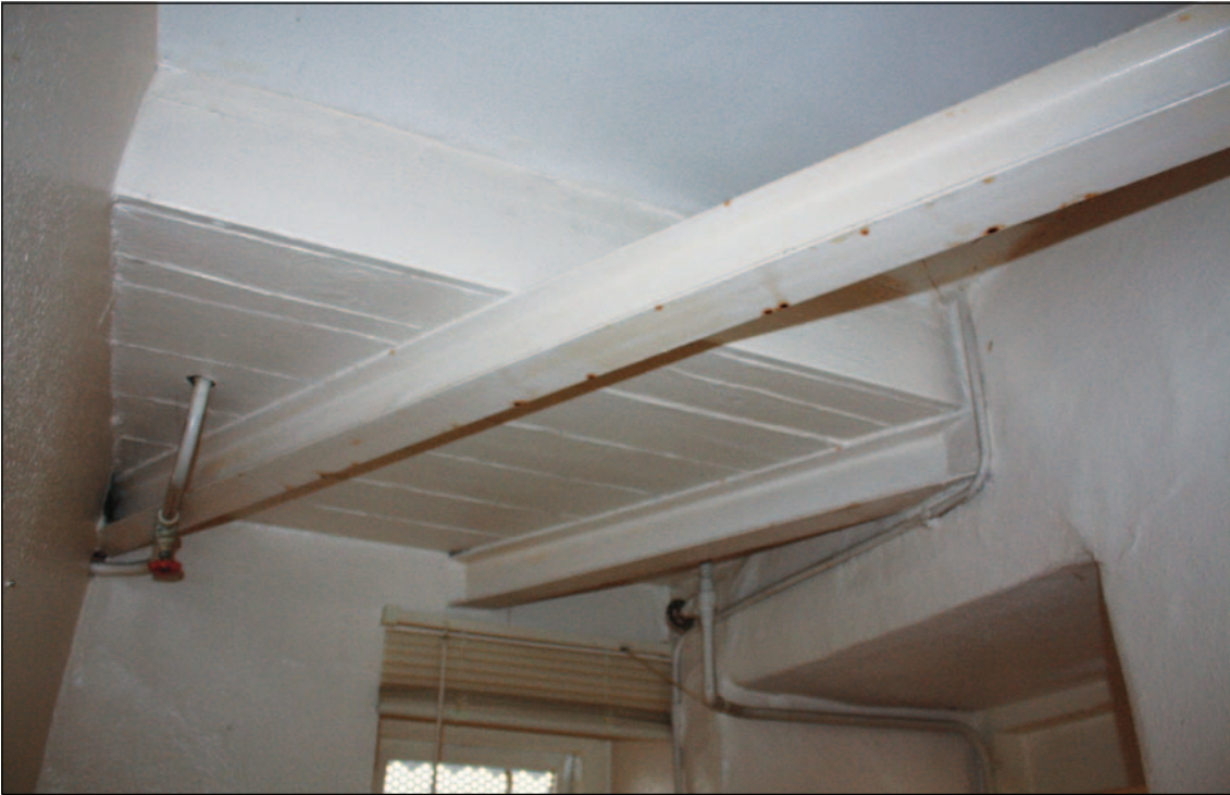
Plate 44: Reinforced steel joists, F3
