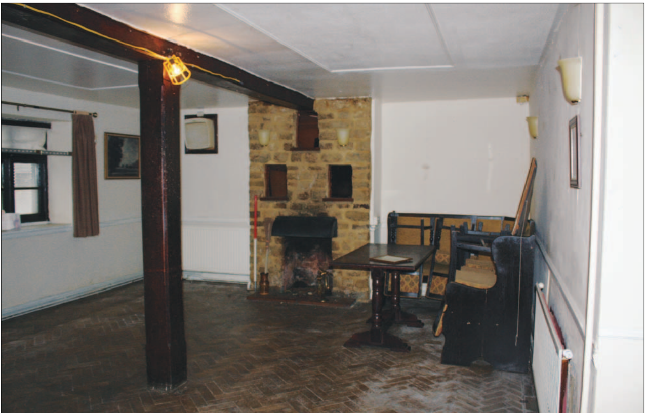
Plate 23: General room view showing fireplace, parquet floor and chamfered beam, G4
