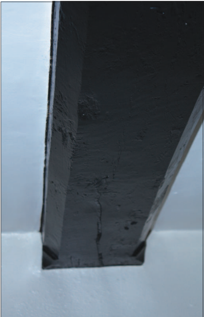
Plate 42: Stop-chamfer, F2
