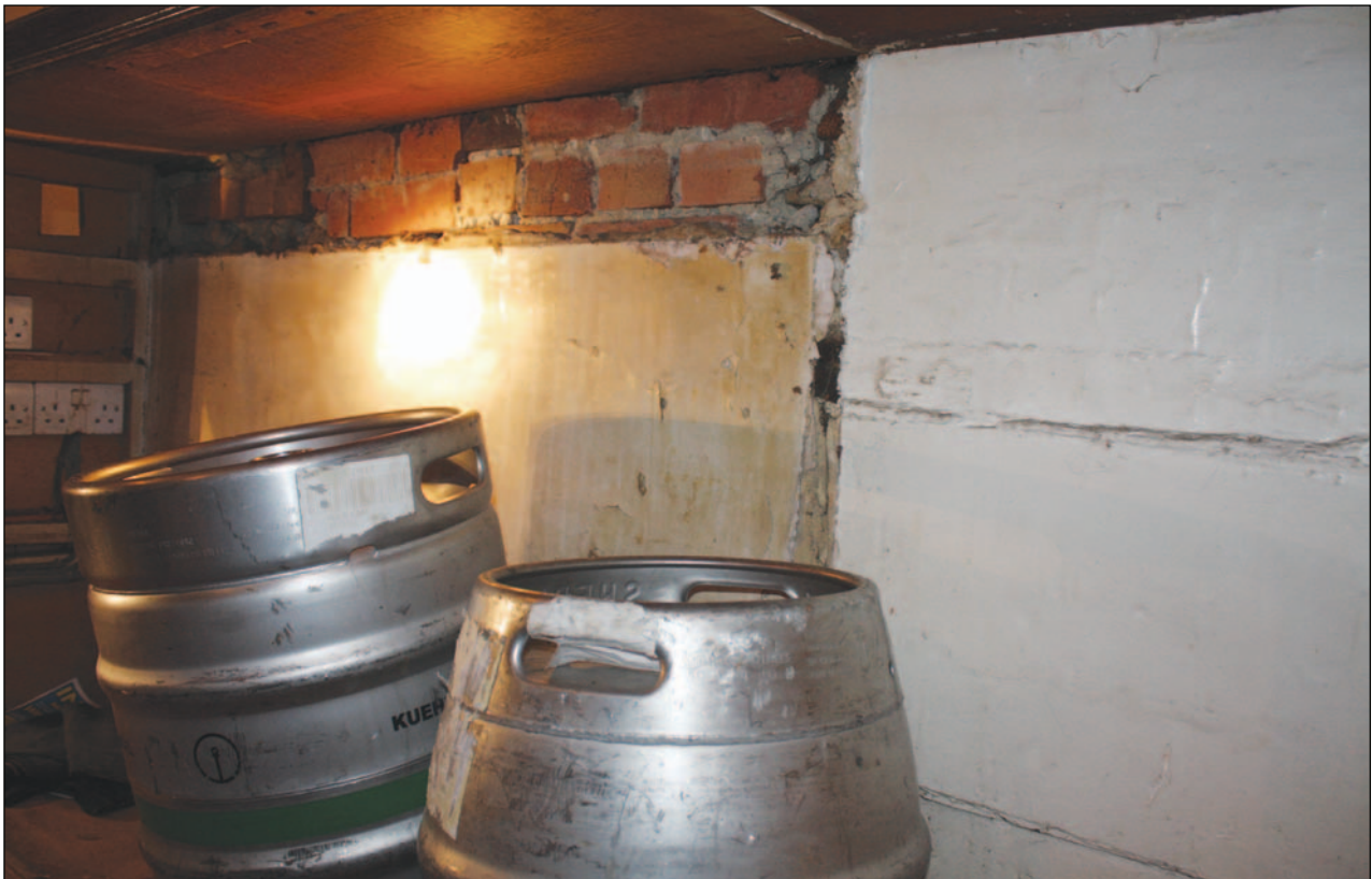
Plate 20: Detail of blocked-up opening behind bar, G2
