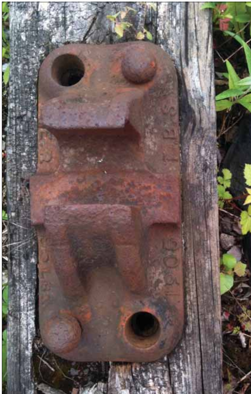
Plate 10: Railway Chair Baseplate (or tie plate)
