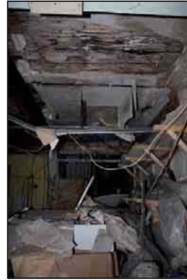
Plate 18: Detail of lath and plaster ceiling and mouldings, G5, 130b
