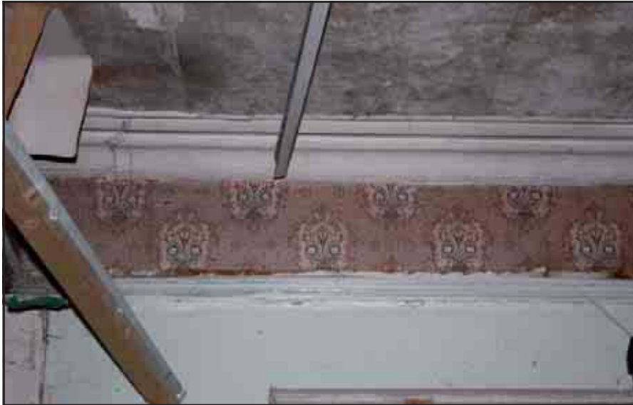
Plate 21: Plaster ceiling cornice, picture rail and decorative wallpaper, G5, 130b
