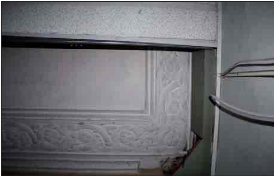
Plate 23: Detail of decorative plaster ceiling cornice, G5, 130b
