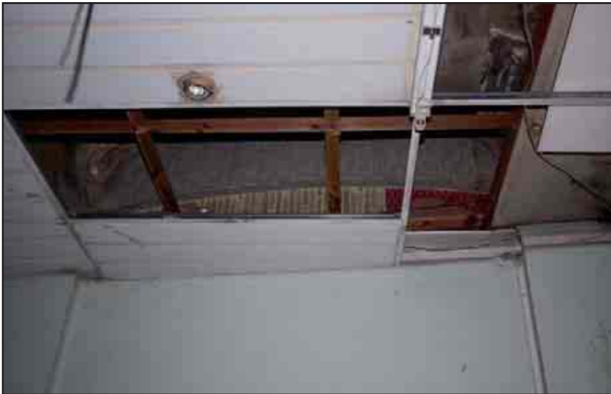
Plate 15: Top of archway, concealed behind C20th shop fittings, G4, 130b
