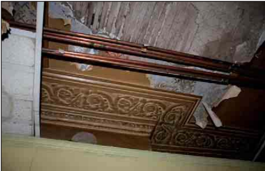
Plate 19: Detail of decorative plaster ceiling cornice around concealed fireplace, G5, 130b
