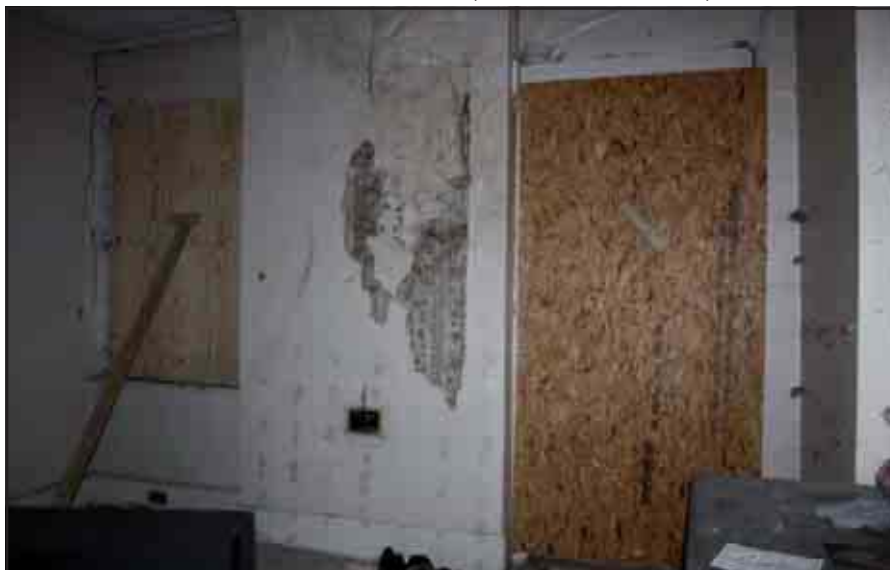
Plate 31: Blocked-up fireplace and boarded-up windows, F2, 130b
