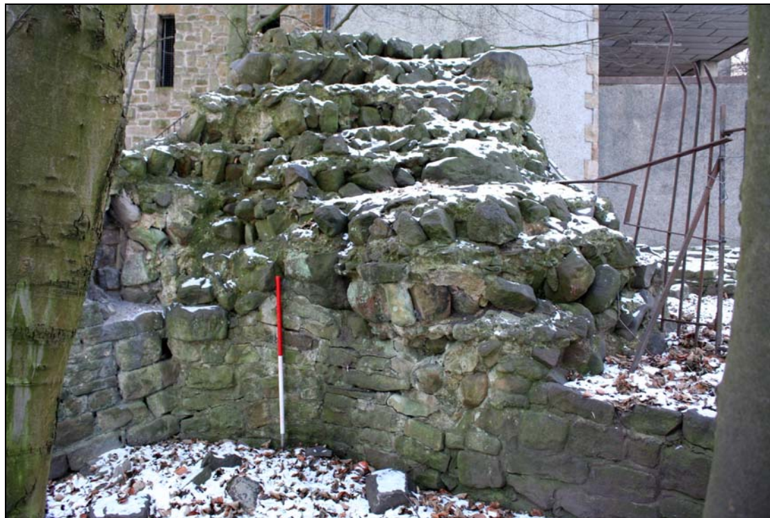
Plate 29: View of the consolidation works undertaken at the foot of the north side of the Wery Wall bastion
