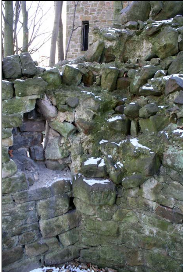
Plate 42: View of the erosion at the interface between the garden wall and Wery Wall fabric on the east side of the bastion
