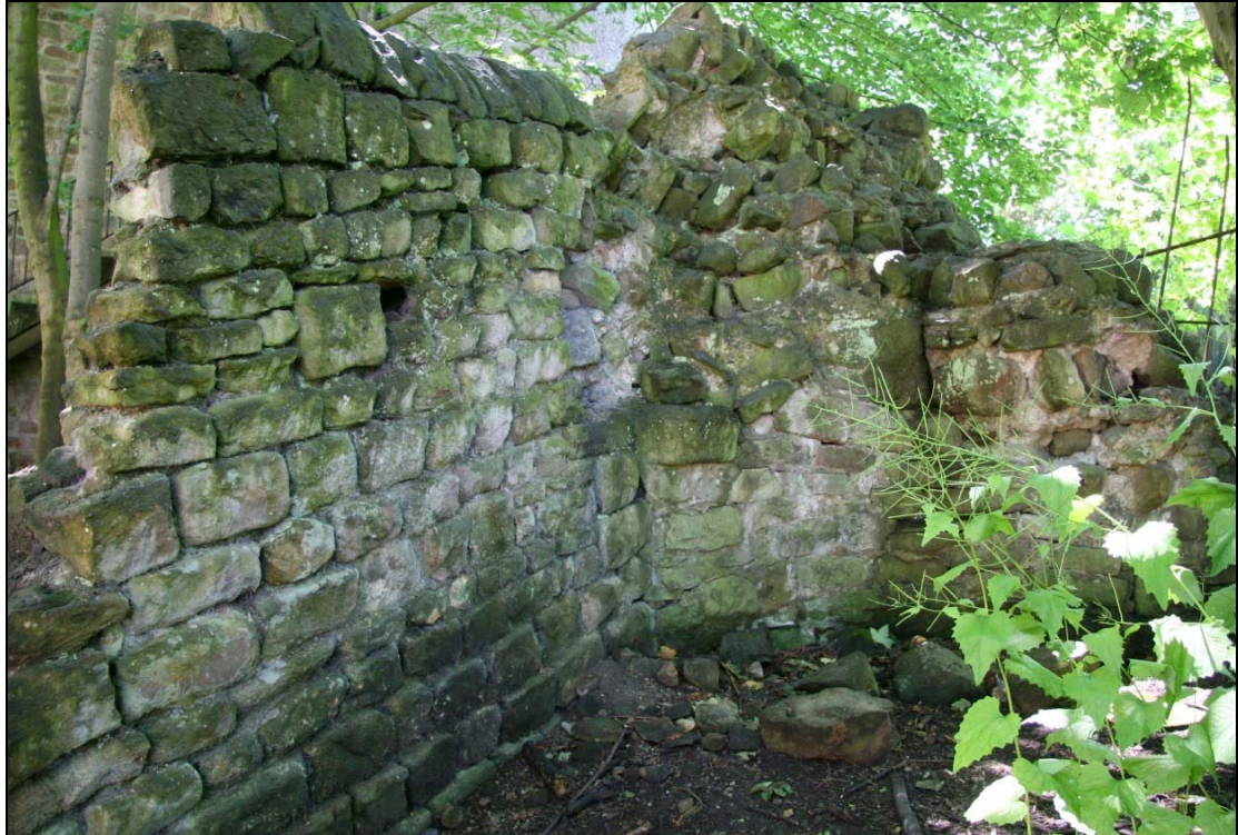
Plate 35: View of the consolidation works undertaken at the foot of the north-east side of the Wery Wall bastion.
