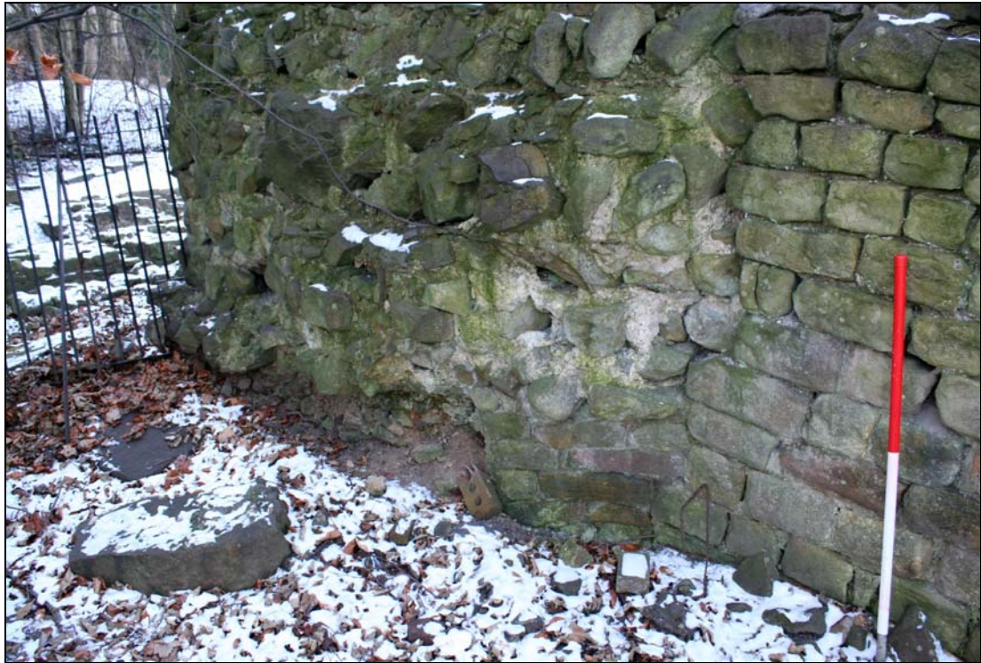
Plate 34: View of the consolidation works undertaken at the foot of the south side of the Wery Wall bastion
