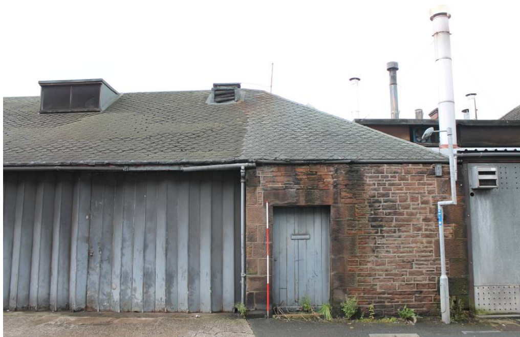
Plate 7: Doorway at the west end of the north elevation of Building 2, also showing quoins on both sides.
