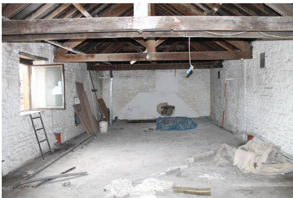
Plate 11: The upper floor of Building 3
