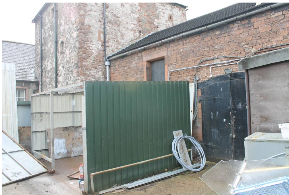
Plate 2: North-facing side of Building 1 showing later additions
