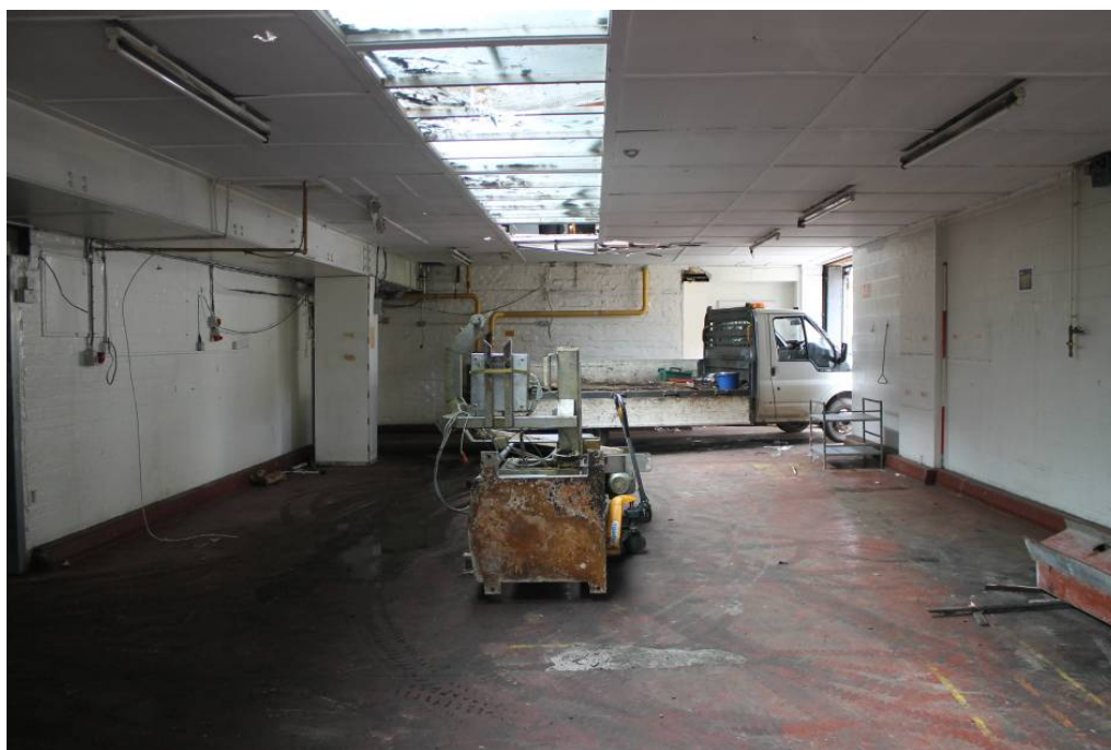
Plate 8: Internal view of Building 2
