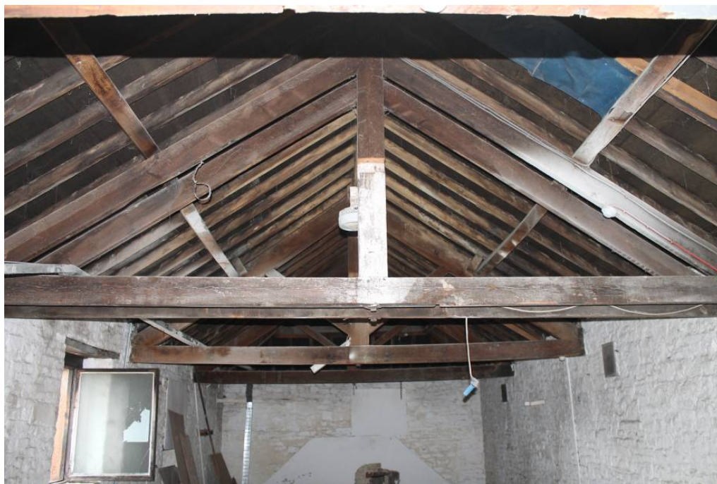
Plate 12: The roof trusses in Building 3
