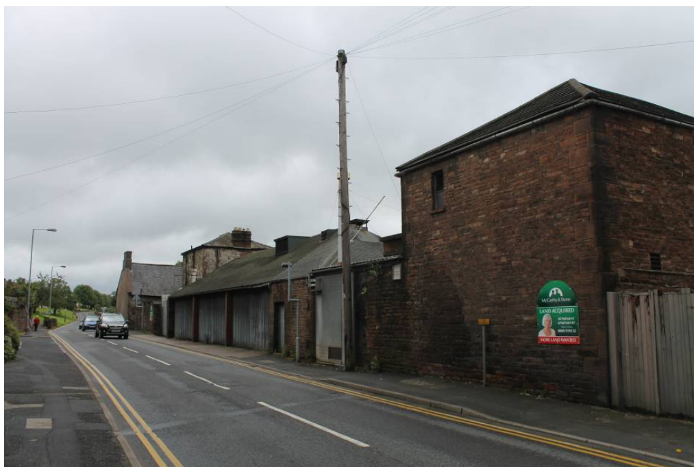
Plate 1: View of the complex from Benson Row, facing south-east, showing Building 3 in the foreground, and Building 2 further along Benson Row
