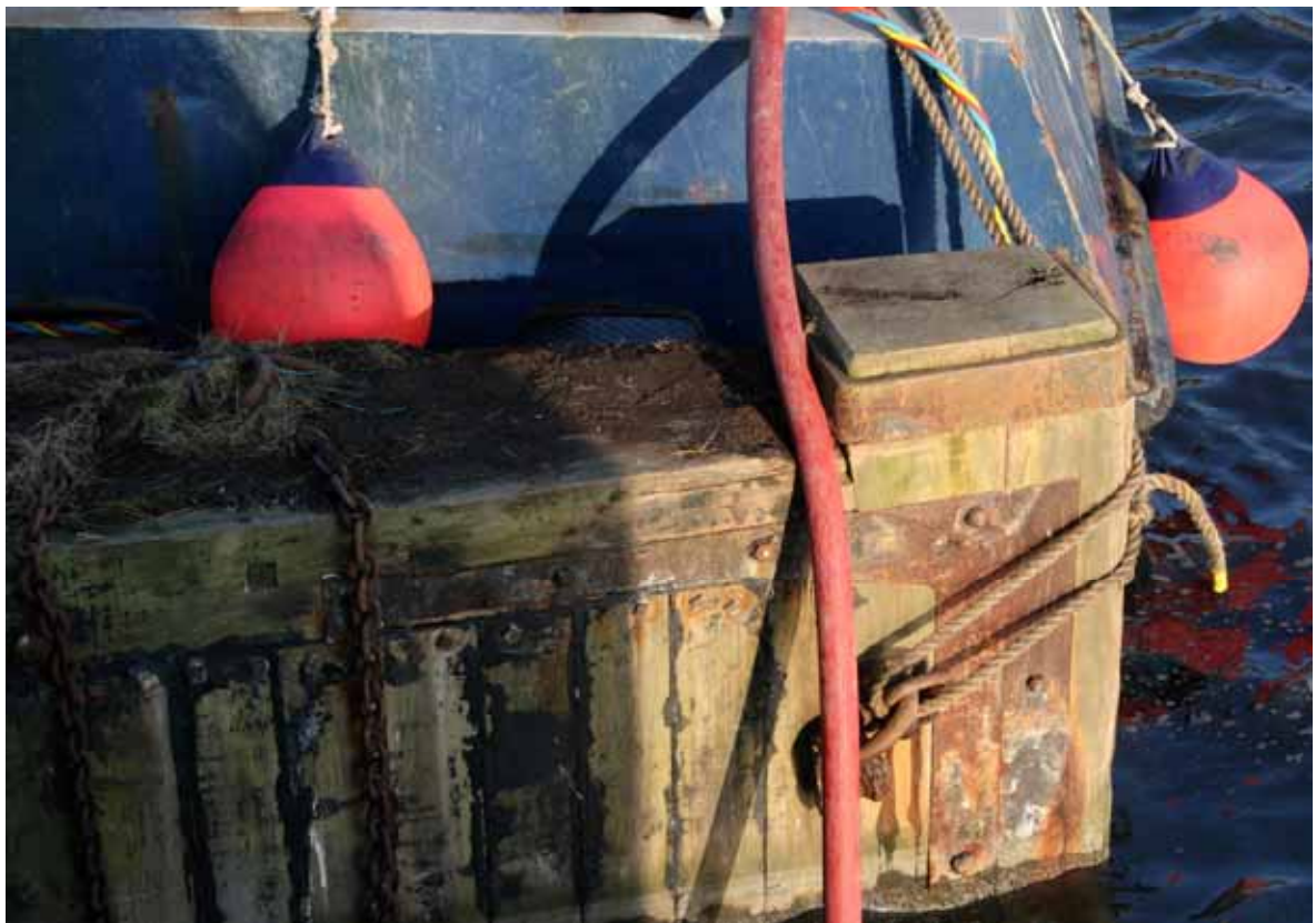
Plate 4: Detail view of metal fixings around the mitre post on the interior elevation of the south dock gate
