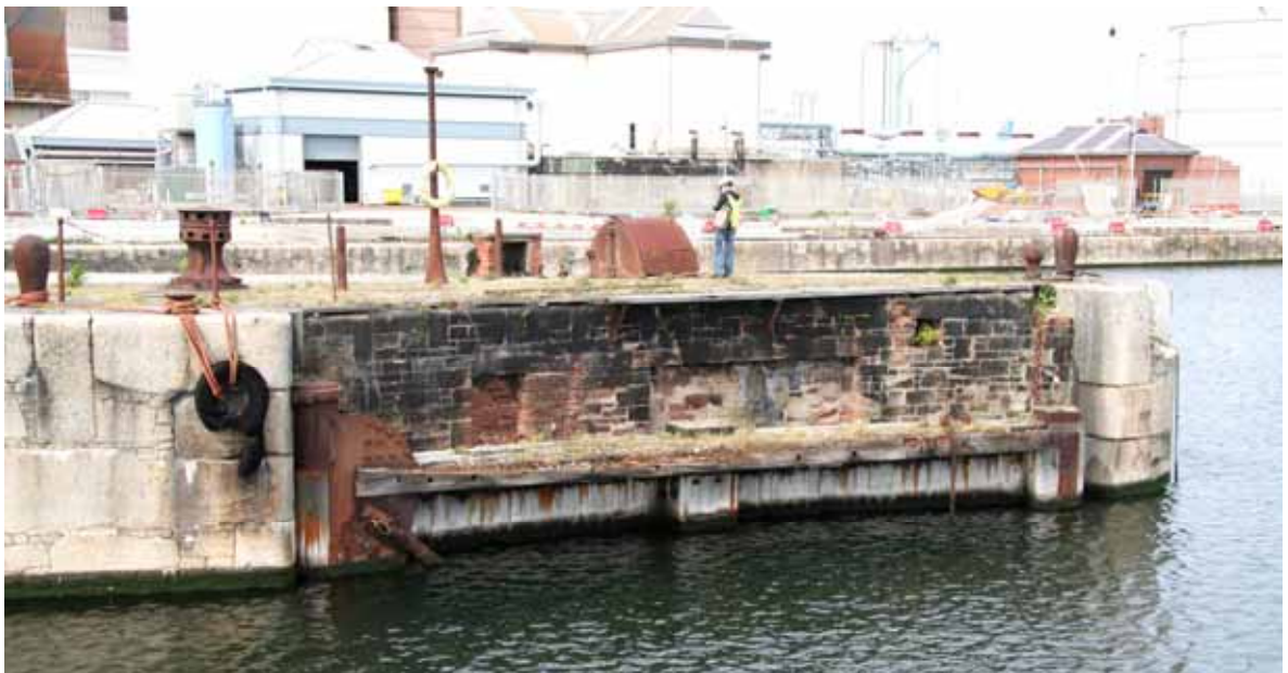
Plate 6: Exterior elevation of dock gates (while still housed in dock gate recess on the north gate pier)
