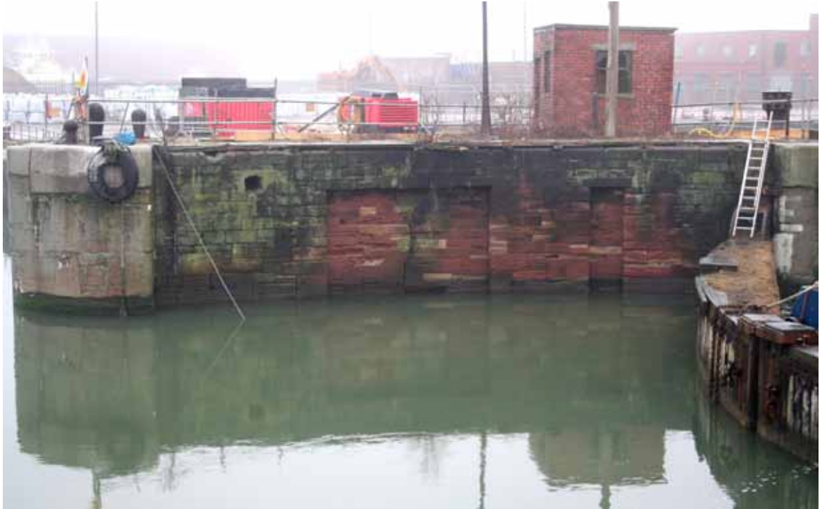
Plate 8: Gate recess in the north-facing elevation of the south gate pier
