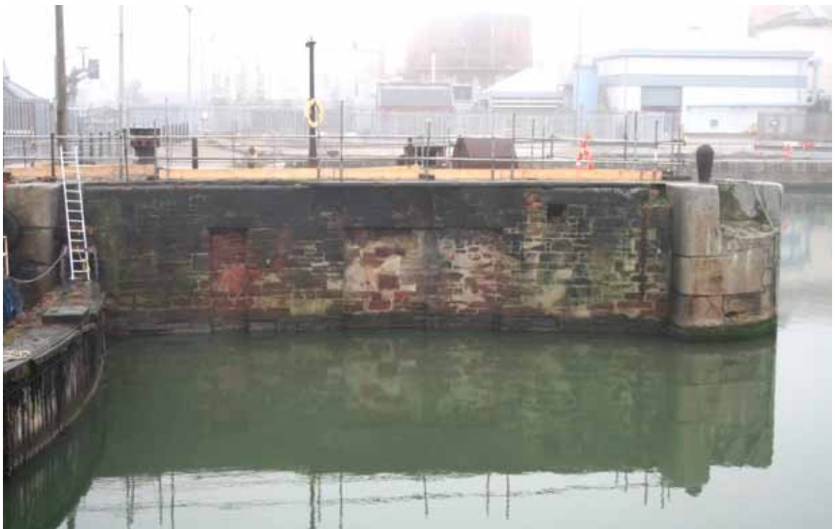
Plate 9: Gate recess in the south-facing elevation of the north gate pier
