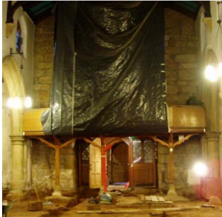
Plate 13: The roof scars visible on the east side of the tower (west end of the nave), either side of the tarpaulin
