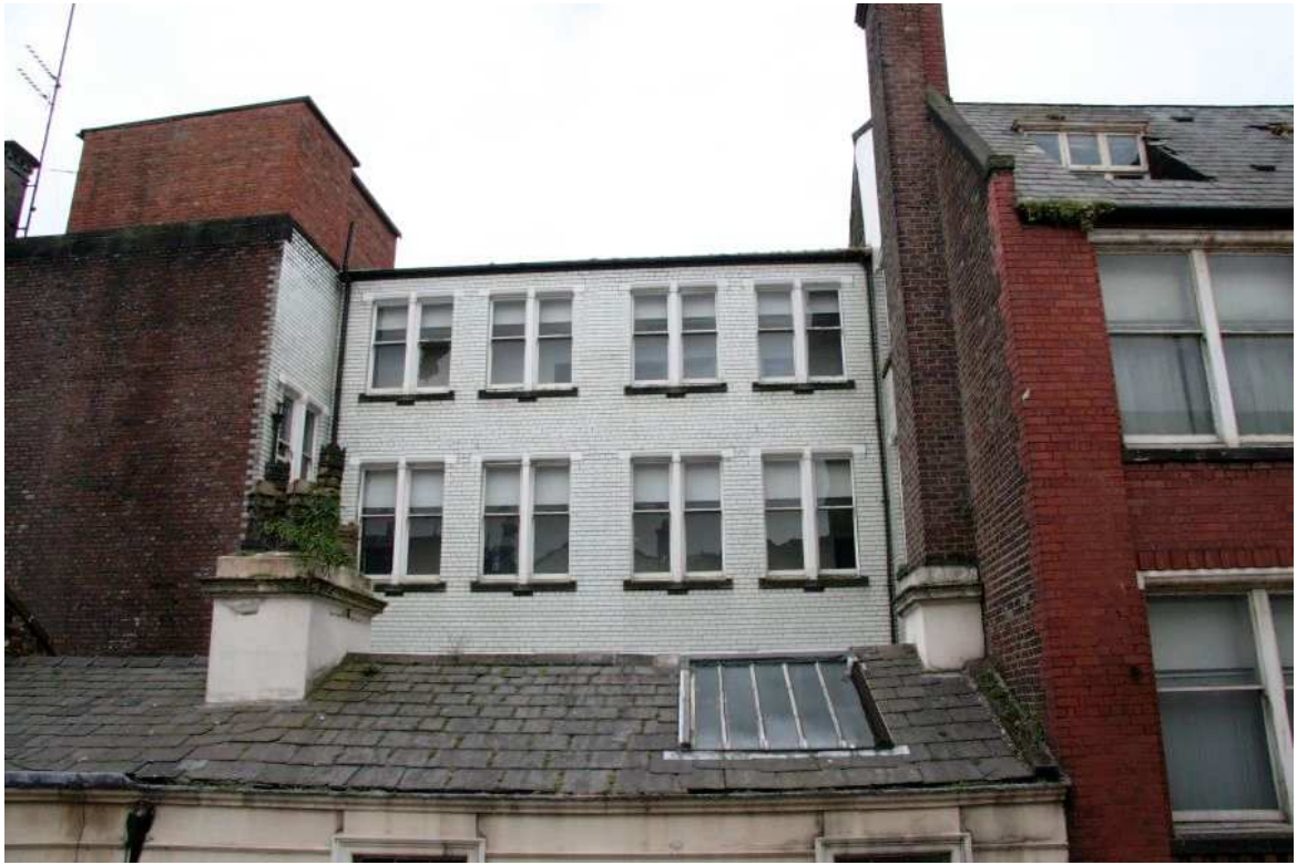
Plate 49: Southern element of the south-facing elevation of 67 Dale Street
