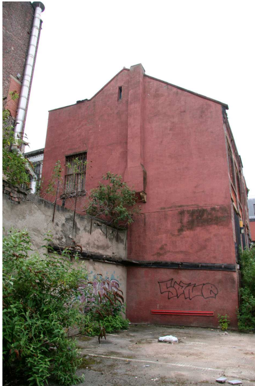
Plate 3: East-facing rendered elevation of Hale Street Warehouse
