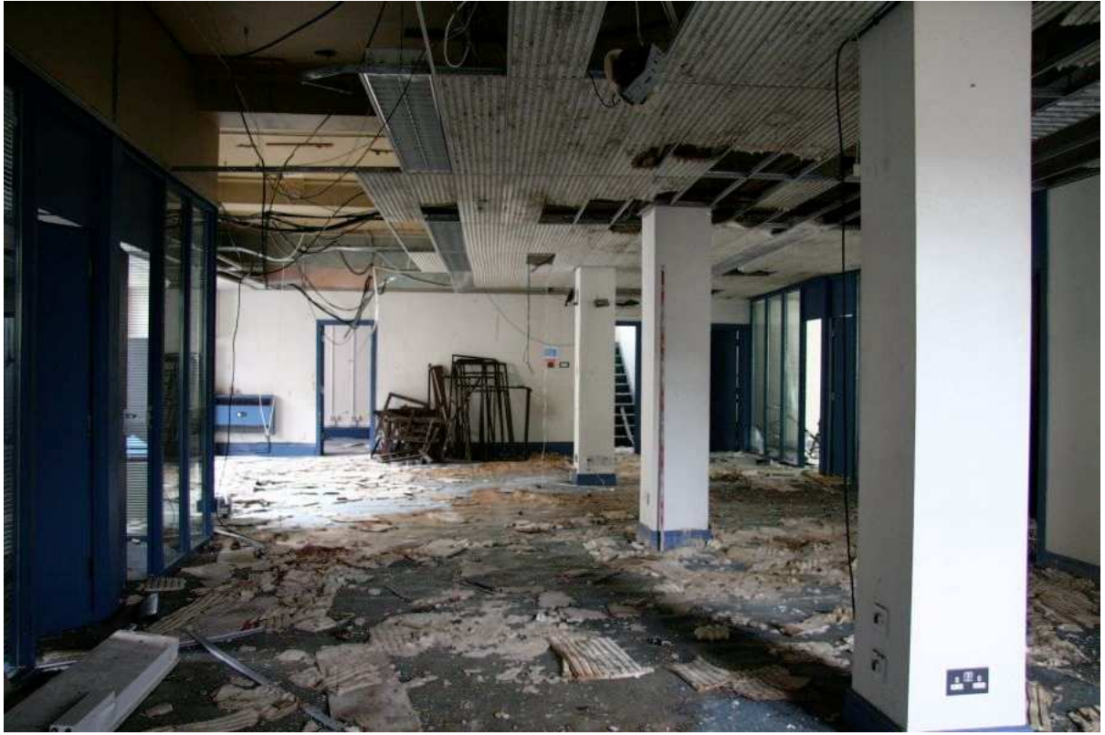
Plate 61: Detail of office arrangement on the third floor
