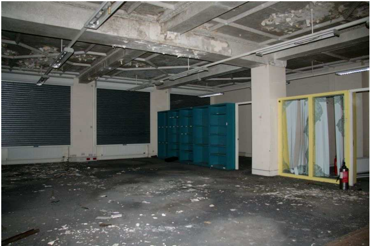
Plate 57: Original plaster moulding detail between the beams in Room 47
