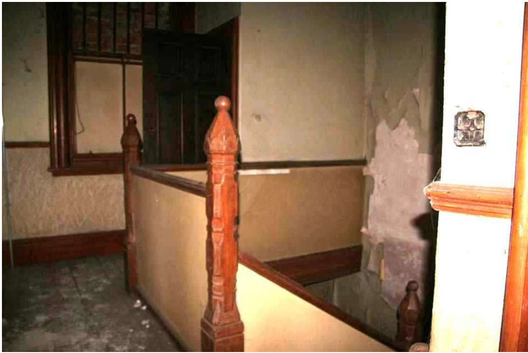
Plate 9: Stairwell 4 and first floor corridor 6 showing newel posts
