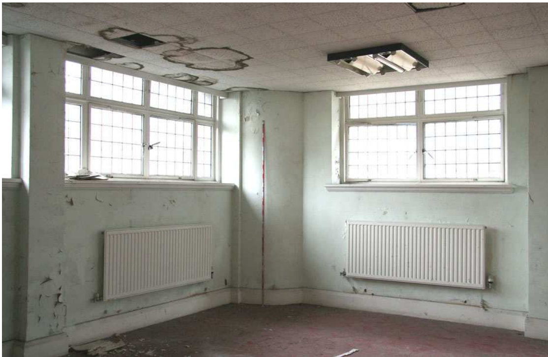
Plate 30: Detail of column in south-west corner of office 18A
