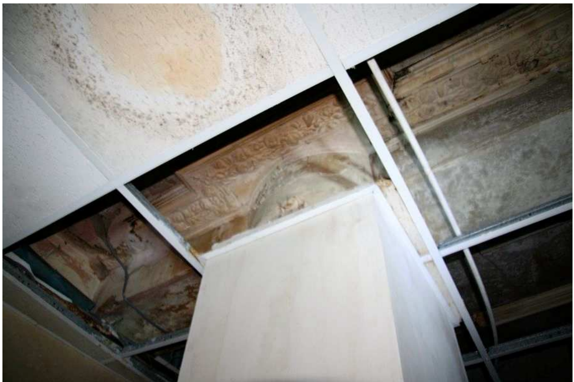
Plate 54: Detail showing the top of the original column and moulded plaster detail
