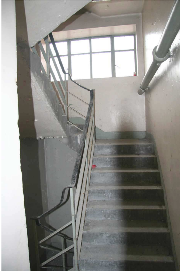
Plate 17: Stairwell 12 at rear of 57 Dale Street
