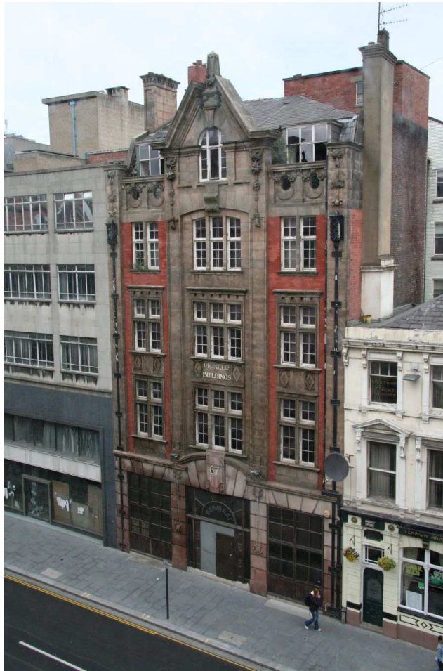
Plate 47: Principal elevation of 67 Dale Street (the Pioneer Building)
