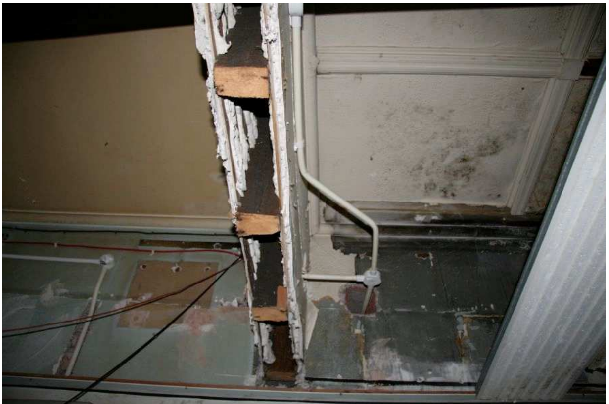
Plate 62: Ornamental plaster moulding, ceiling detail
