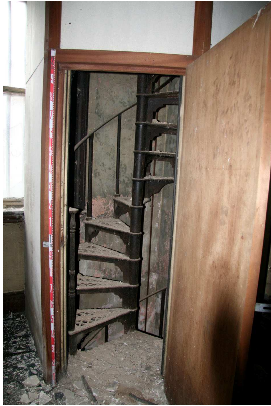
Plate 11: Access to spiral staircase from first floor room 10
