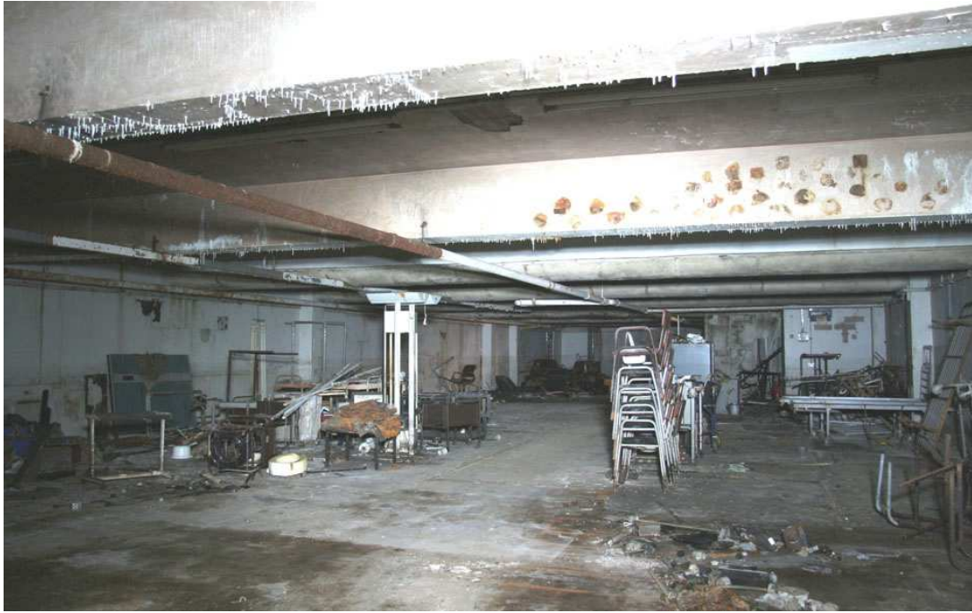
Plate 35: Basement of 61 Dale Street
