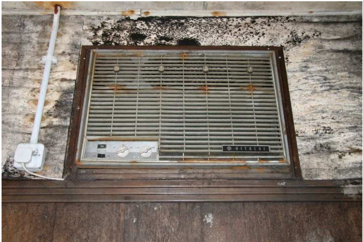
Plate 39: Original air-conditioning system on the first floor
