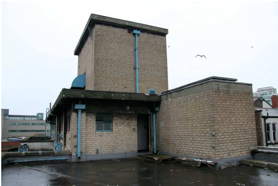
Plate 32: Roof of Eagle Star Building (57 Dale Street)
