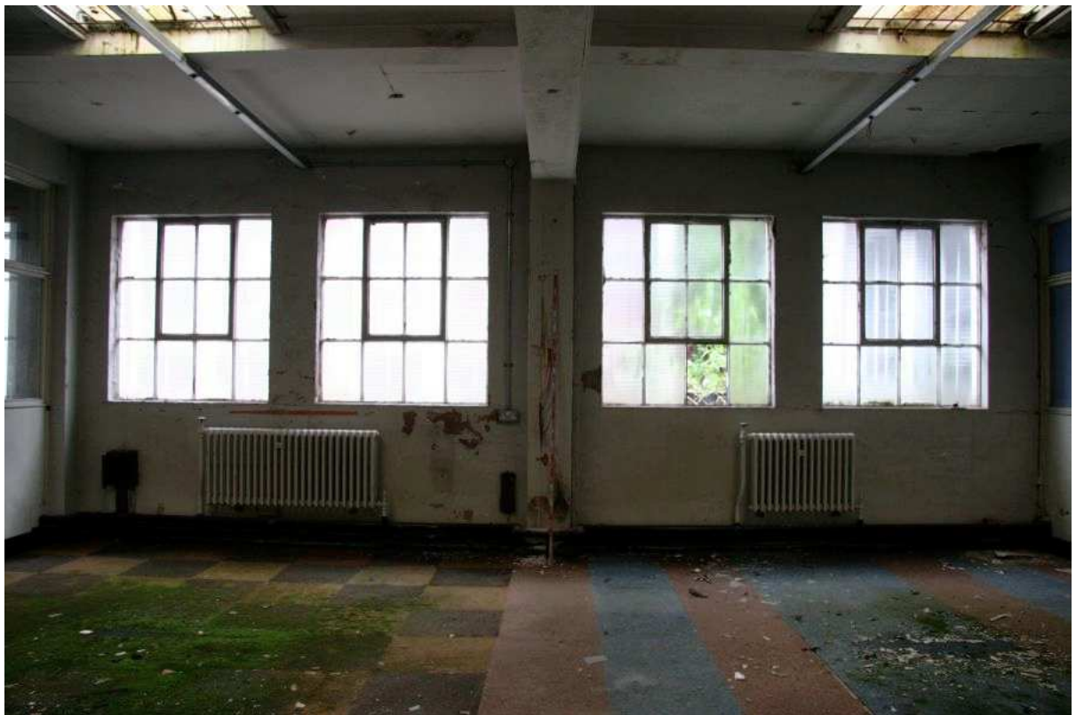
Plate 43: Third floor windows in the east-facing elevation of 61/63 Dale Street
