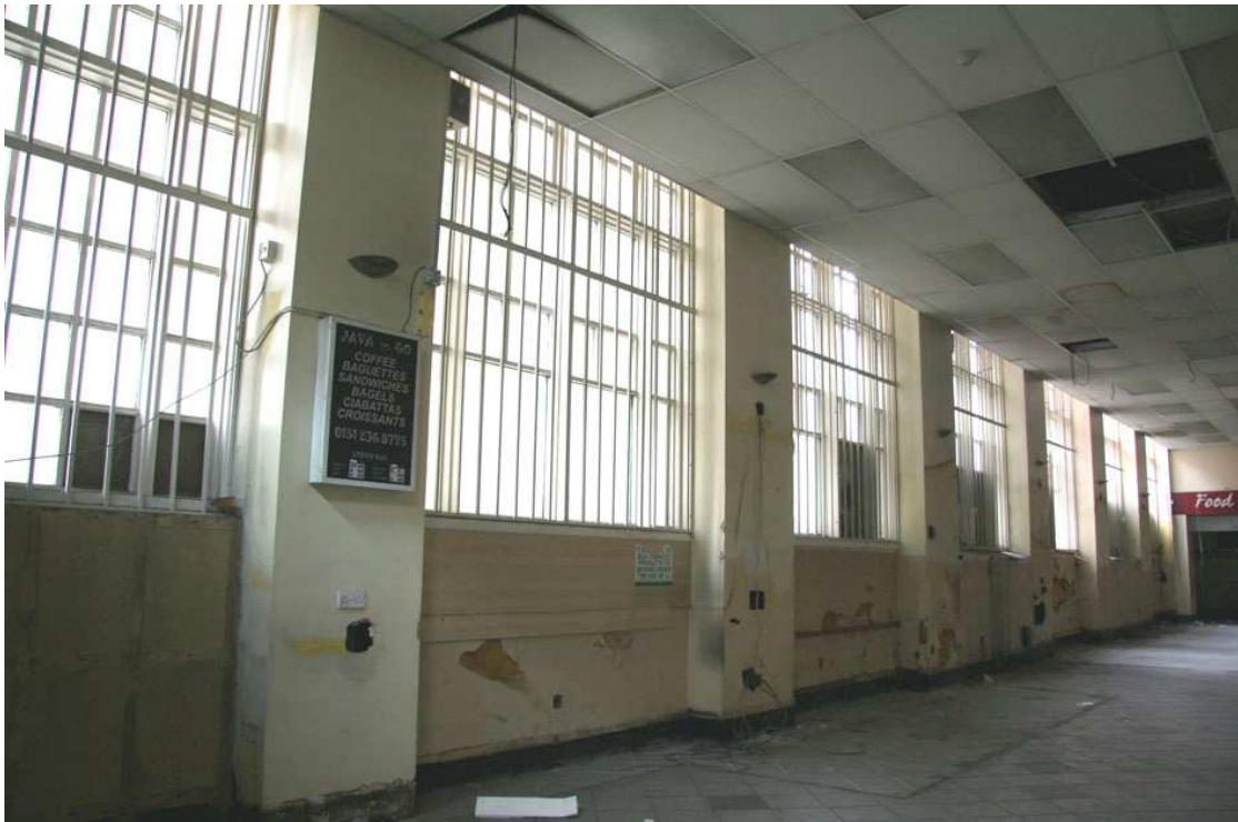
Plate 16: Crittall-style steel-framed windows on west-facing elevation of Spar retail outlet
