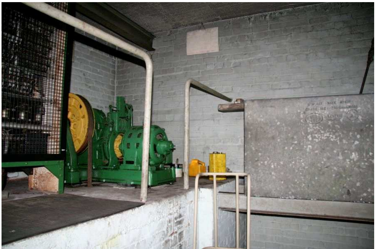
Plate 46: Fifth floor lifting gear
