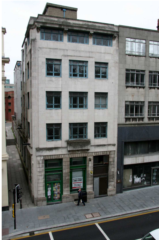
Plate 13: South-facing elevation of 57 Dale Street
