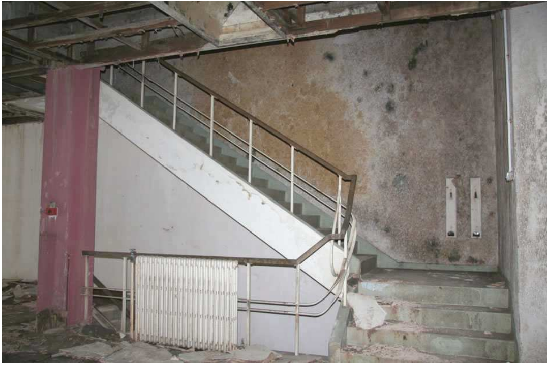
Plate 37: Principal stairwell 26 (west side of building) 61 Dale Street
