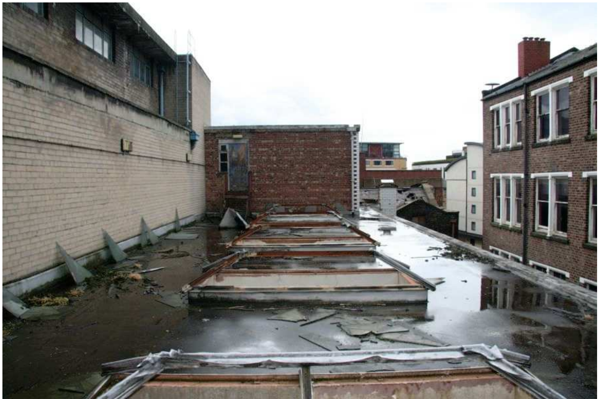
Plate 45: View across the roof to the access door, fourth floor
