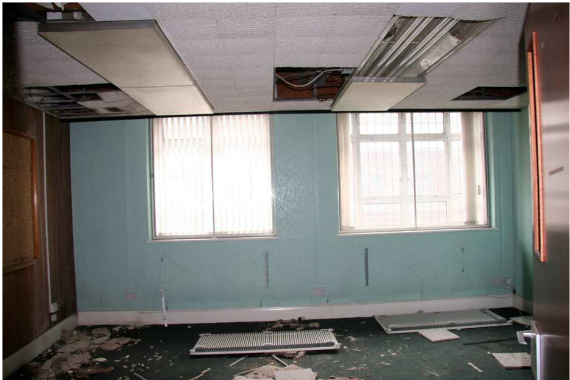
Plate 23: Second floor office space 16E showing panelled walls and suspended ceiling
