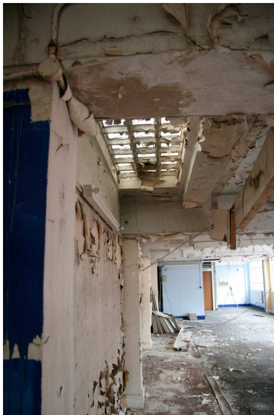
Plate 28: Fourth floor glass brick skylight detail in ceiling of office 18 along eastern wall
