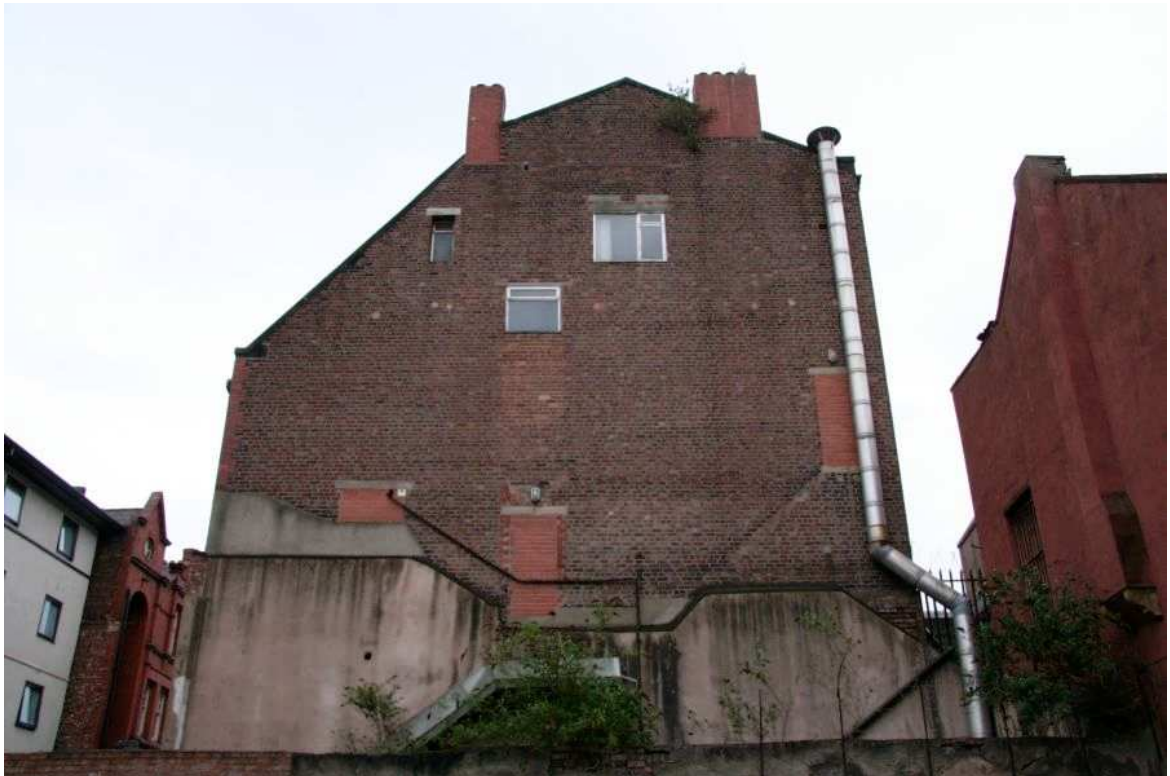
Plate 50: North-facing elevation of 67 Dale Street
