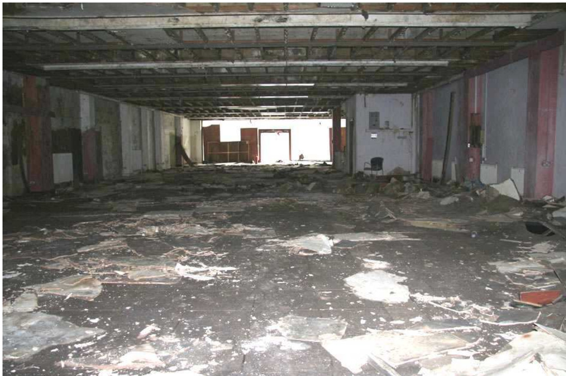
Plate 36: Ground floor of 61 Dale Street
