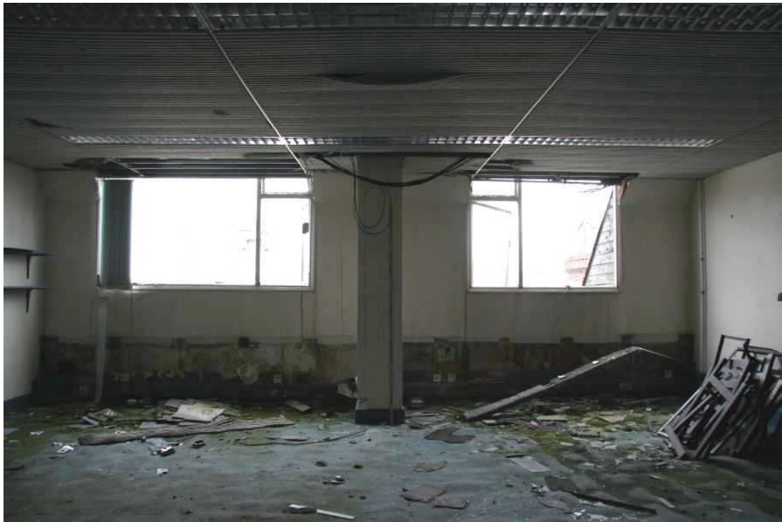
Plate 63: Windows in the east-facing elevation, fourth floor
