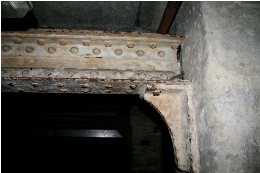
Plate 6: Basement I column and riveted steel joist detail
