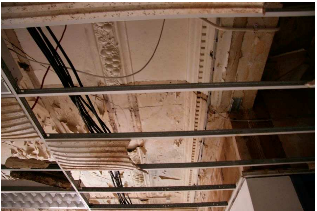
Plate 60: Original plaster moulding detail behind the suspended ceiling in Room 60
