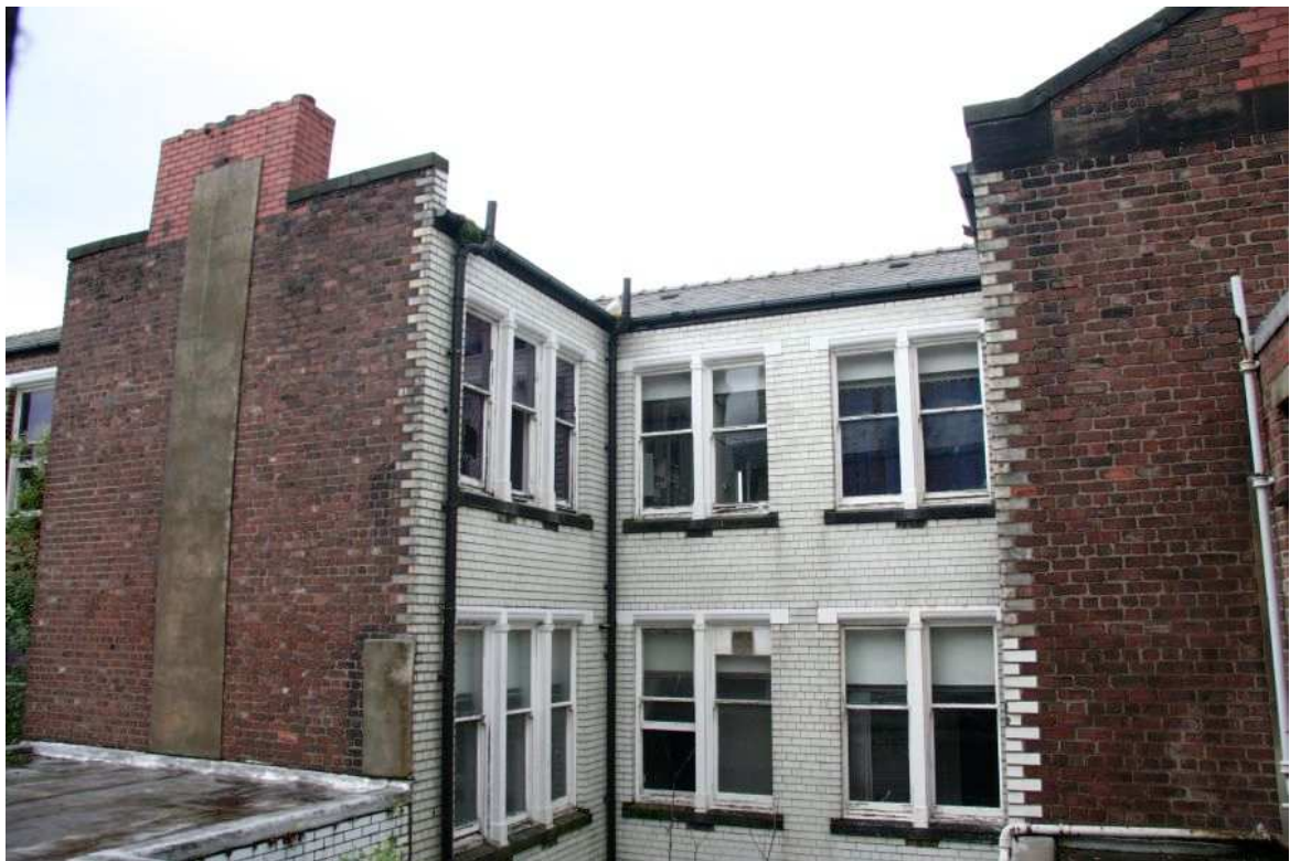
Plate 51: West-facing elevation of 67 Dale Street
