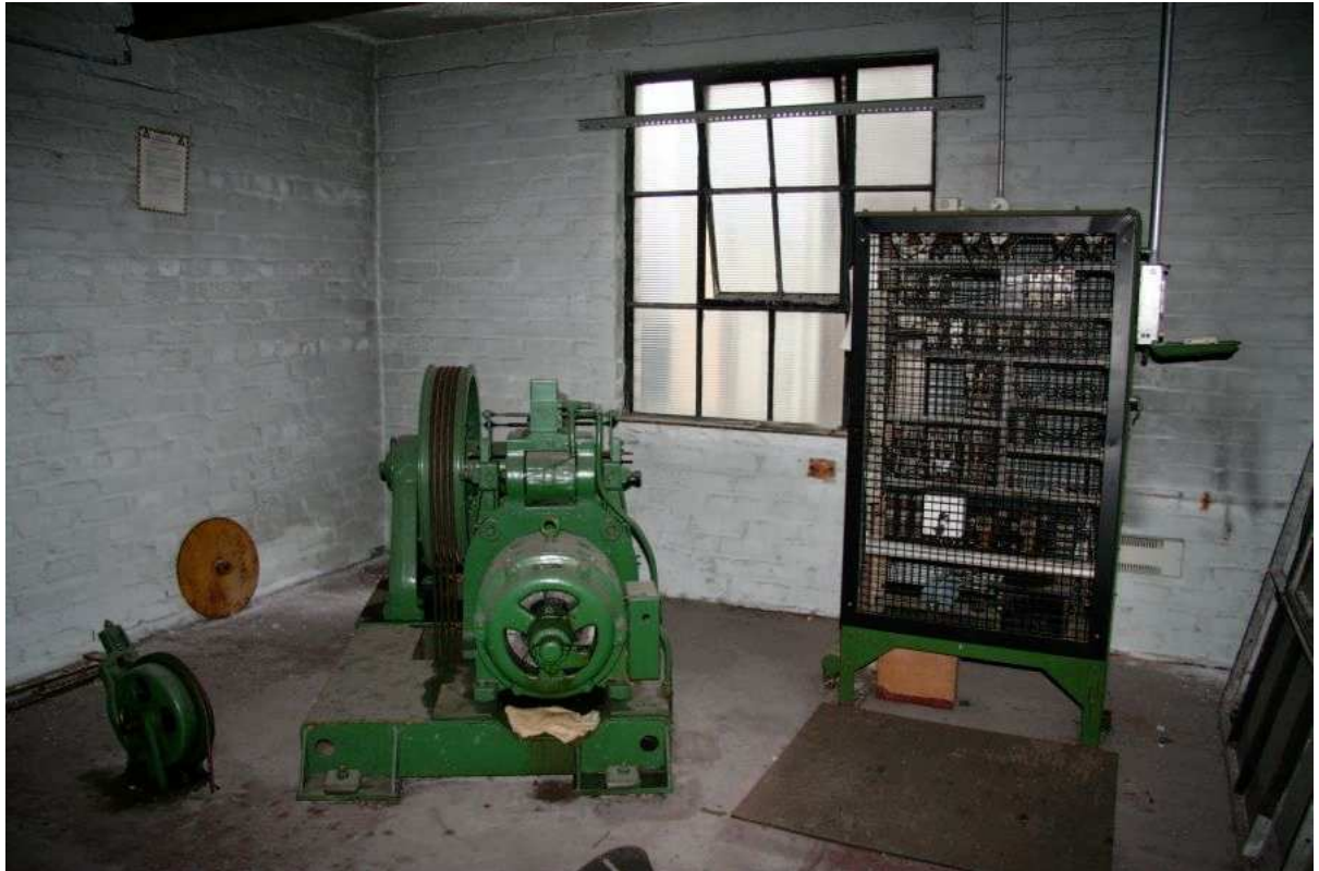
Plate 44: Fourth floor lifting gear in Room 35
