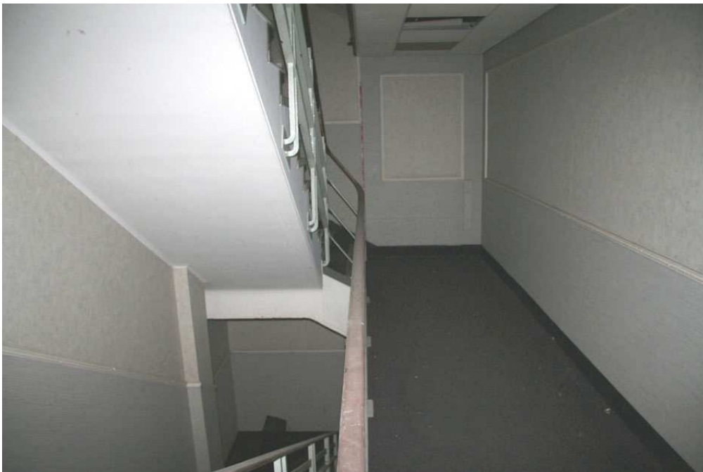
Plate 18: Stairwell 12 at rear of 57 Dale Street
