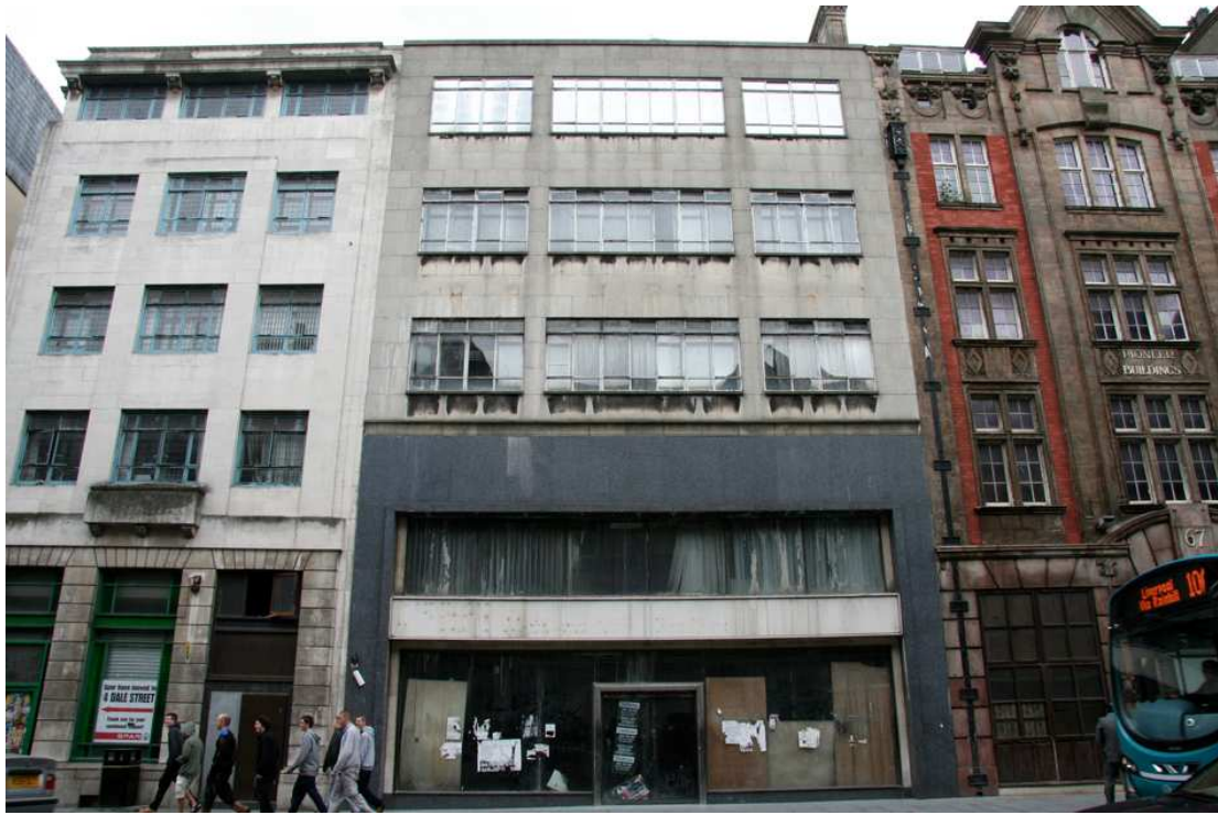
Plate 33: South-facing elevation of 61/63 Dale Street (centre)
