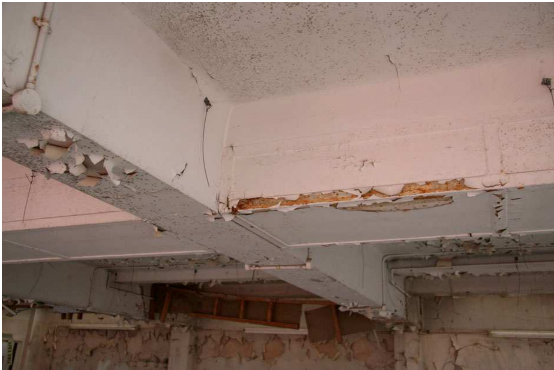
Plate 29: Detail of cross beams in ceiling
