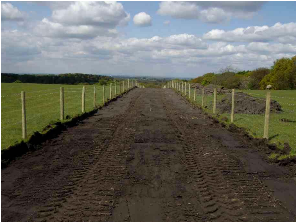
Plate 1: View of the access road illustrating the shallow nature of the topsoil strip
