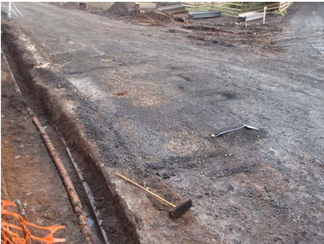
Plate 2: Cobbled surface revealed beneath the modern tarmac of the road junction
