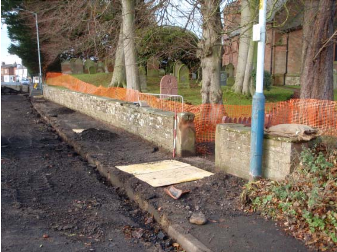
Plate 3: The southern church wall prior to removal
