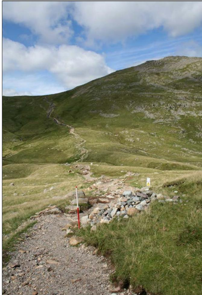
Plate 1: Footpath erosion to the north-west of Angle Tarn
