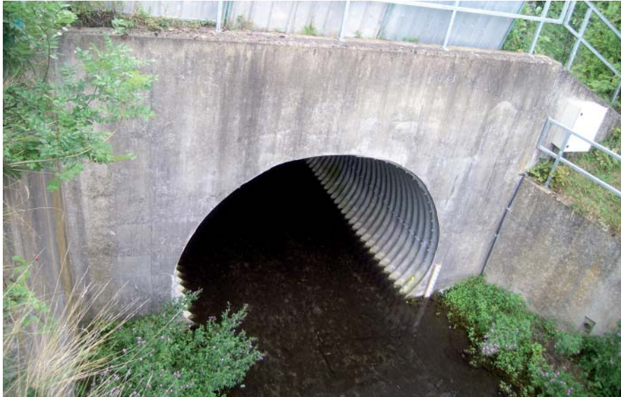
Plate 7: Entrance of river Misbourne culvert
