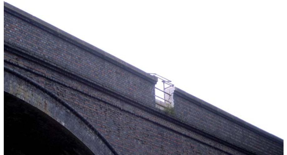
Plate 16: View of railing on parapet wall
