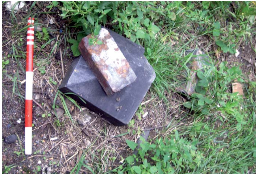
Plate 5: Detail of fallen bricks from north facing elevation
