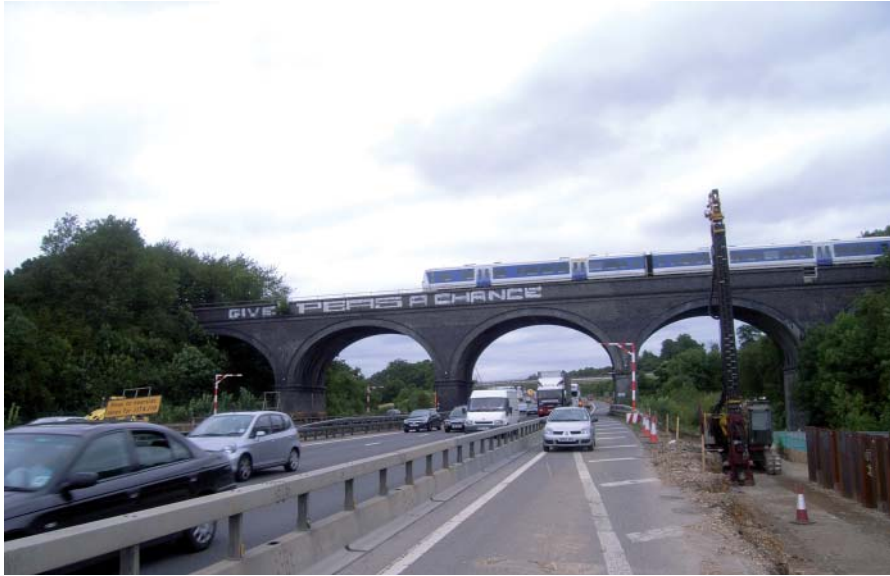
Plate 1: View of south facing elevation from M25 hard shoulder
