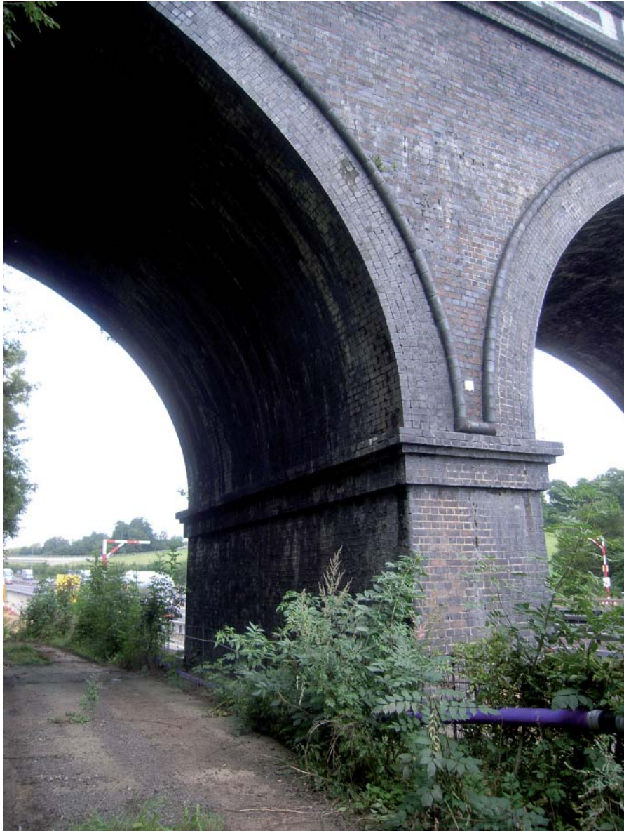
Plate 17: View of the track under the western arch of the viaduct
