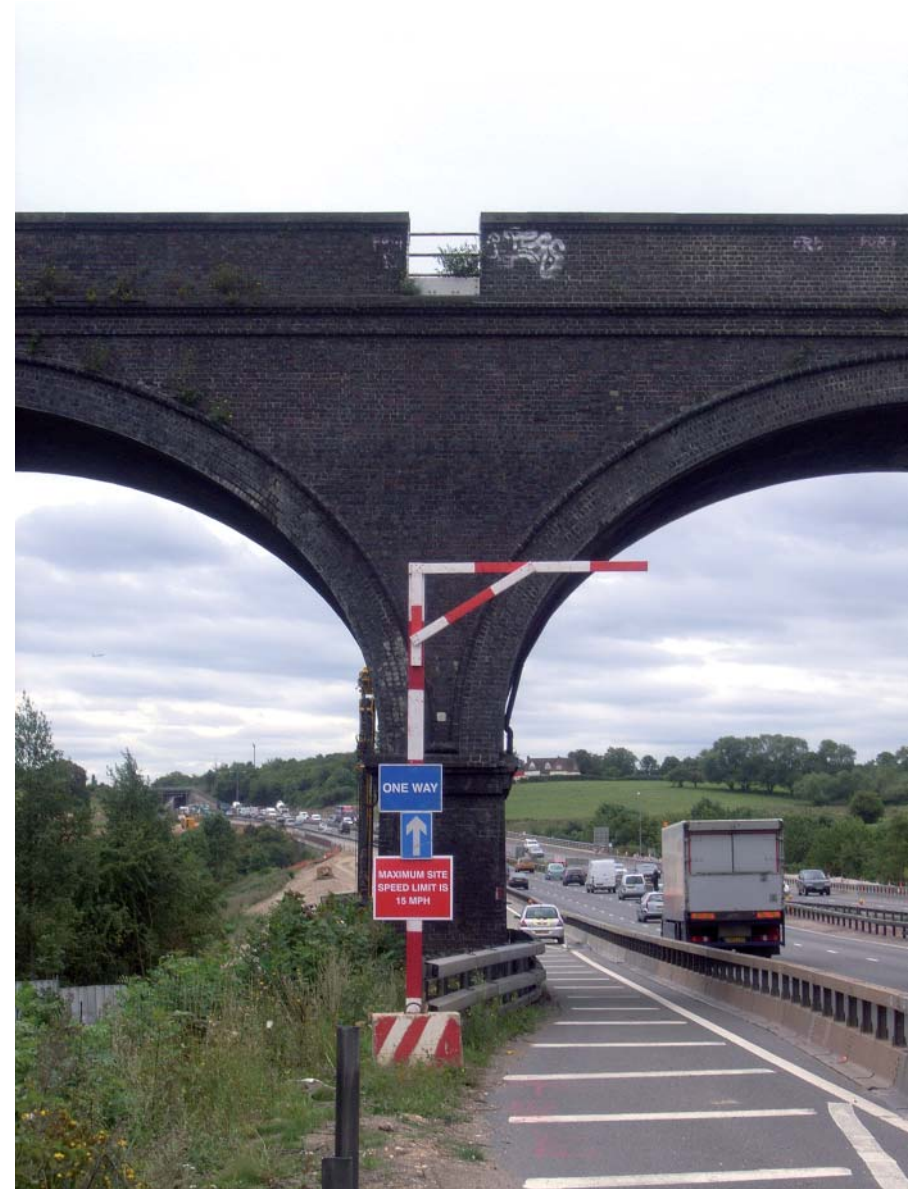
Plate 3: View of pier on north facing elevation
