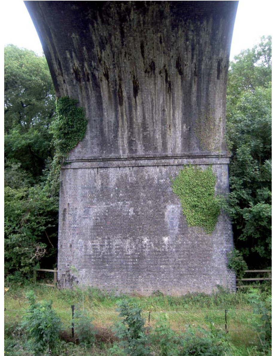
Plate 6: View of east elevation of pier
