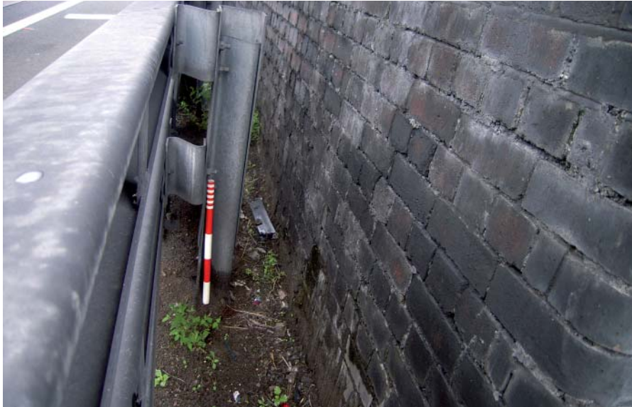
Plate 10: Detail of crash barrier
