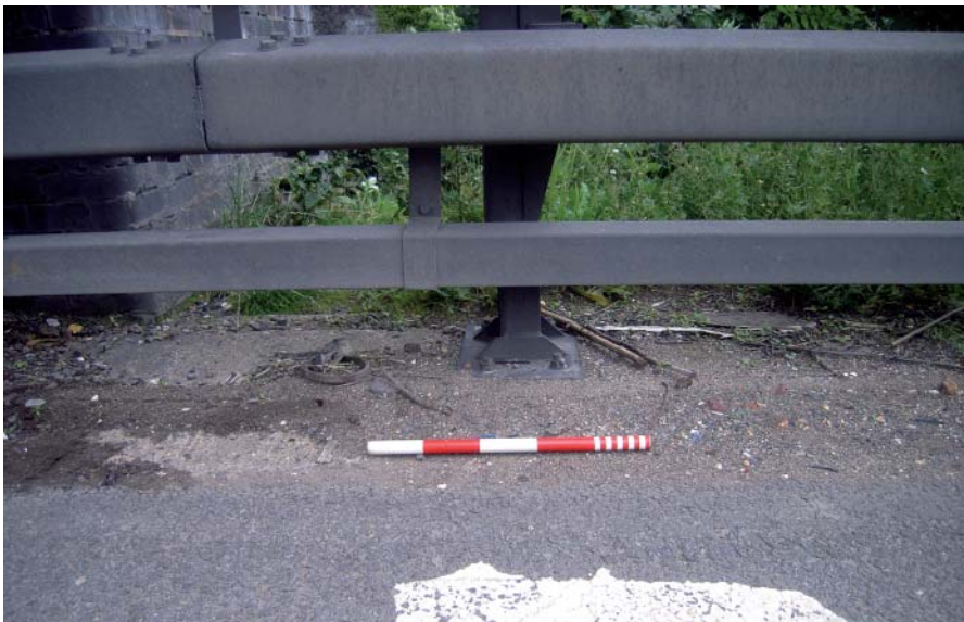
Plate 9: Detail of crash barrier ground surface
