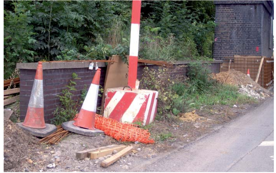
Plate 12: View of low brick wall
