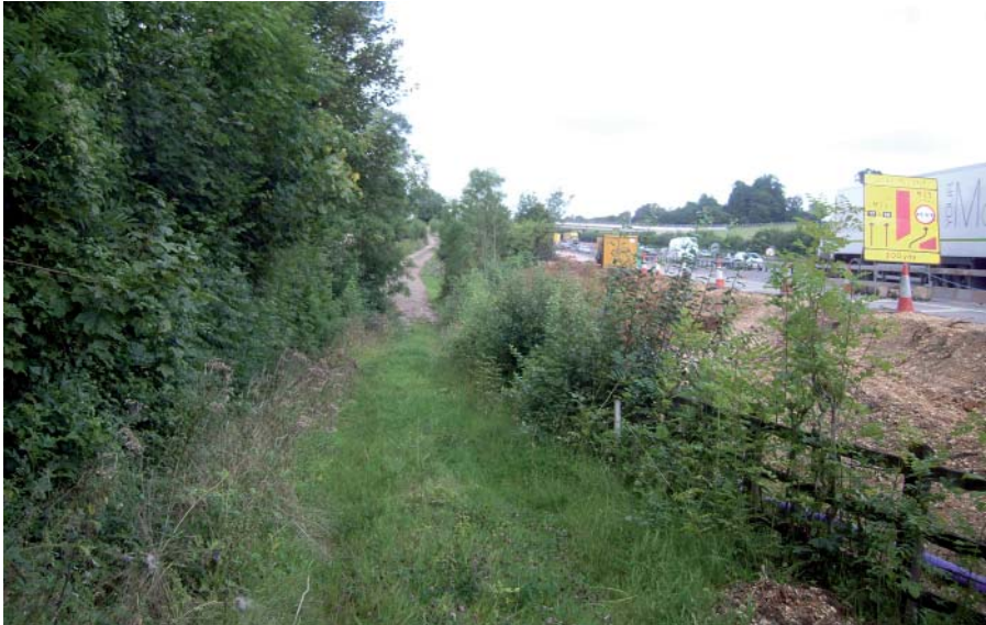
Plate 14: View of track to western end of viaduct
