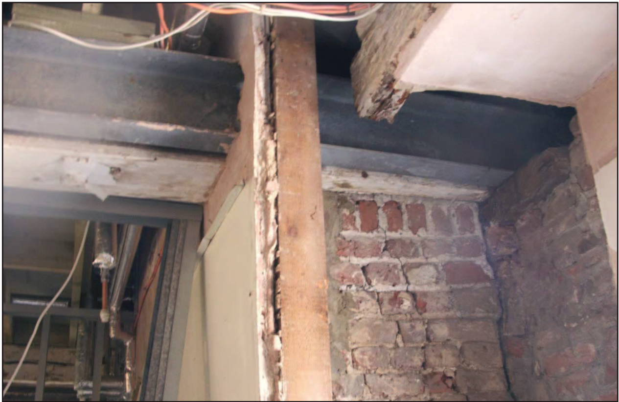
Plate 11: Exposed brickwork of chimney breast (centre right) and inner face of exterior north wall (extreme right)
