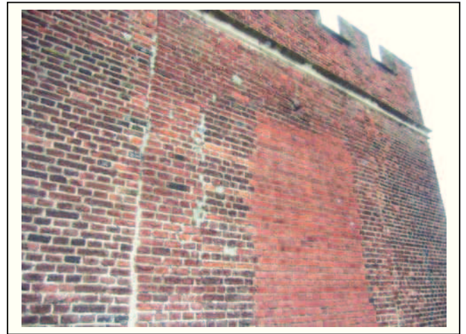
Plate 2: Blocked features on the south wall investigation focused on the area above the large blocked window.
