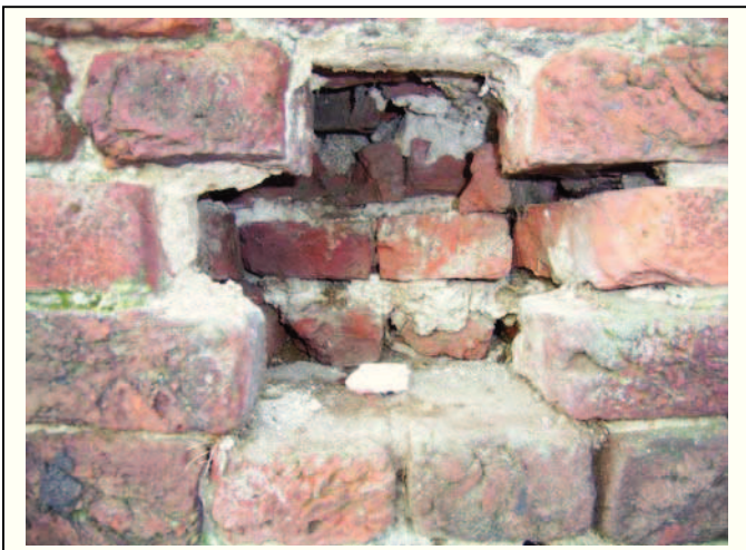
Plate 3 External intervention showing core of south wall.
