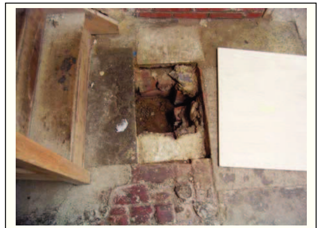
Plate 4: Raised slab in basement showing drain beneath.
