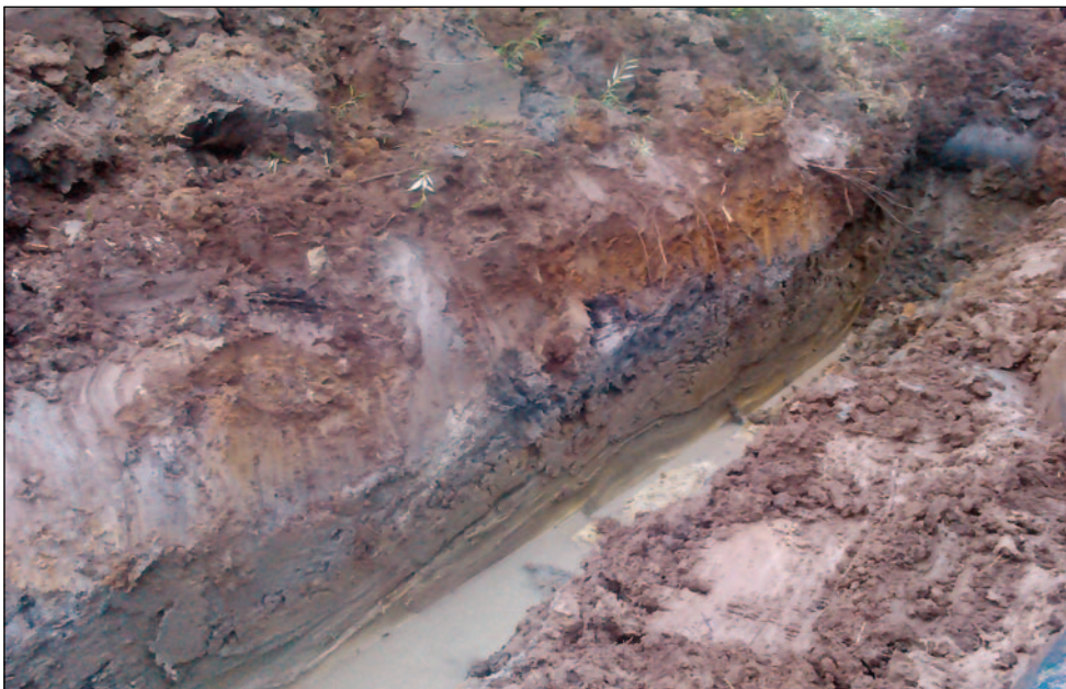
Plate 2: Digging adjacent to the Brook
