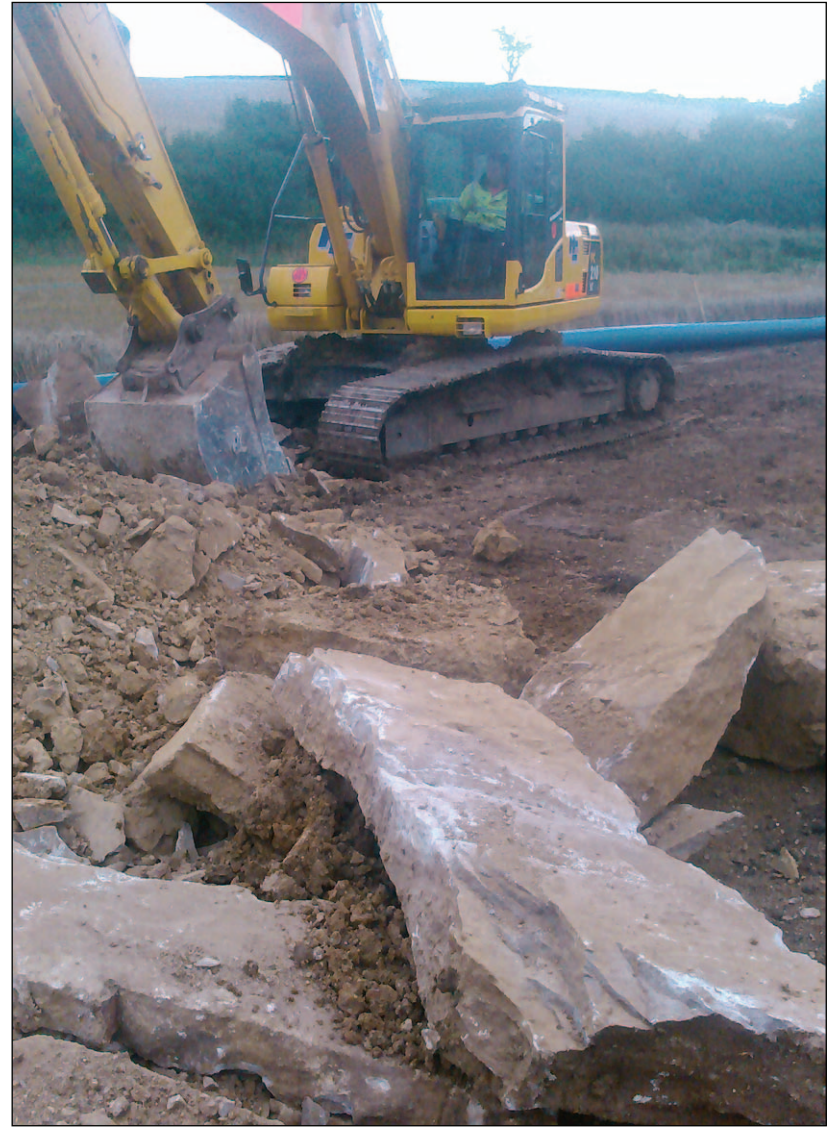
Plate 4: Laying pipe in area 3
