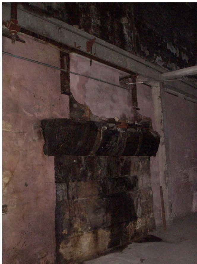
Plate 8: Footstep bearing for vertical driveshaft, Building 1
