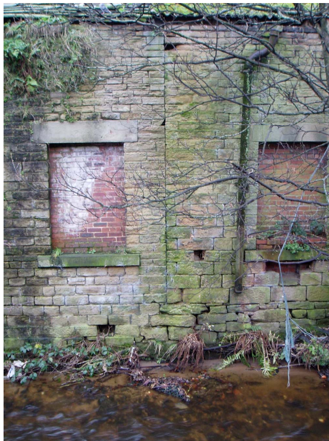
Plate 16: Butt joint between phases, Building 3
