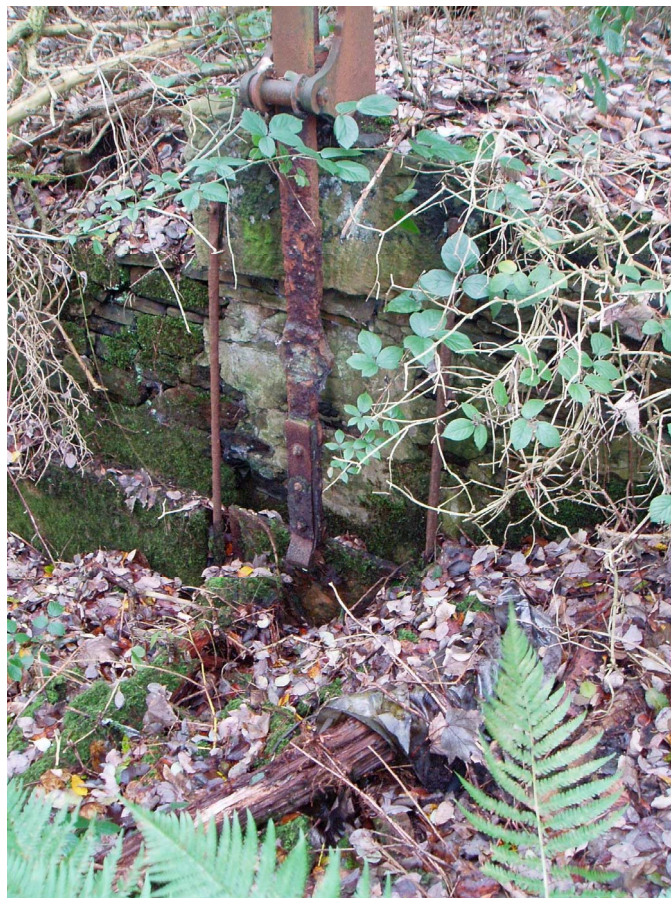
Plate 50: Remains of sluice gate, central mill pond
