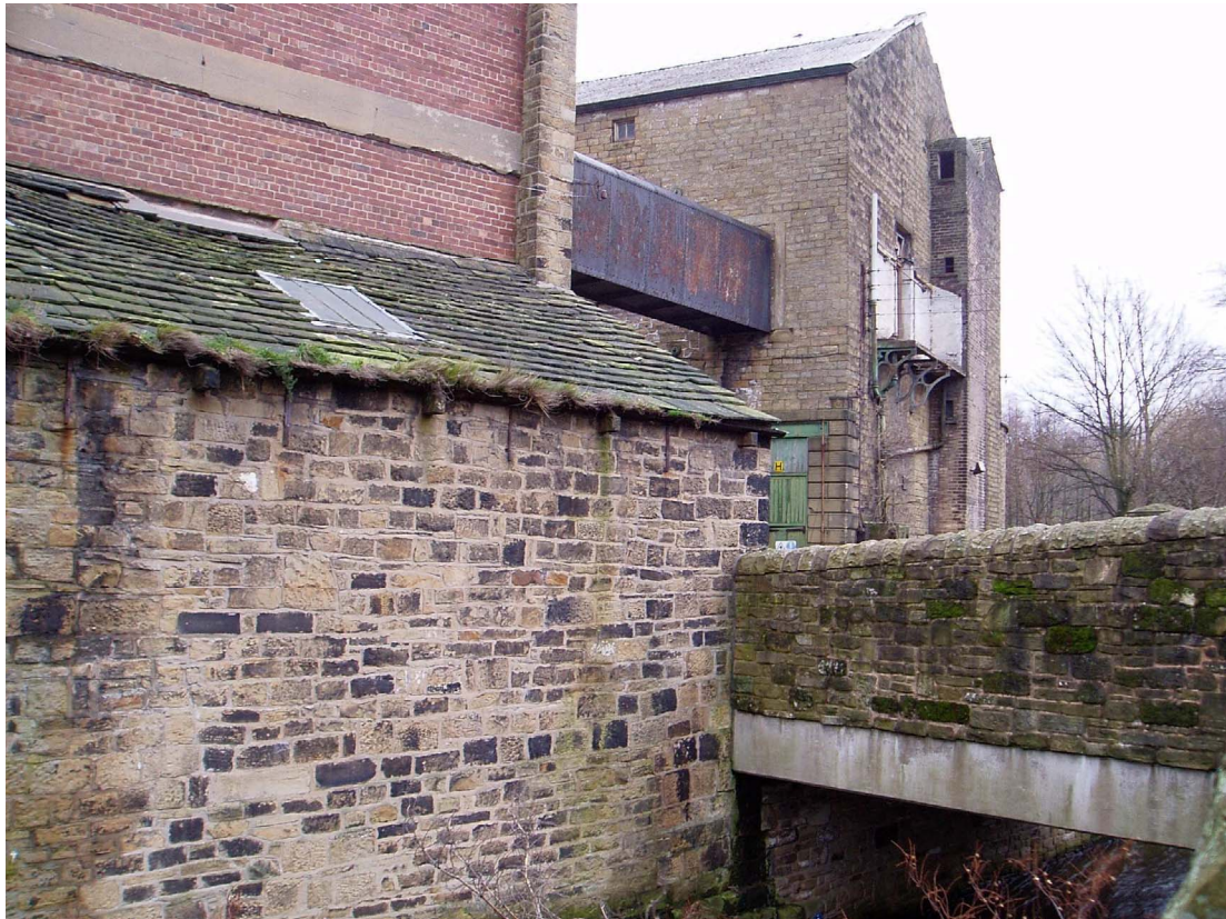
Plate 15: Detail of projecting corbels, Building 3
