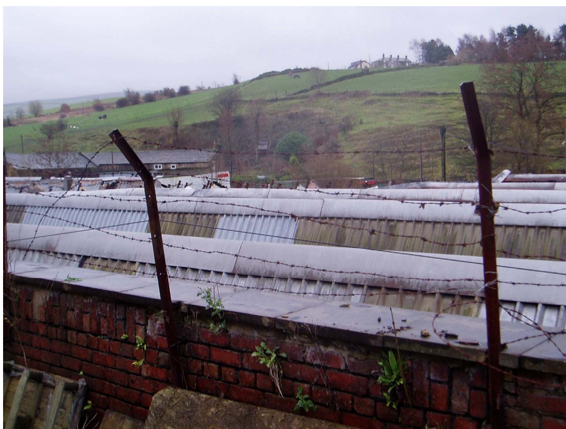
Plate 40: Multiple-span north-light roof, Building 17
