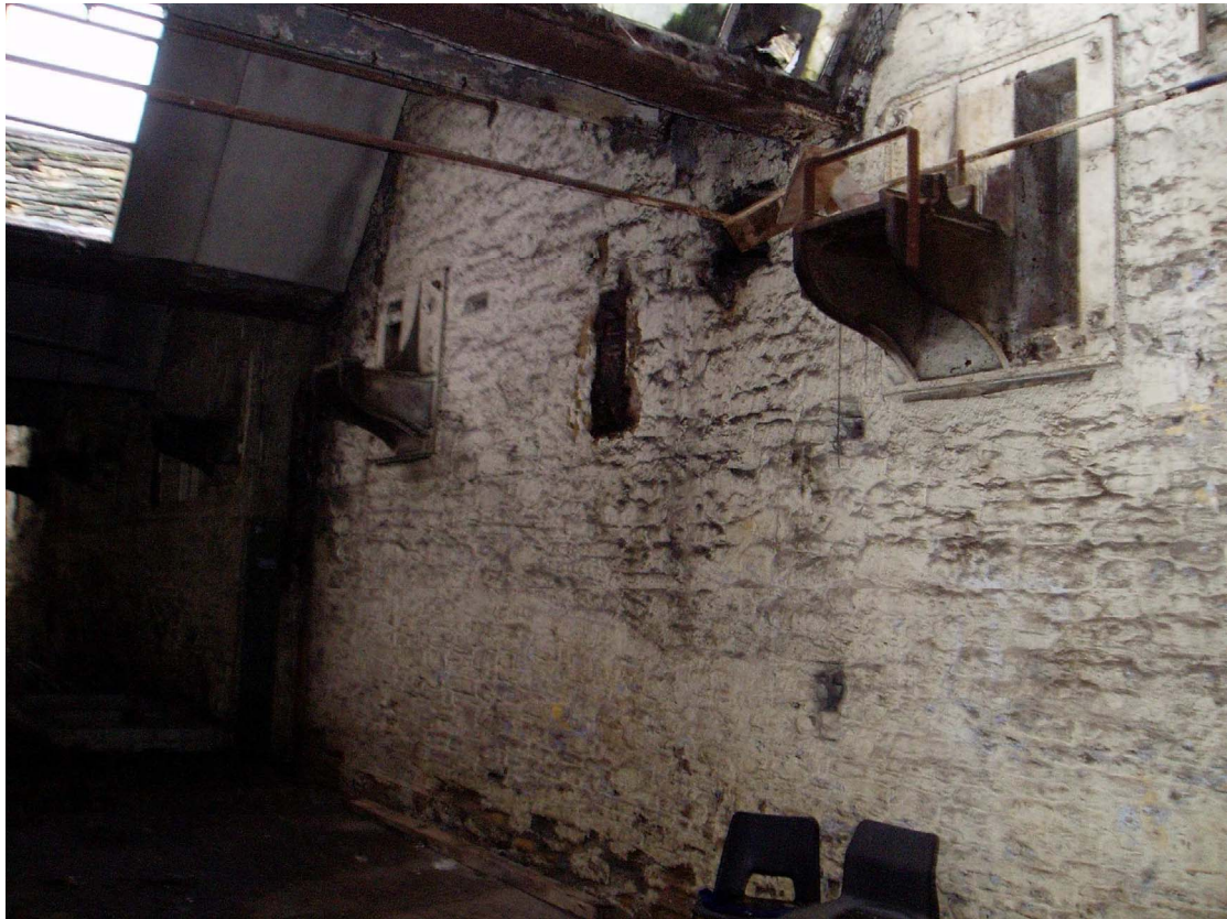
Plate 27: Lineshaft-carrier bearing, east elevation, Building 7
