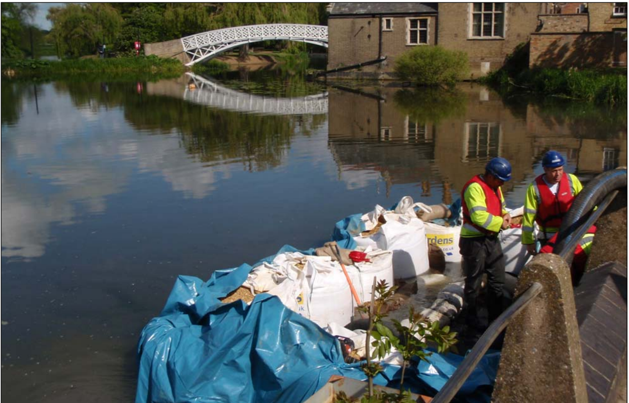
Plate 6: Causeway Test Pit 1 during excavation
