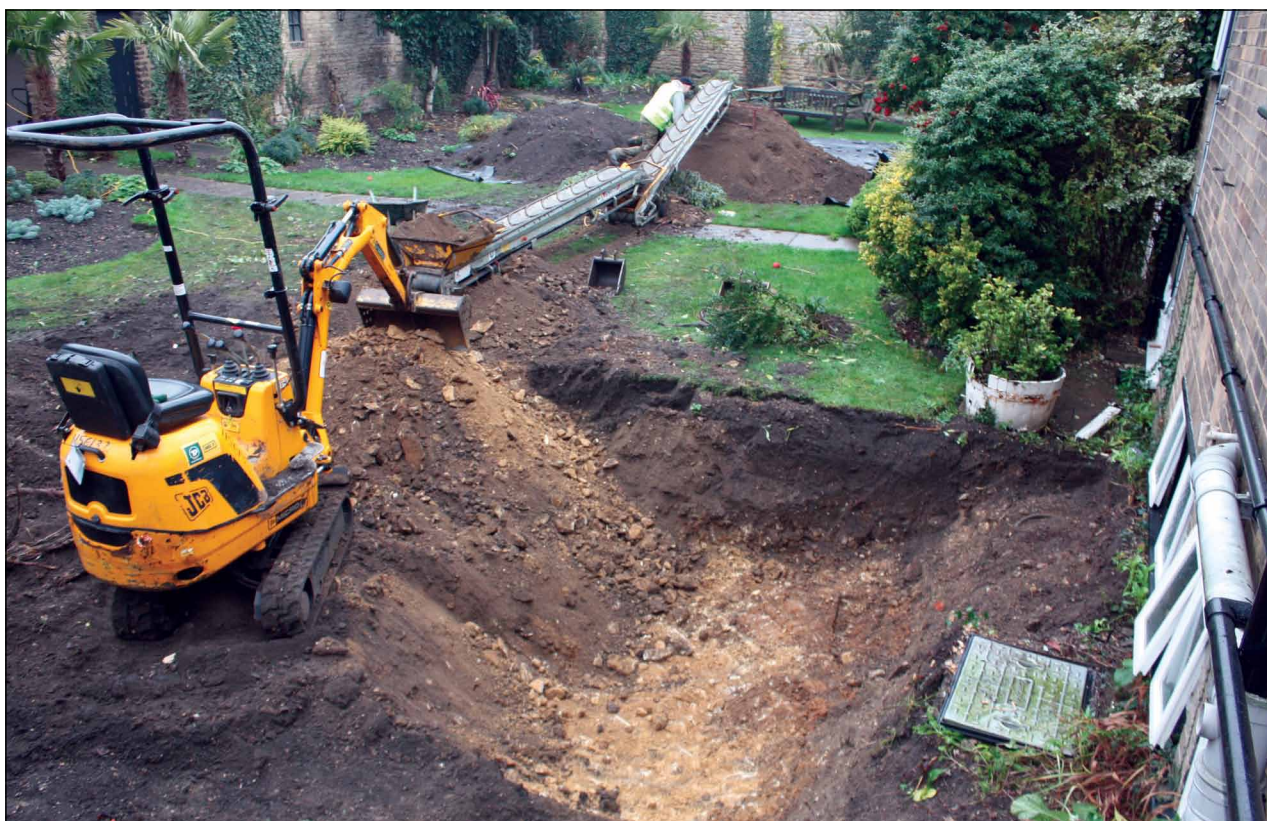
Plate 1: Ground reduction at the rear of the hotel
