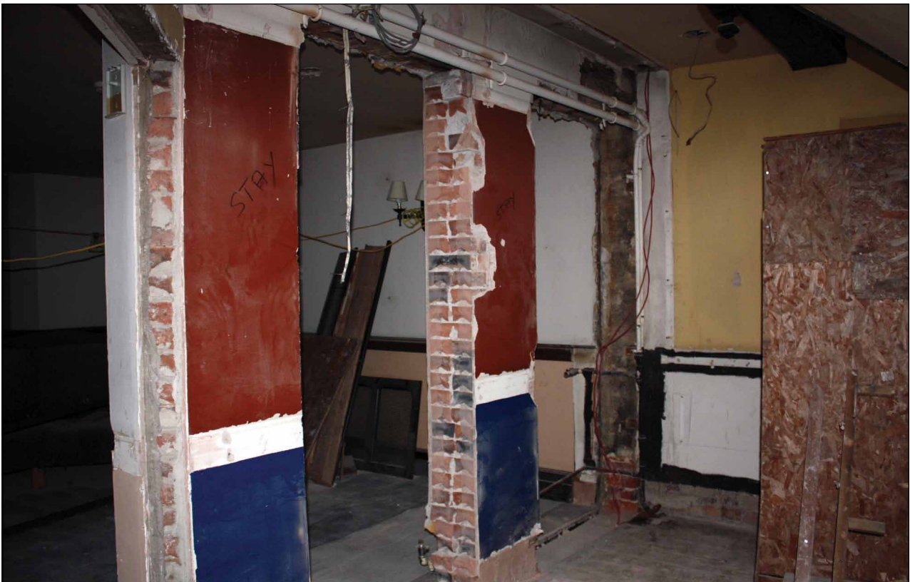
Plate 23: Reinstated opening between stairs and bar, taken during alteration works
