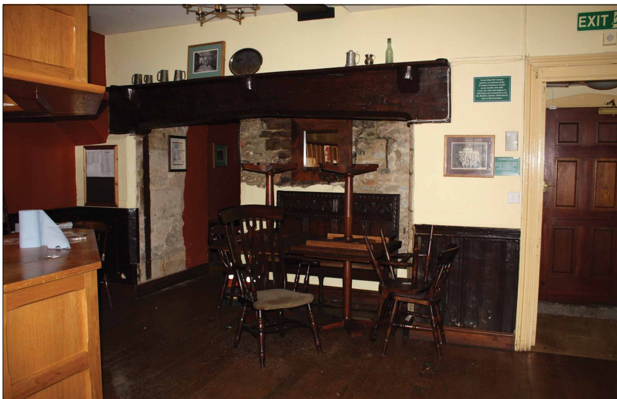
Plate 4: Large bressumer, viewed from front bar
