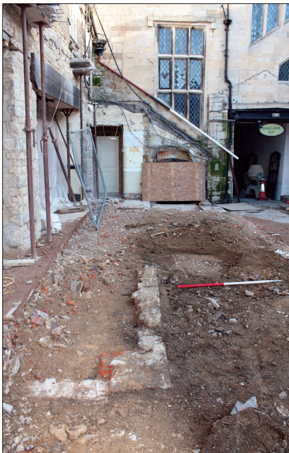
Plate 71: Foundations and cobbled surface in courtyard exposed during external alterations
