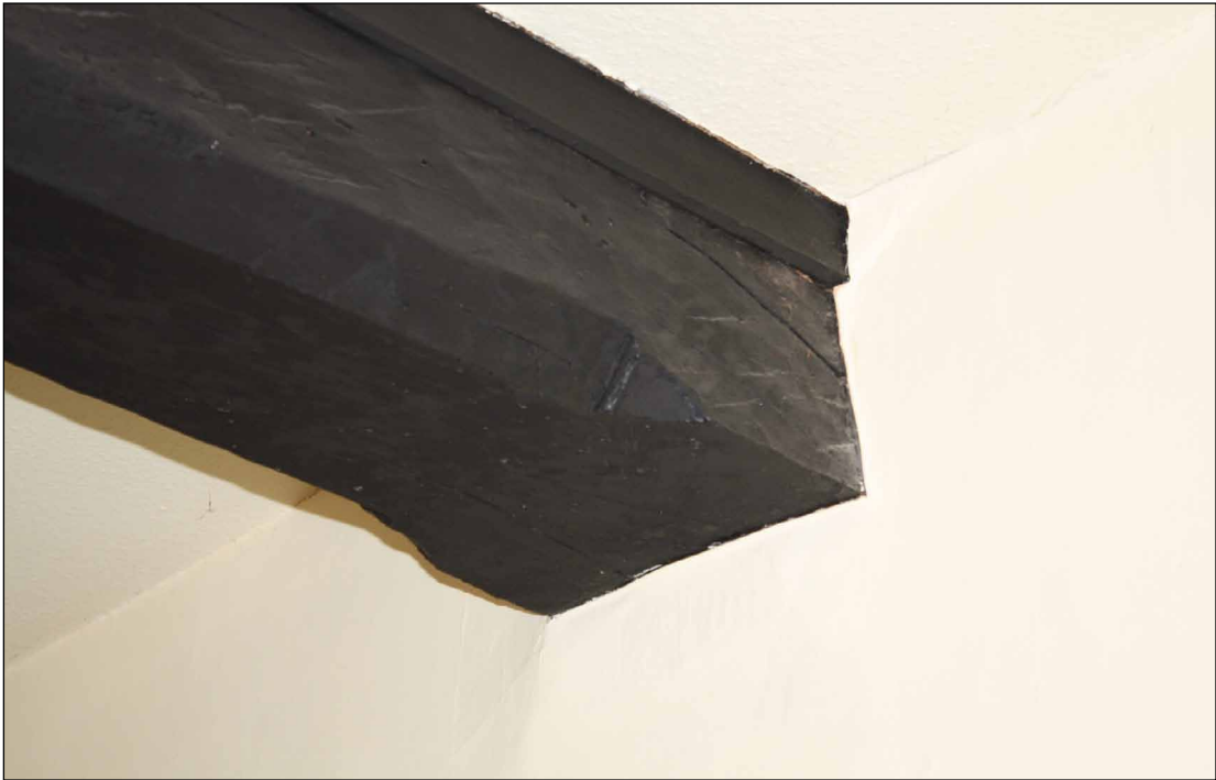
Plate 53: Detail of stop-chamfered beam in Tabret Room
