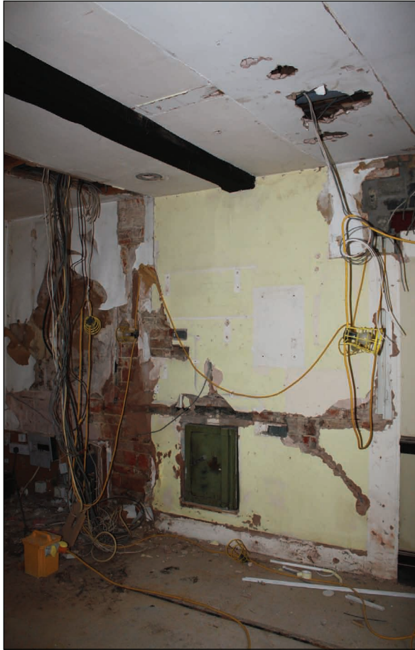
Plate 41: Safe inserted into former fireplace, exposed during building alterations
