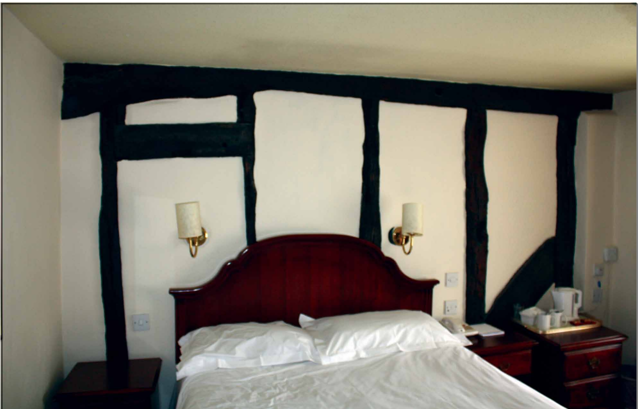
Plate 30: Exposed timber frame in first floor guest bedroom
