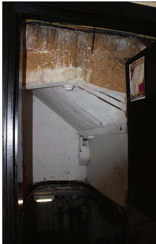
Plate 25: Detail of stone arch over access to cellar
