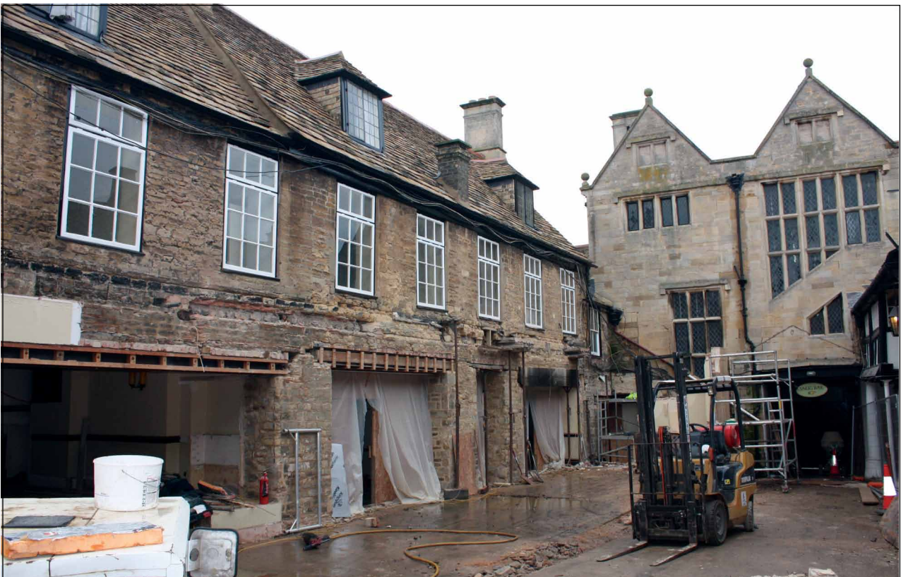
Plate 48: Exposed façades of Buildings 5 and 7 following removal of 1949 extension
