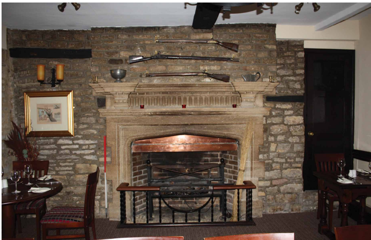
Plate 35: Blocked up doorway and later fireplace within restaurant
