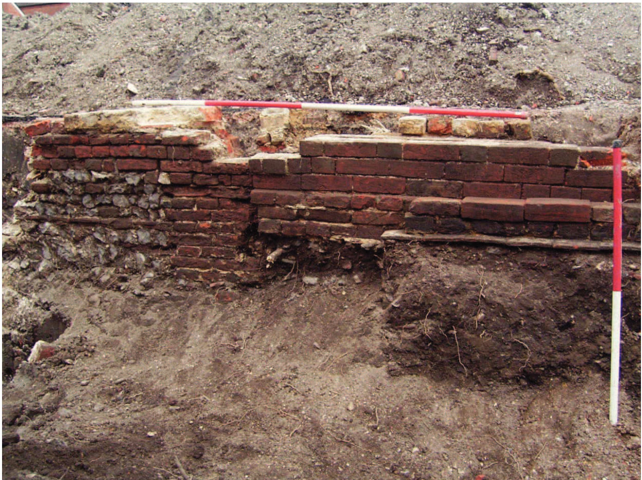
Plate 27: Wall 2001 showing different builds and dates of brickwork
