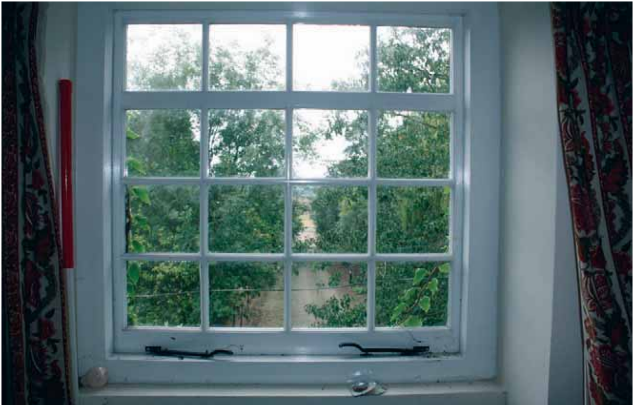
Plate 58: Internal detail of window, looking west along access road, F3
