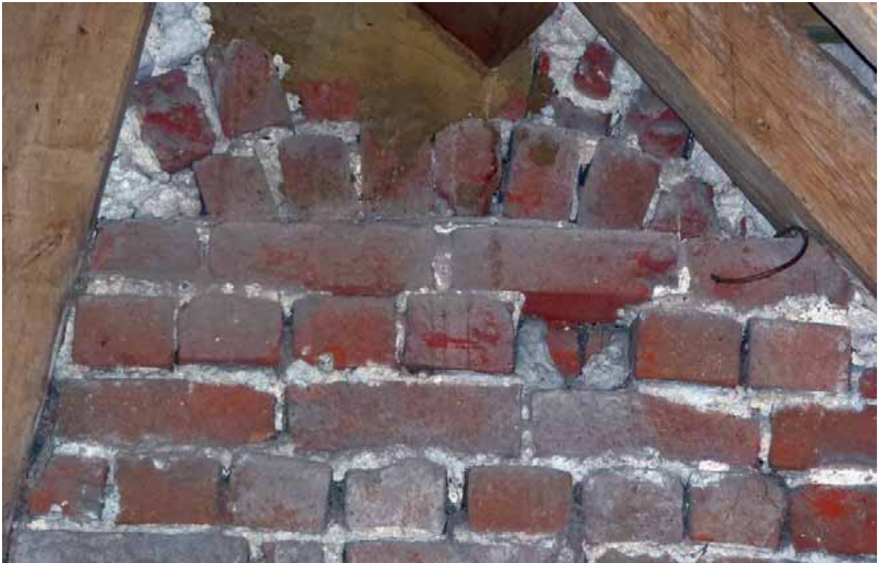
Plate 46: Internal detail of roundel brickwork
