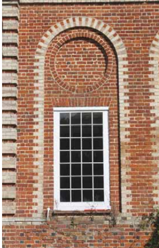
Plate 4: Detail of window on south-facing elevation
