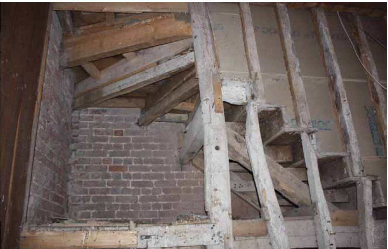
Plate 33: Detail of modern alteration to staircase
