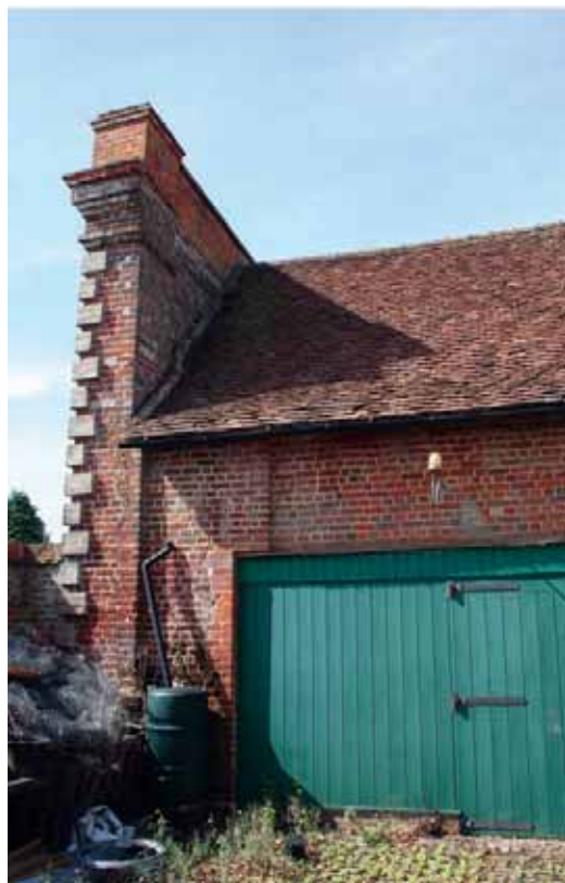
Plate 13: Detail of raised parapet from north-east
