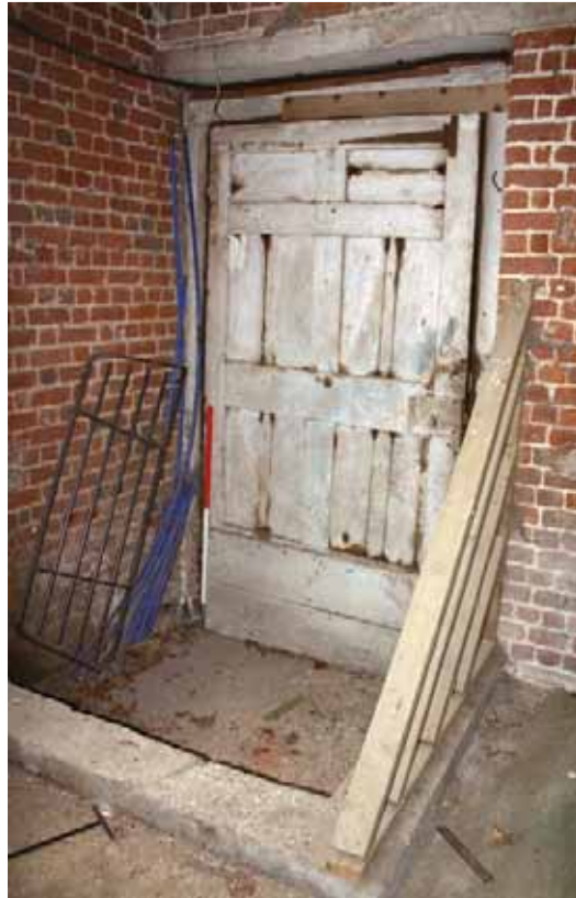
Plate 36: Internal view of door showing reduced ground level, G4
