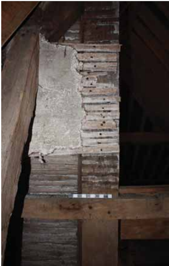
Plate 75: Detail of lath and plaster screen in roof space 1
