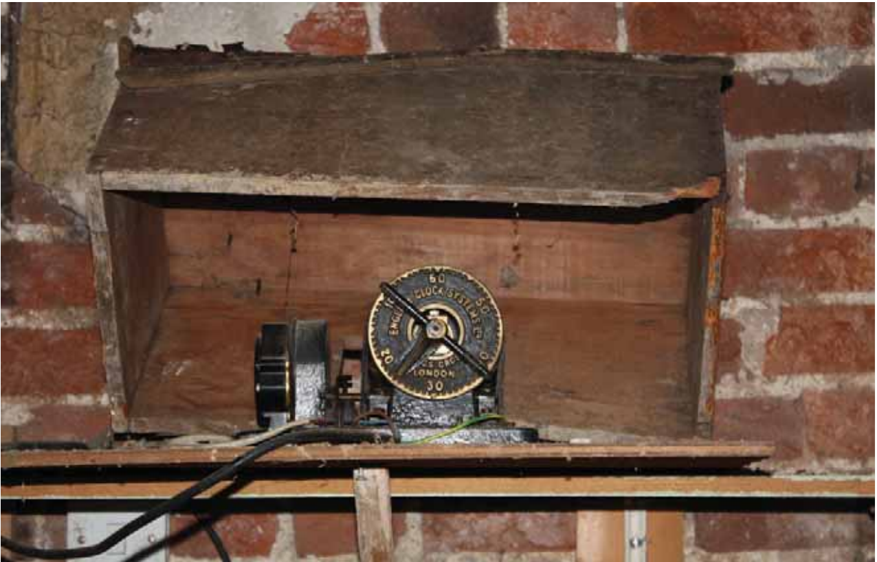
Plate 80: Clock mechanism, roof space 1
