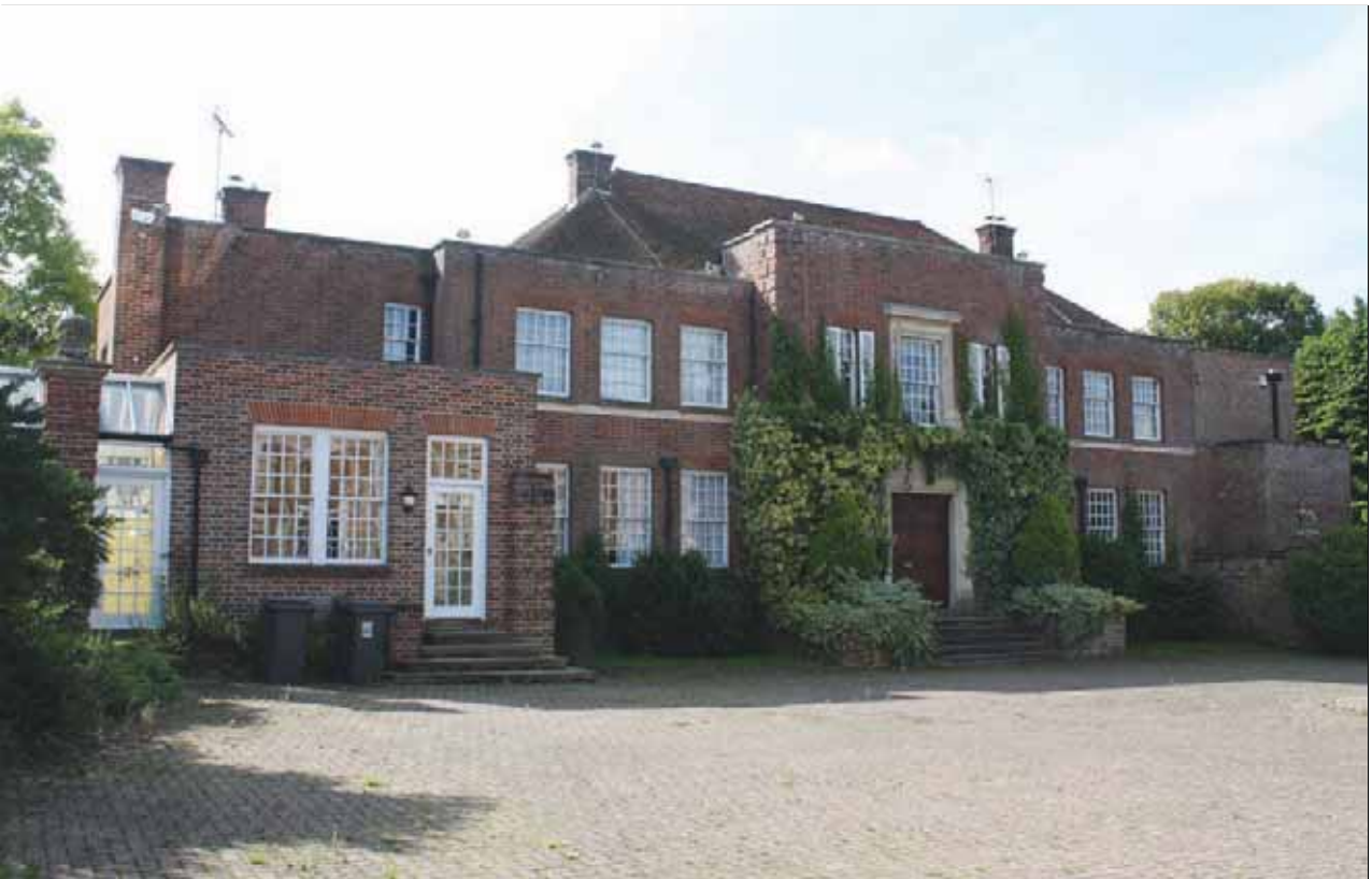
Plate 2: Broadfield Hall from northeast
