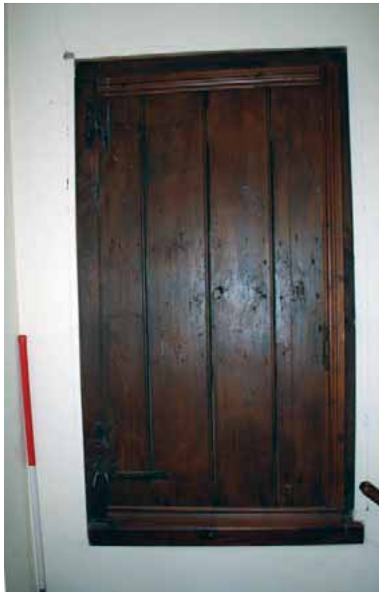
Plate 67: Access door from F7 into G4 roof space
