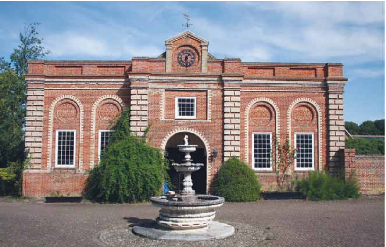
Plate 1: Broadfield Hall Stables, southern elevation
