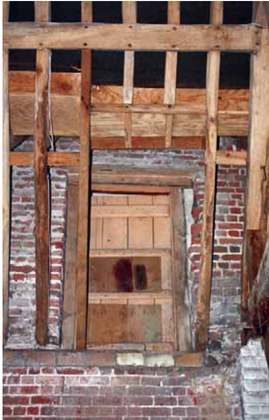
Plate 40: Detail of access door from F7 into roof space of G4
