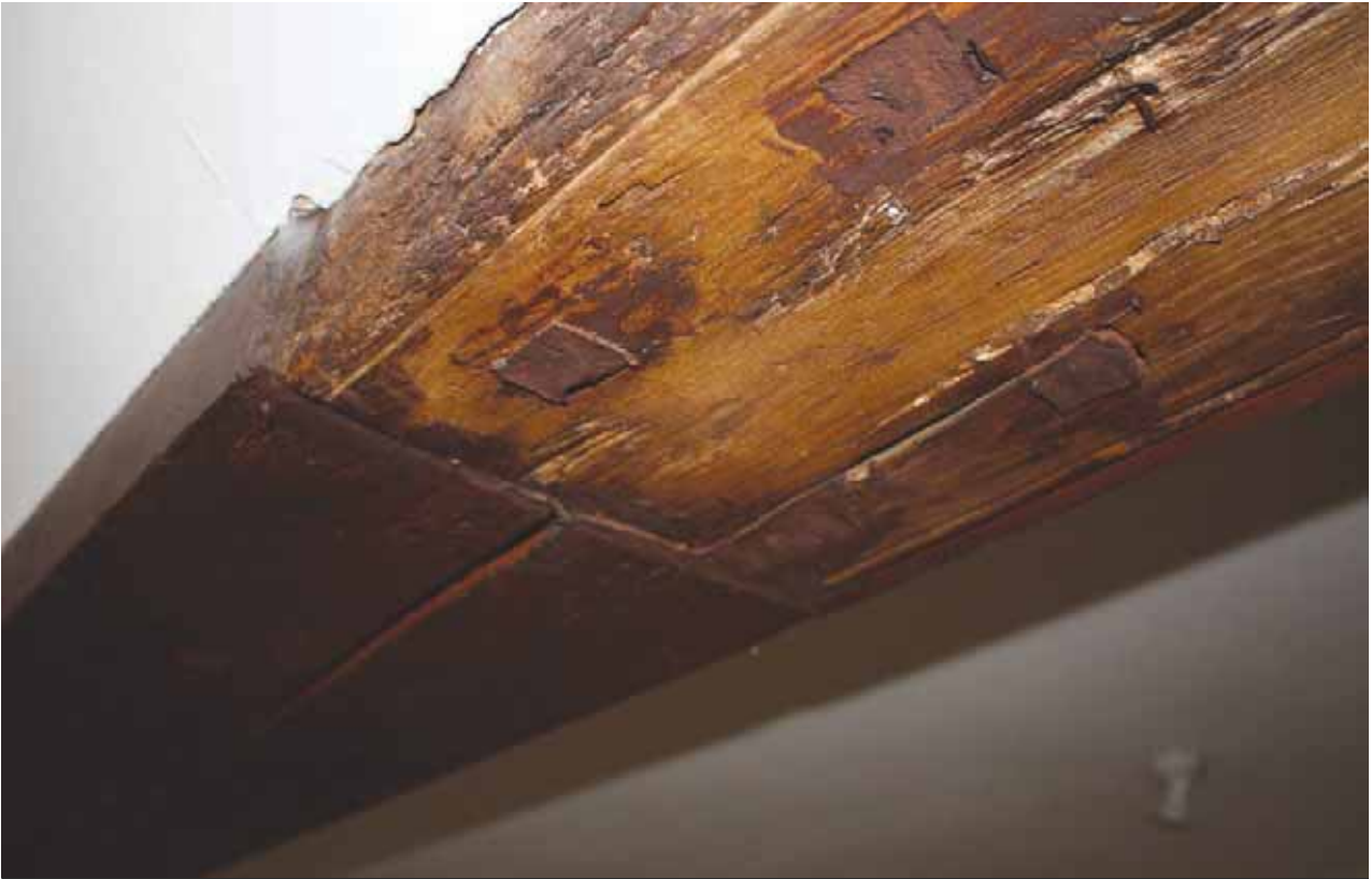
Plate 56: Detail of repair/replacement of moulded tie beam and filled square peg holes
