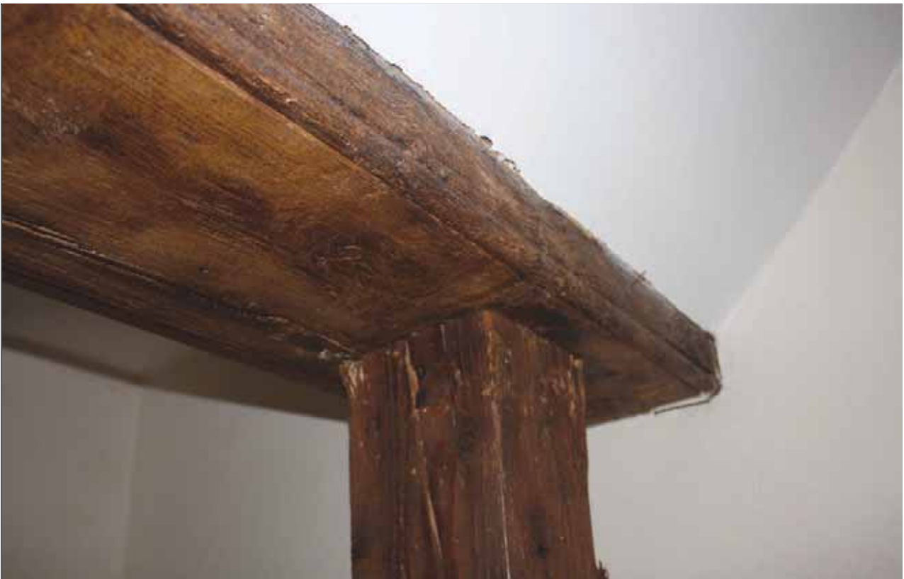
Plate 55: Detail of support post and tie-beam, F3
