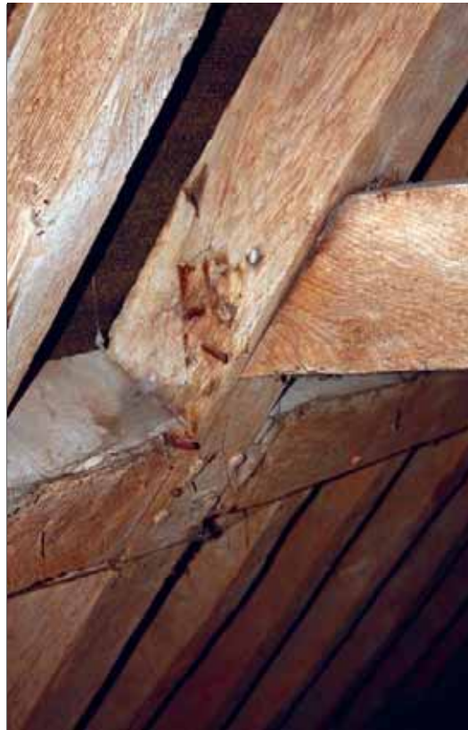
Plate 72: Half-lap joint connecting the principal rafter and purlin
