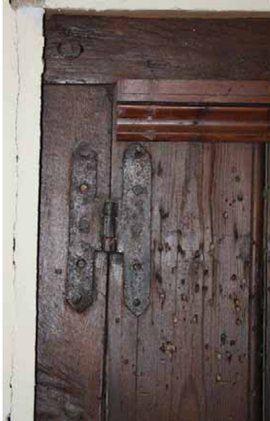
Plate 68: Detail of "H" hinge on access door, F7
