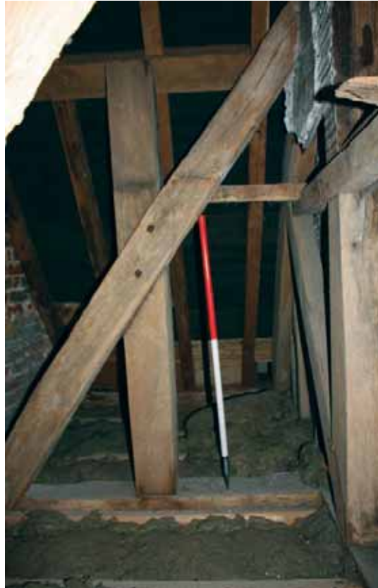
Plate 76: Diagonal and upright posts behind pediment at southern end of roof space 1
