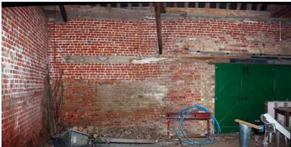
Plate 47: West-facing internal elevation, G4 (using "Autostitch")
