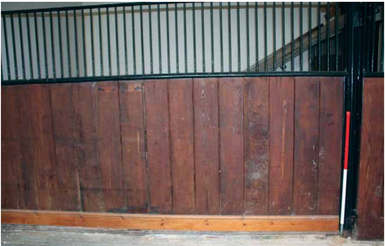
Plate 23: Detail of loose box screen, G1
