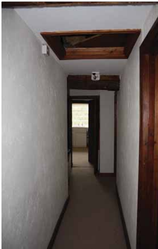
Plate 63: View along first floor corridor, F6
