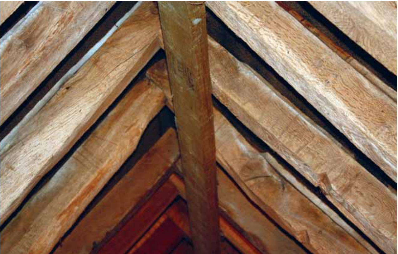
Plate 71: Detail of roof ridge showing carpenter's marks on common rafters
