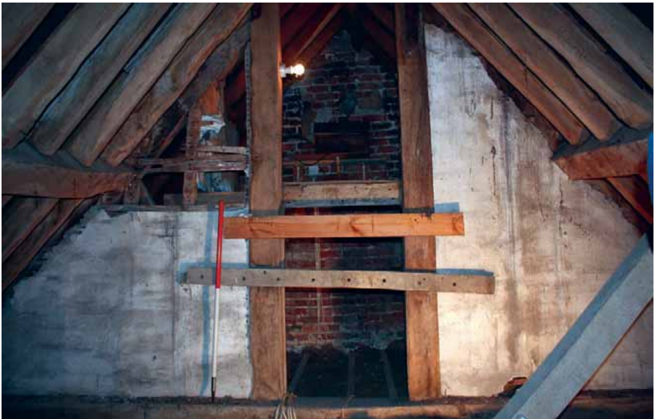
Plate 73: View of roof space 1, looking southwards
