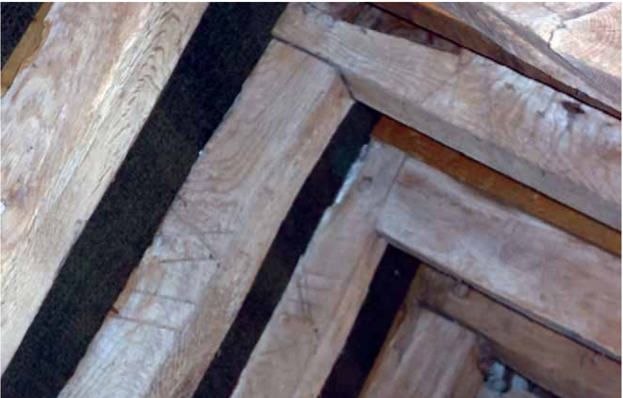
Plate 81: Common rafters with carpenter's marks, roof space 2
