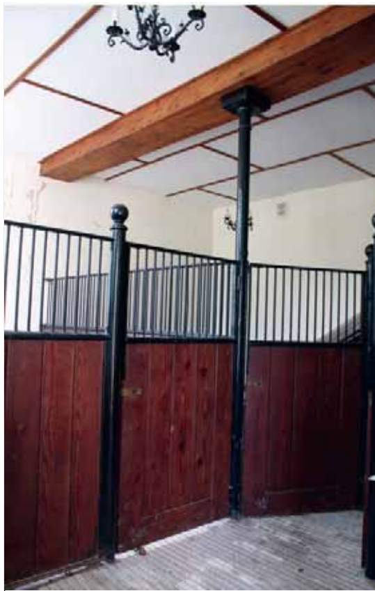
Plate 21: Internal view of G1 showing loose-boxes, ceiling joist and iron support post
