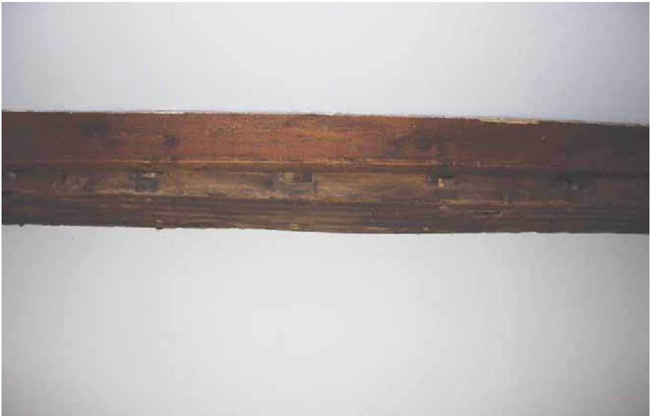
Plate 53: Detail of empty mortices, F2
