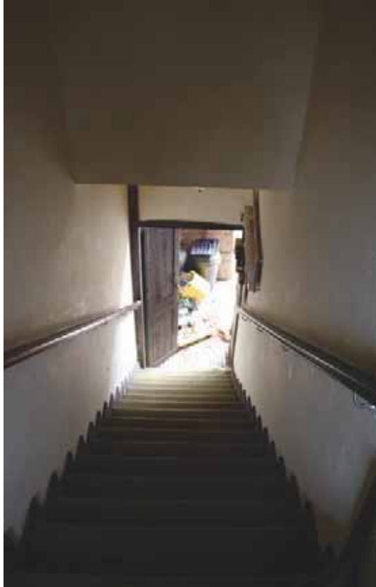
Plate 66: View from top of stairs, F7
