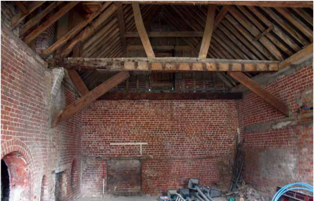
Plate 44: View of south-facing internal elevation, G4
