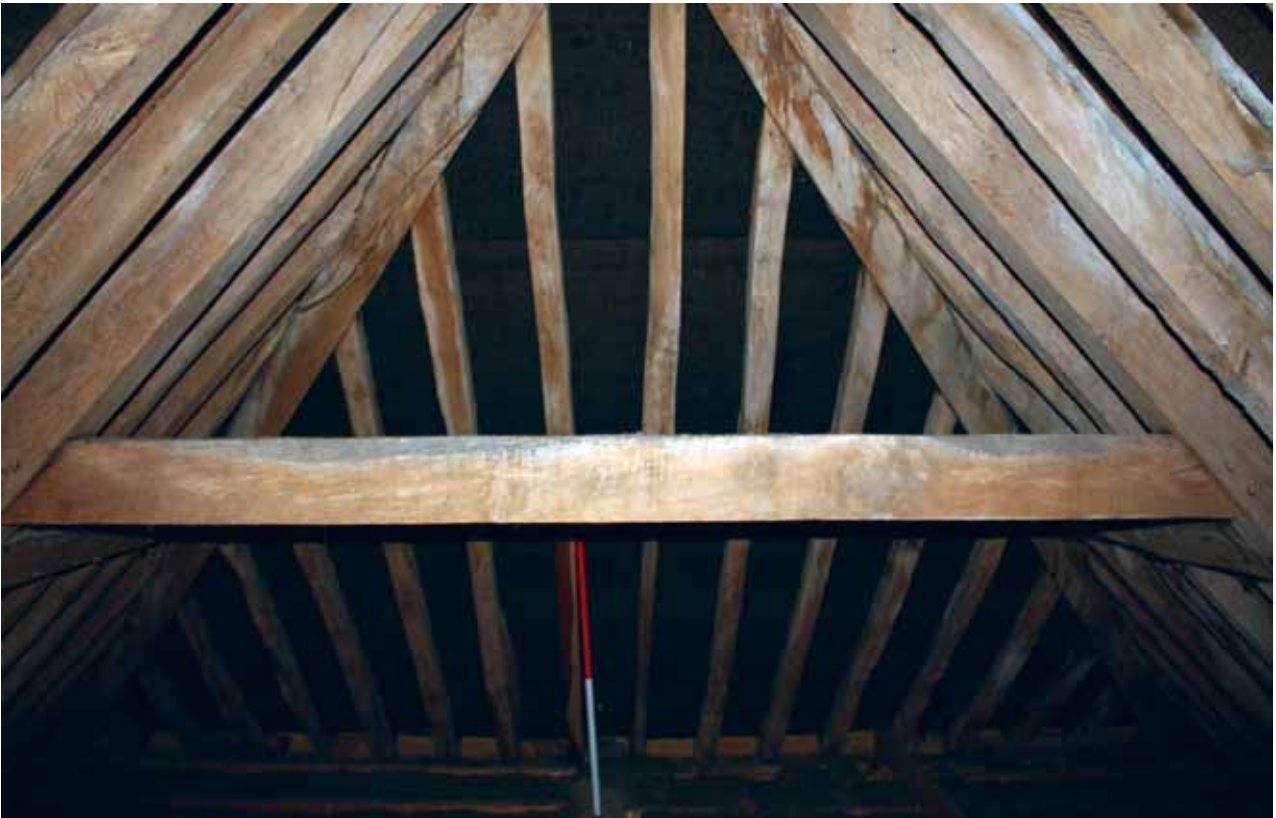
Plate 70: Detail of hipped roof
