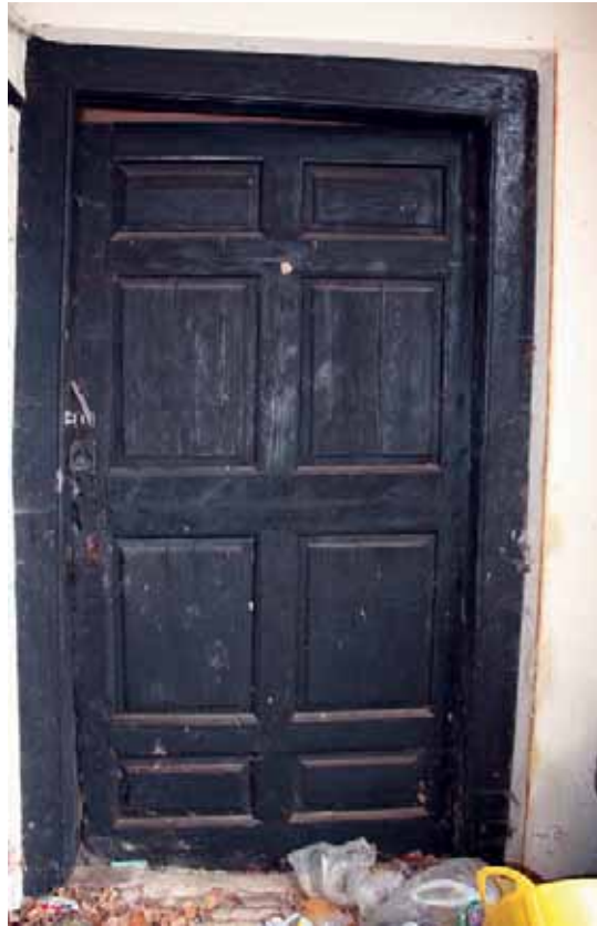
Plate 20: External door leading into G3
