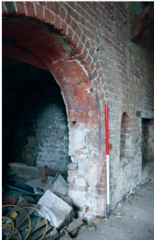
Plate 43: Detail of archway leading from G4 into G5
