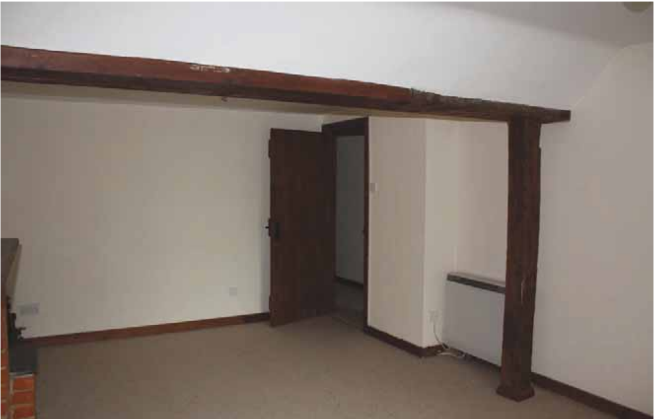
Plate 54: General room view, F3
