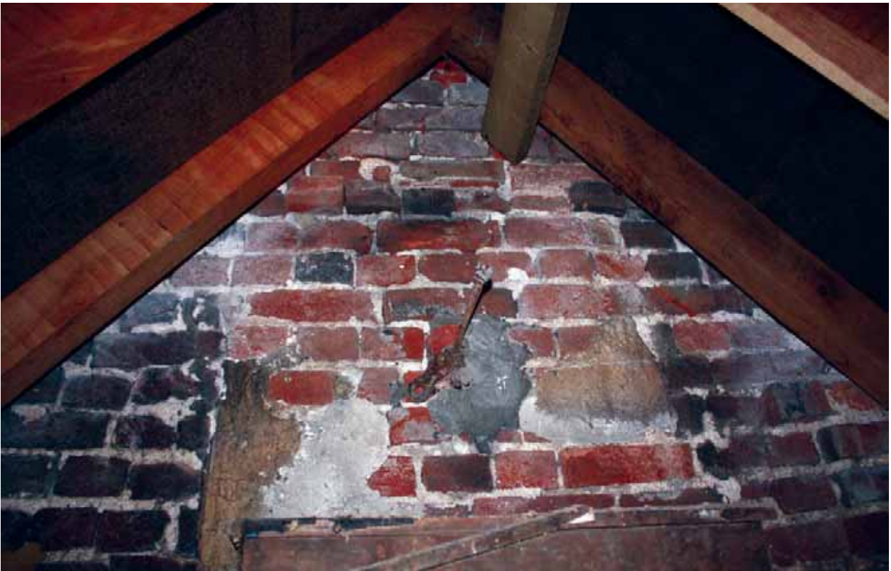
Plate 79: Detail of raised pediment brickwork from inside roof space 1
