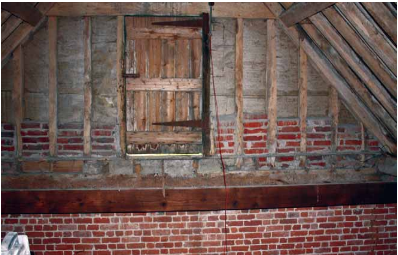
Plate 45: Detail of loading door
