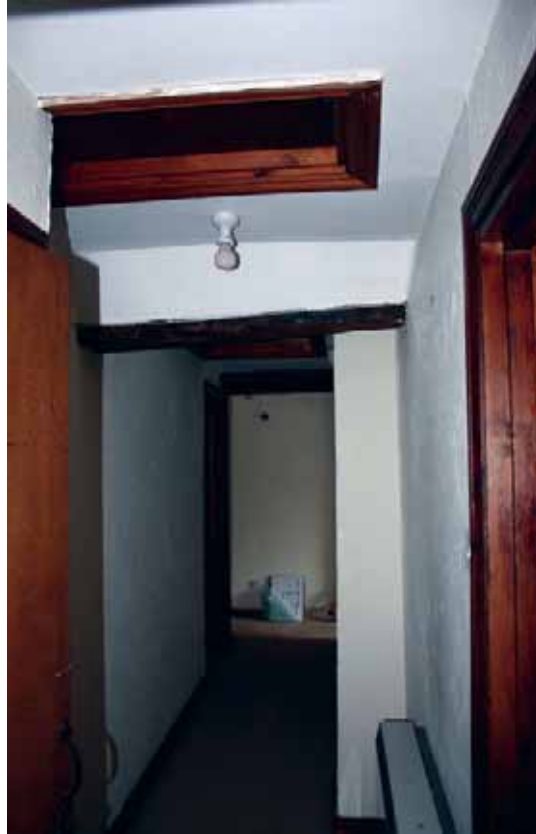
Plate 64: View along first floor corridor, F6
