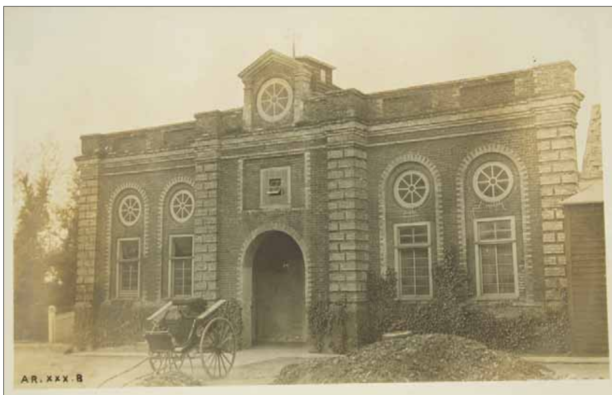
Figure 16: Photograph of Broadfield Hall Stables, 1910
