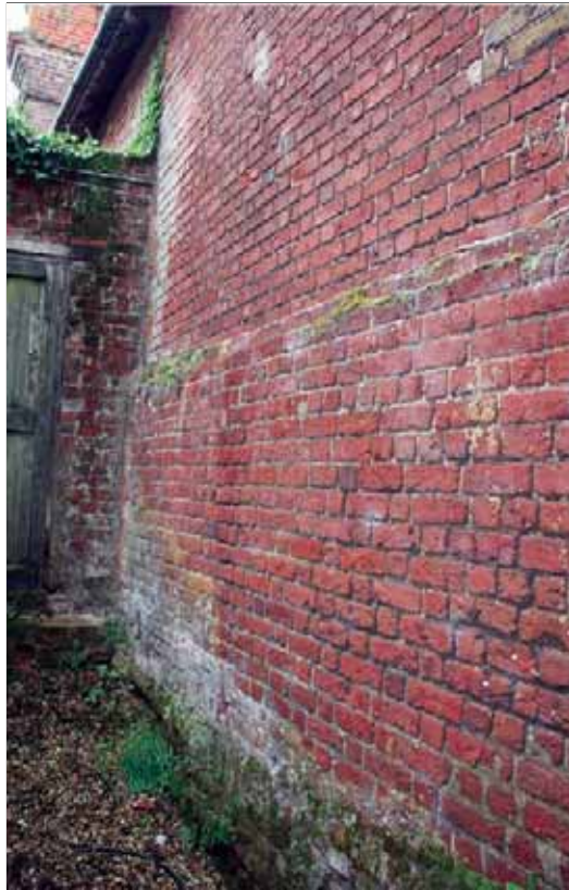
Plate 14: East-facing elevation on Hall Farm side of boundary wall
