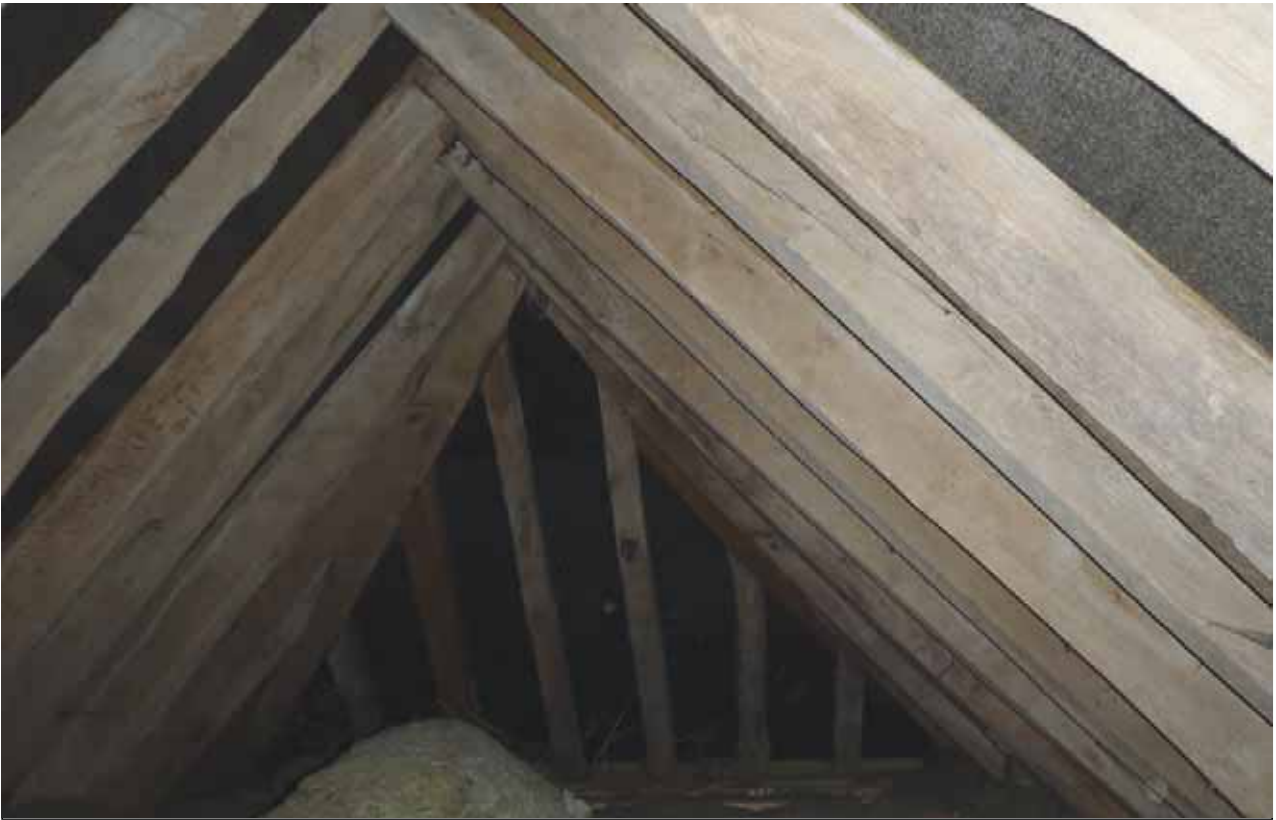
Plate 82: Hipped roof at northern end of roof space 2
