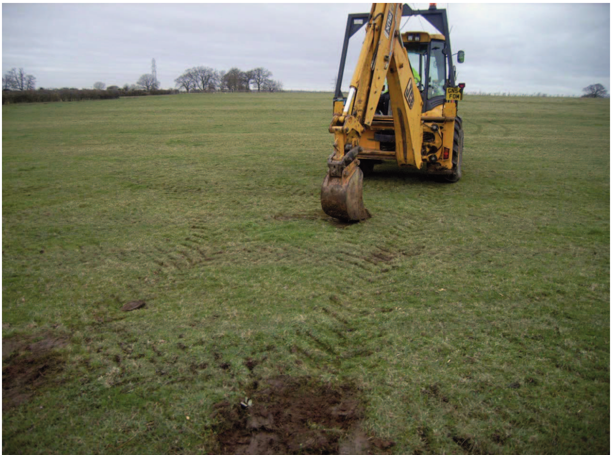
Plate 4: View N illustrating the limited surface disturbance adjacent to pole 11
