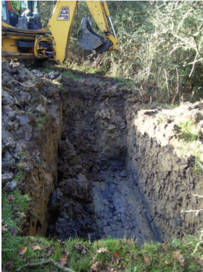
Plate 5: Replacement pole 48 excavated trench
