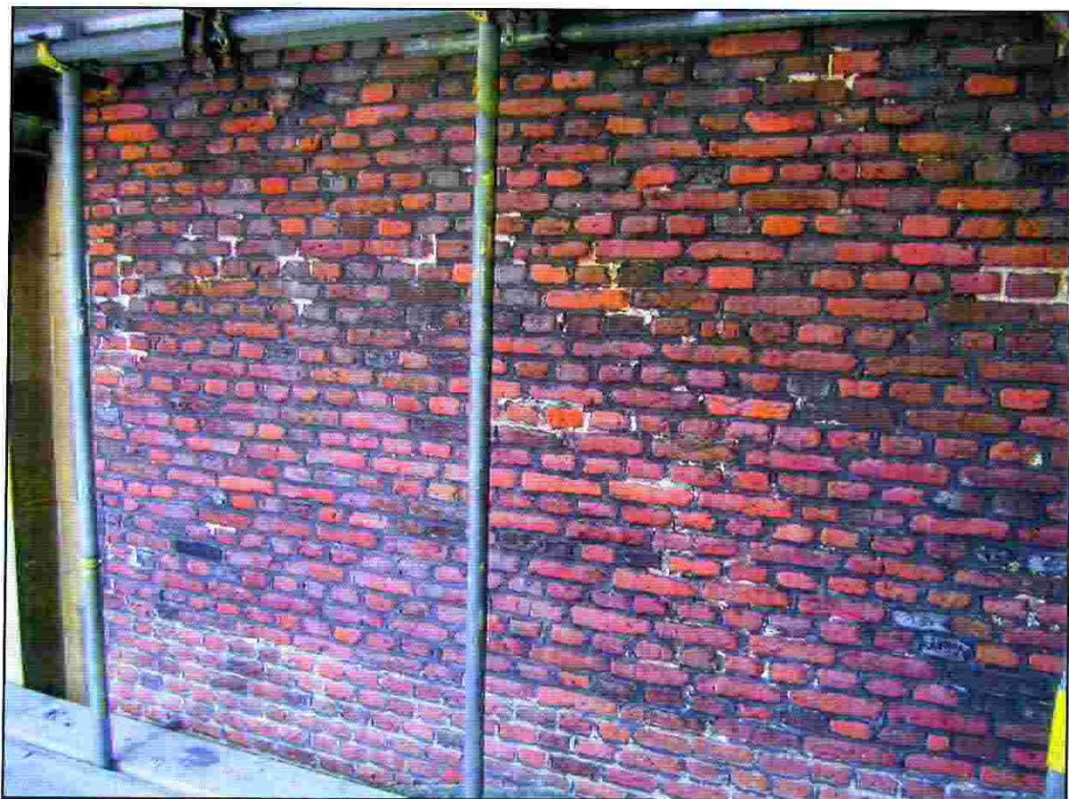
Plate 5: Chapel Court, North Facing Elevation - Test panel prior to raking out
