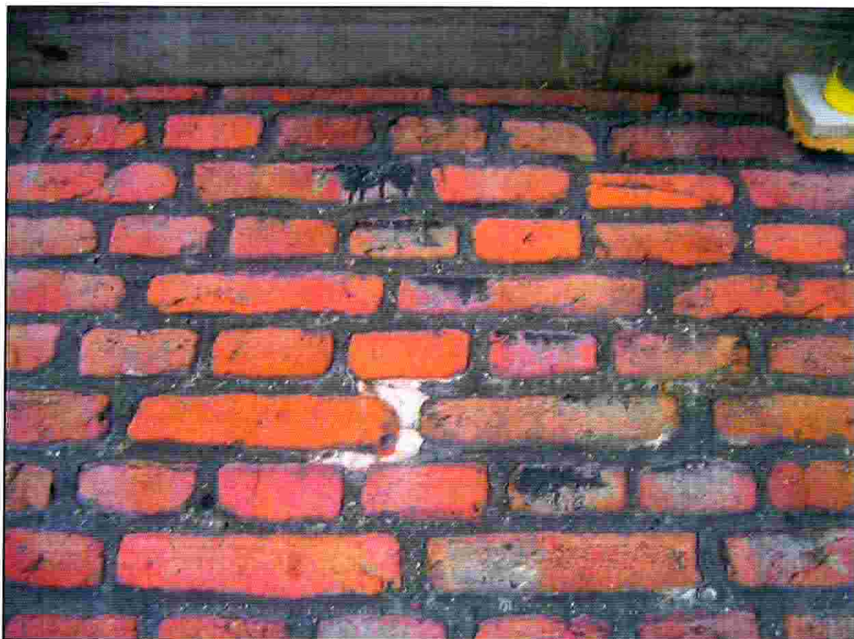
Plate 10: Chapel Court, North Facing Elevation - Black paint roughly applied
