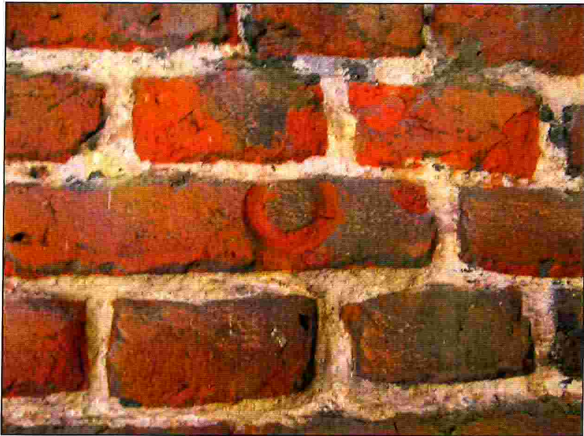
Plate 11: Chapel Court, North Facing Elevation - 20th century scaffold mark
