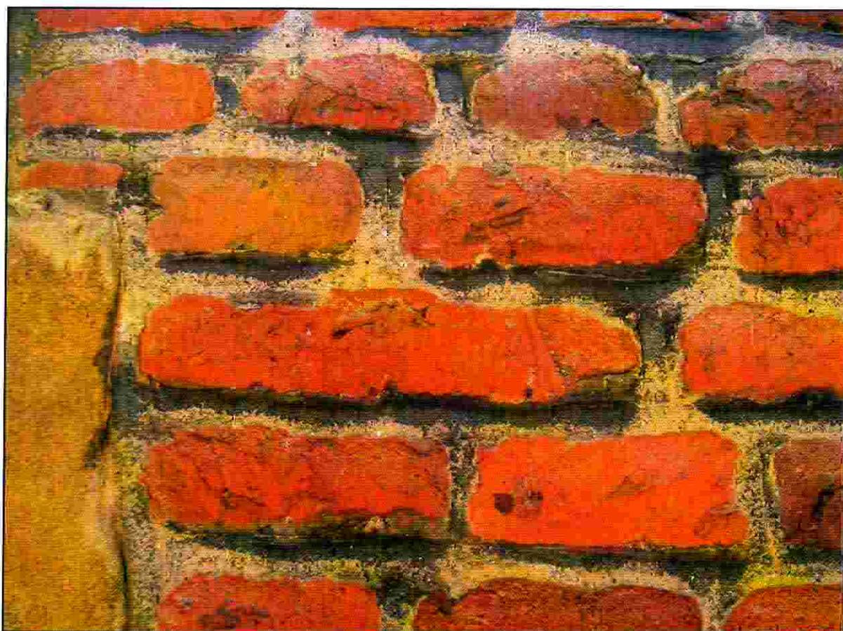
Plate 4: Chapel Court, North Facing Elevation - The painted mortar
