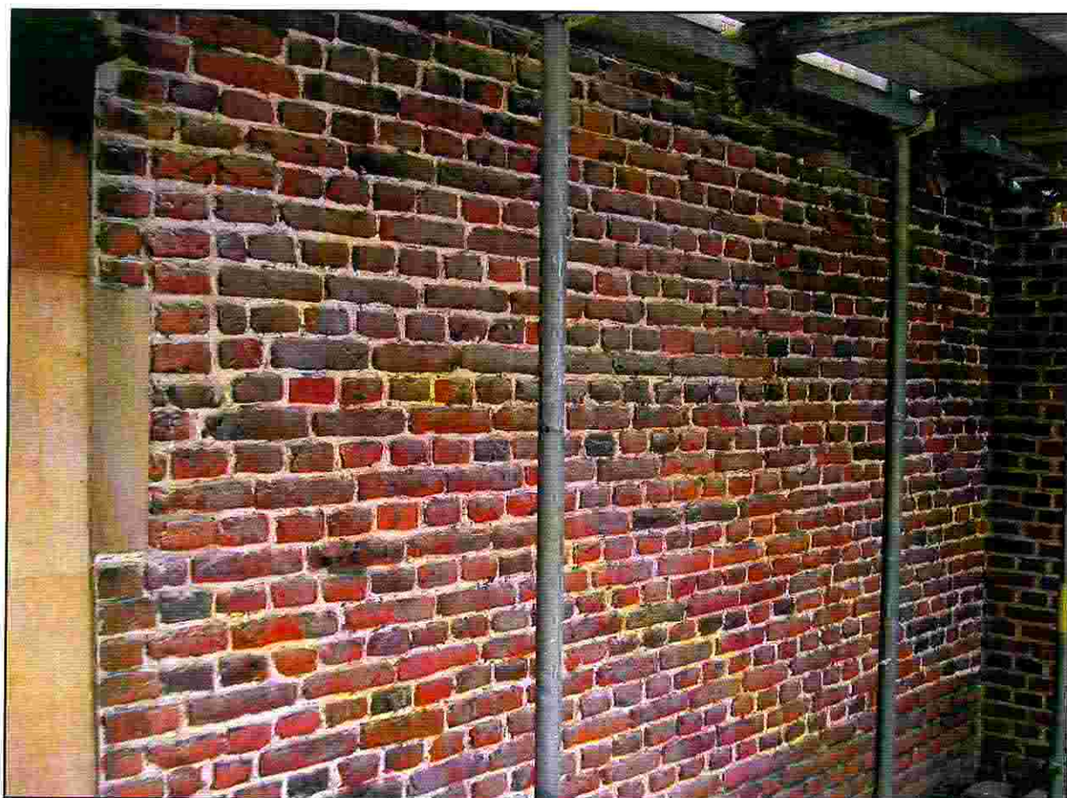
Plate 6: Chapel Court, North Facing Elevation - Test panel after raking out
