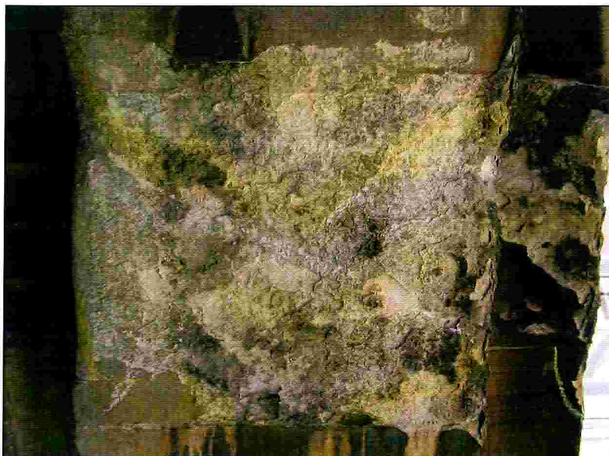
Plate 18: Chapel Court, North Facing Elevation - Blistering on lower pilaster stonework
