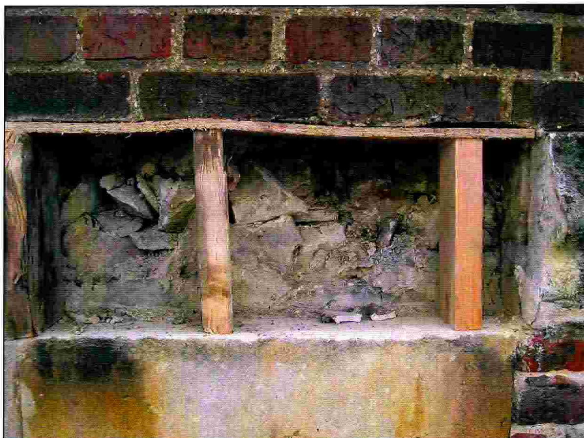
Plate 24: Chapel Court, North Facing Elevation - Brickwork and fill from behind upper string course stonework
