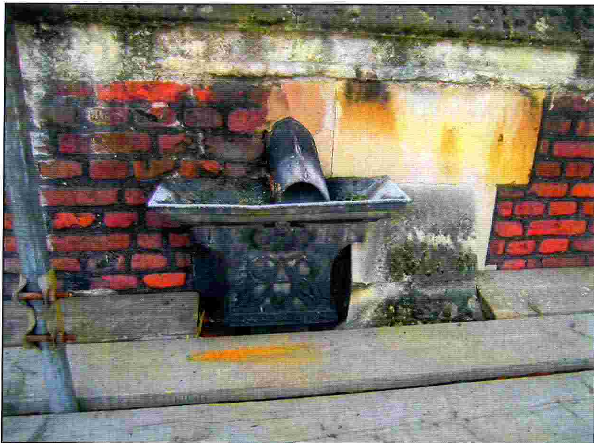
Plate 12: Chapel Court, North Facing Elevation - 1711 hopper
