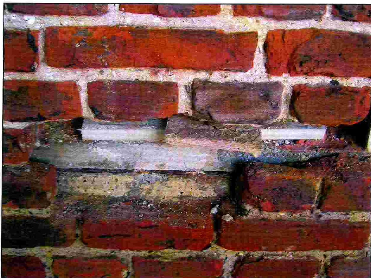
Plate 22: Chapel Court, North Facing Elevation - Concrete lacing piece located behind window insertion brickwork
