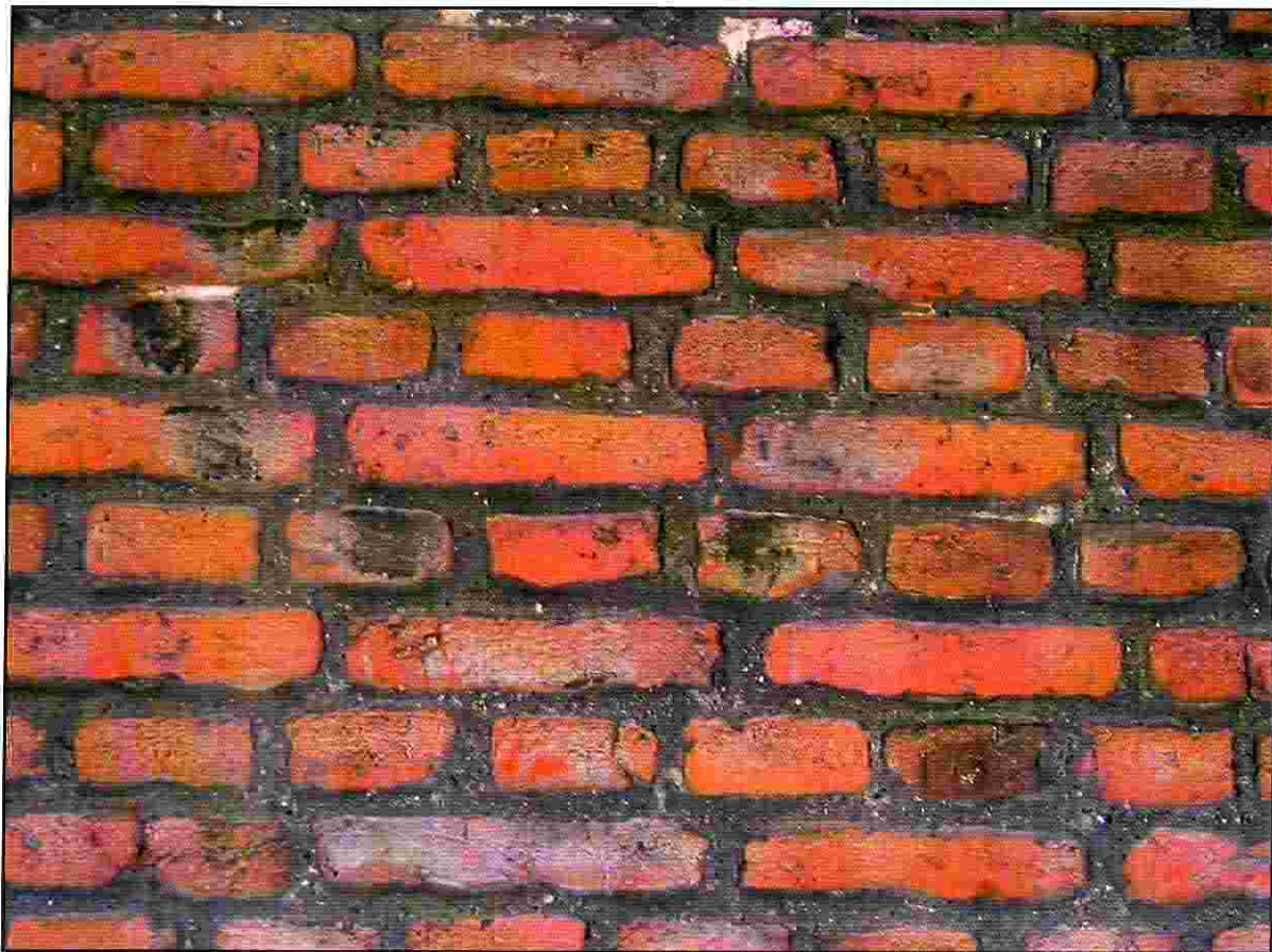
Plate 9: Chapel Court, North Facing Elevation - Diaperwork
