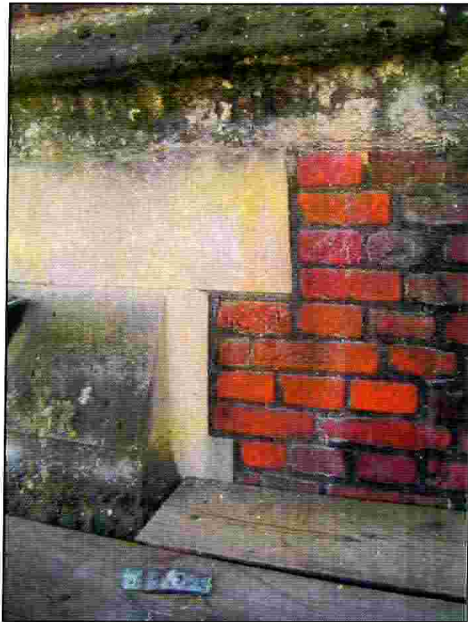
Plate 15: Chapel Court, North Facing Elevation - 19th century new brick repairs beside replaced stonework
