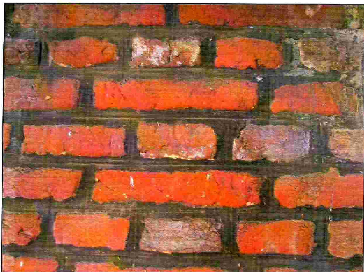
Plate 3: Chapel Court, North Facing Elevation - The black ash mortar
