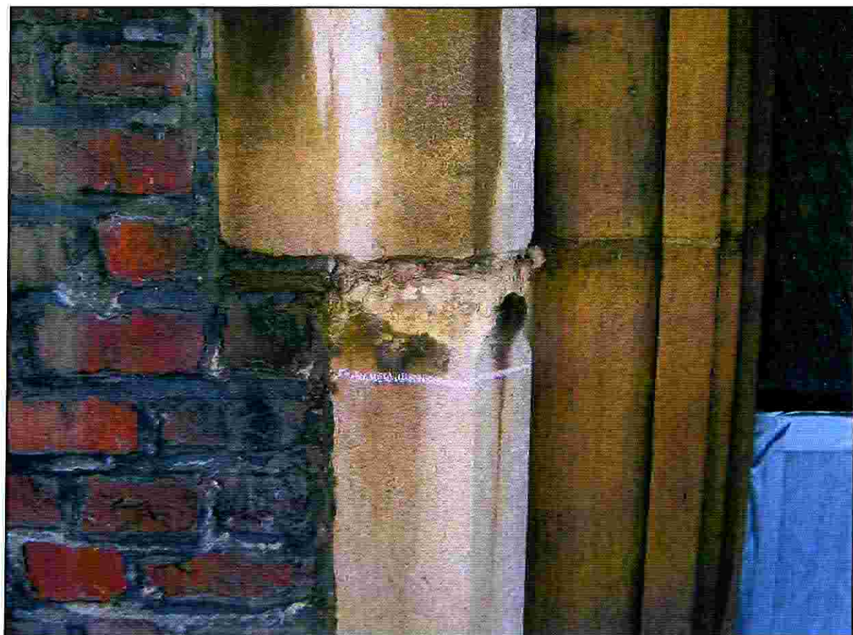
Plate 17: Chapel Court, North Facing Elevation - Blistering on window stonework
