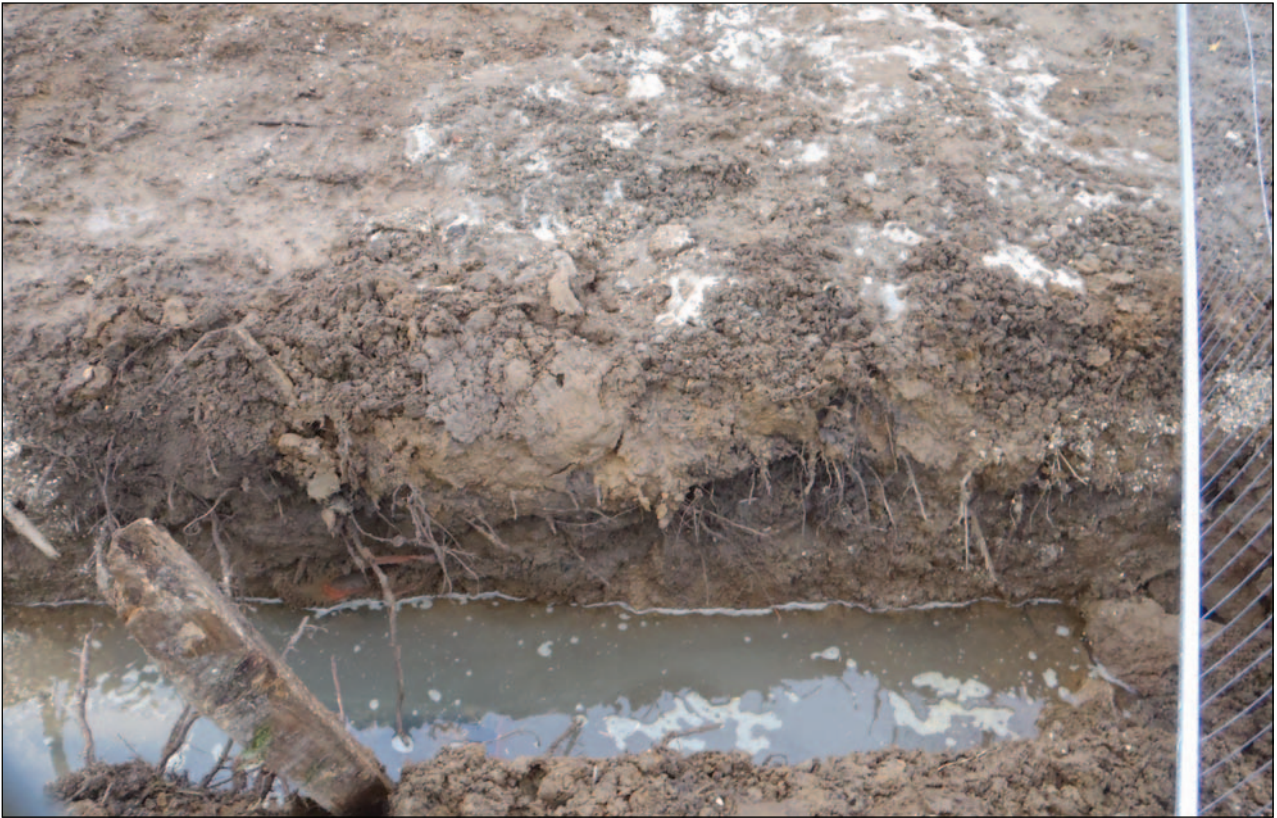
Plate 1: Working shot of service trench being excavated. Palaeochannel visible in section.
