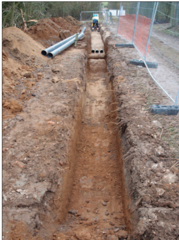
Plate 2: Working shot of service trench excavated through farm trackway.
