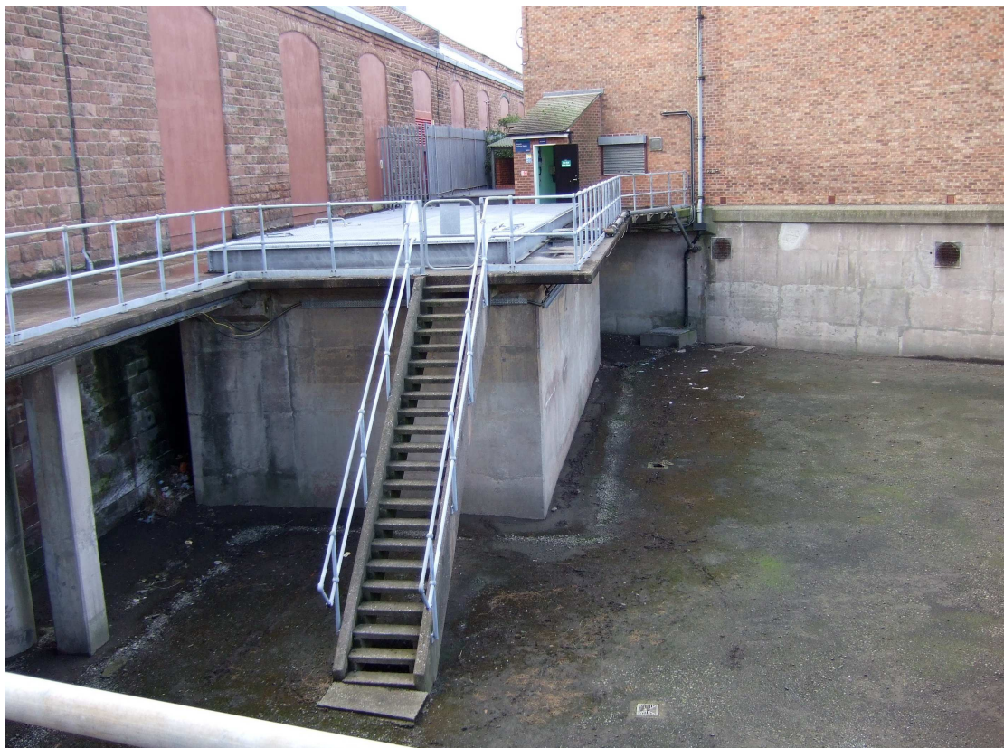
Plate 10: Detail of tidal flap chamber against the southern side of the dock
