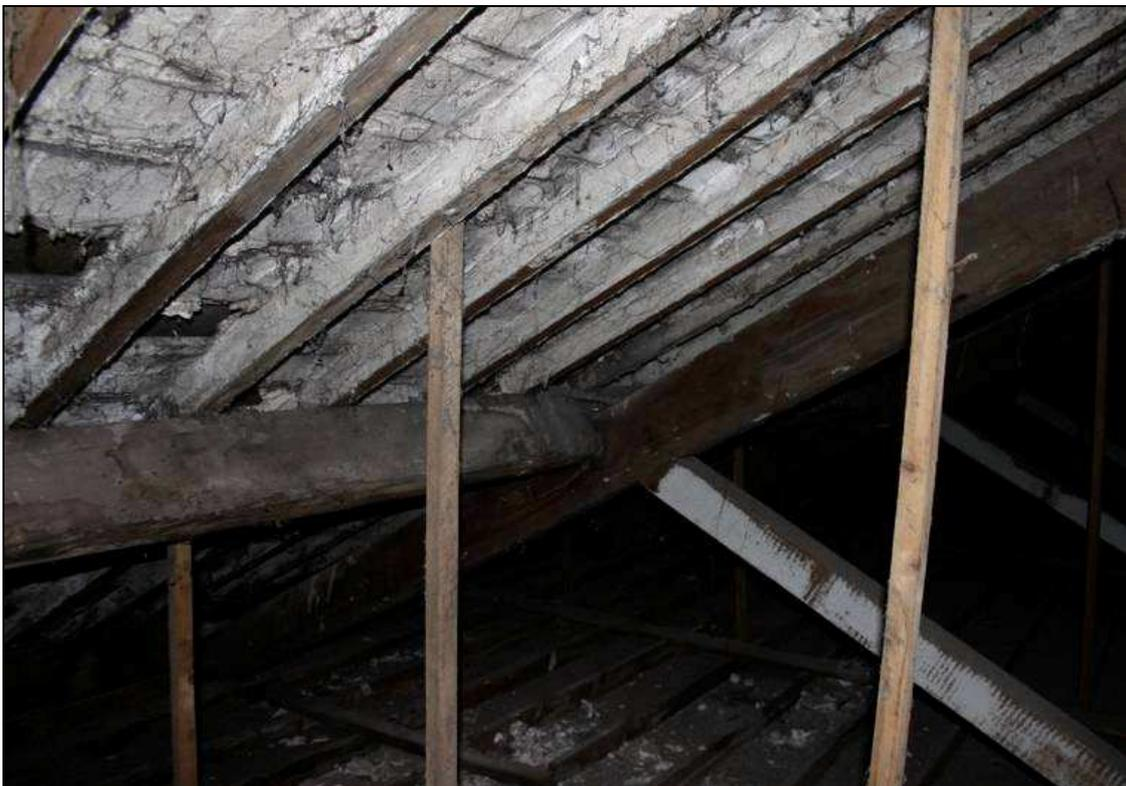
*Plate 20: Roof purlins and slate roof undersealed with whitewash*
