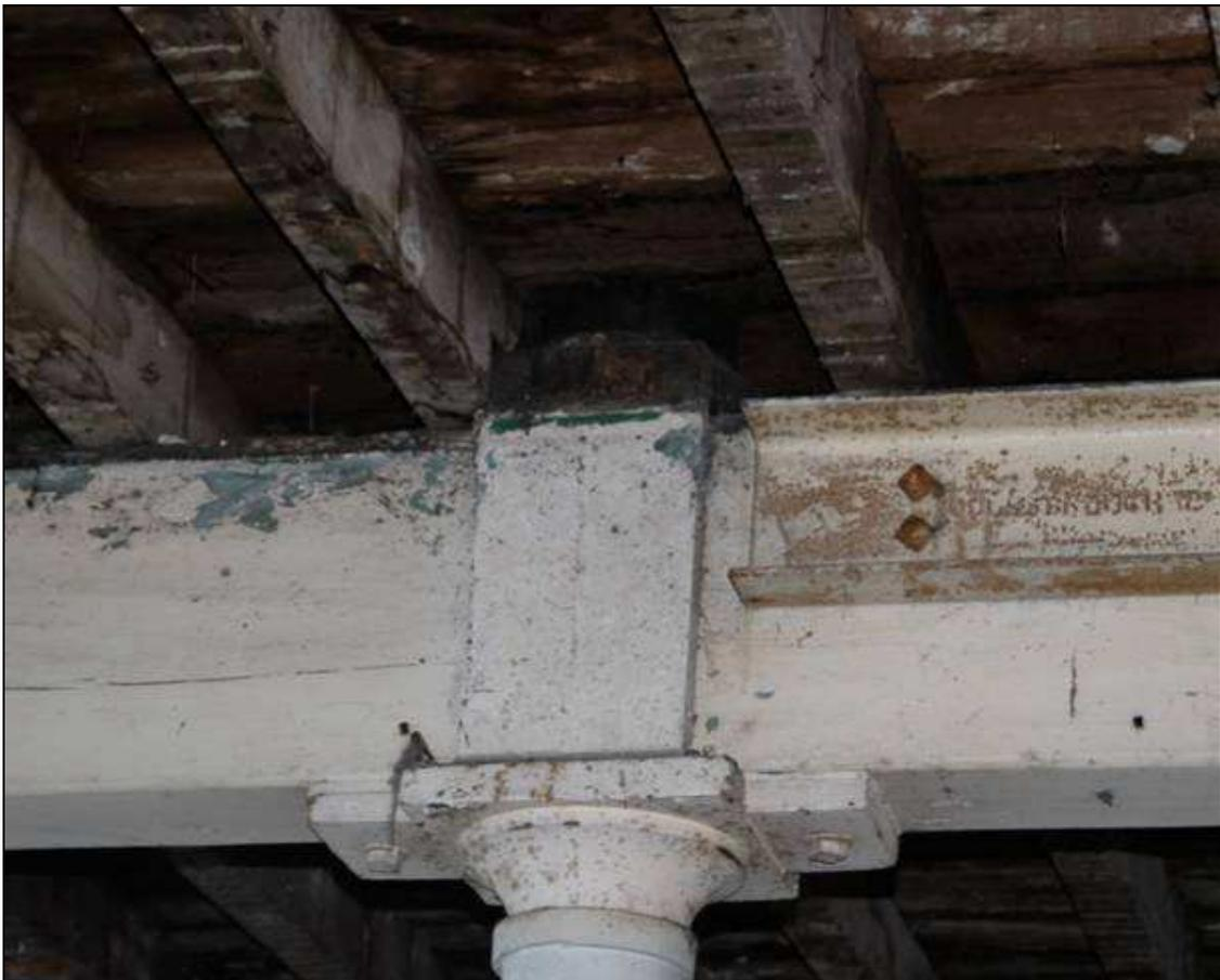
*Plate 17: Example of a crush box attached to the head plate of a column*
