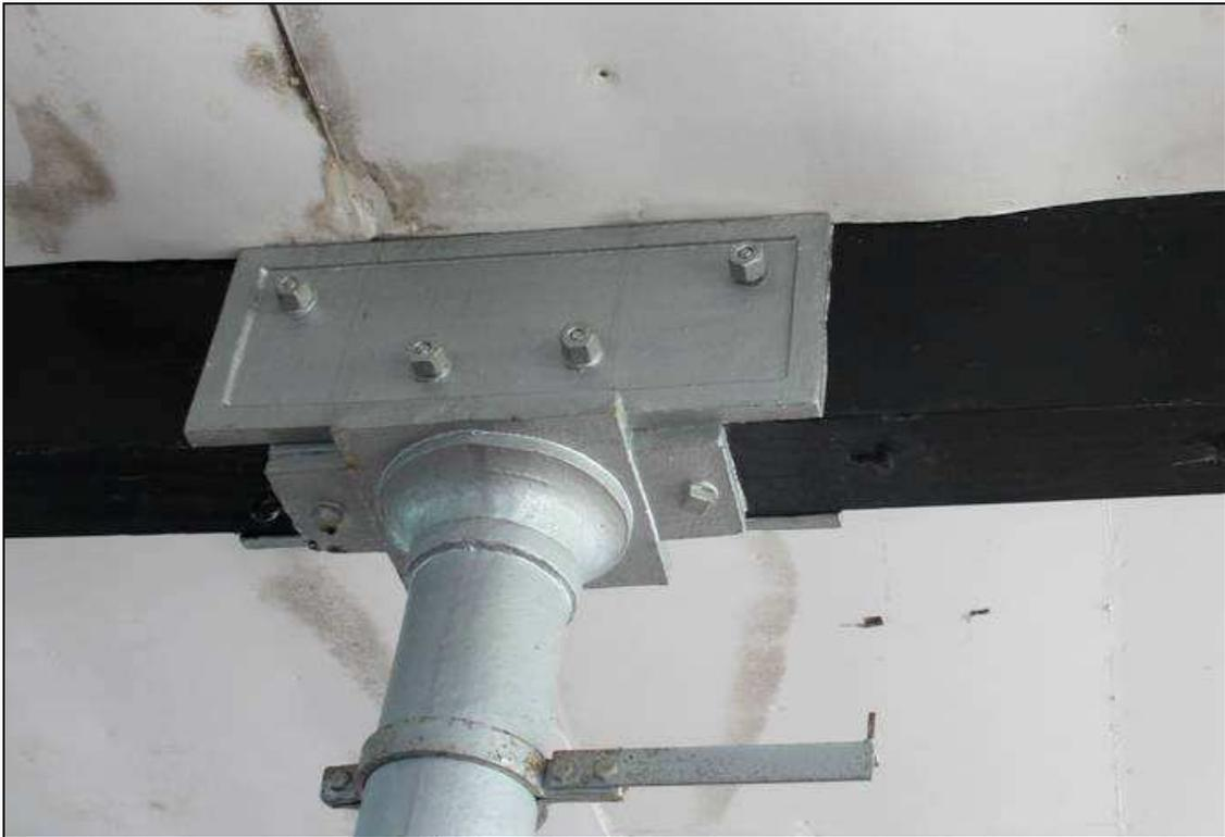
*Plate 16: Column capital and bolting arrangement on a fourth-floor column*
