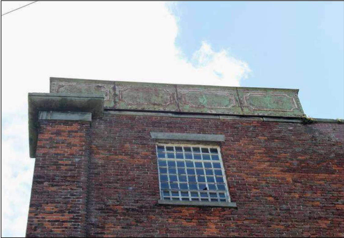
*Plate 11: Cast-iron water tank*
