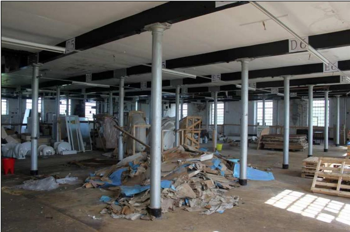
*Plate 19: Columns on the ground floor, showing line shaft hanging brackets*
