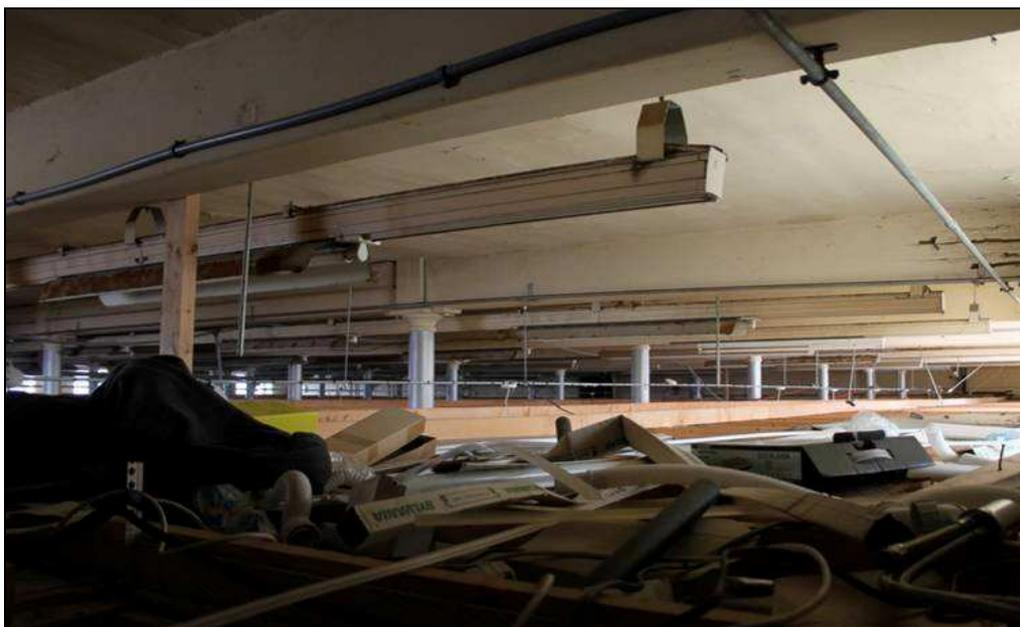
Plate 22: Top of the columns rising above modern suspended ceiling on the ground floor
