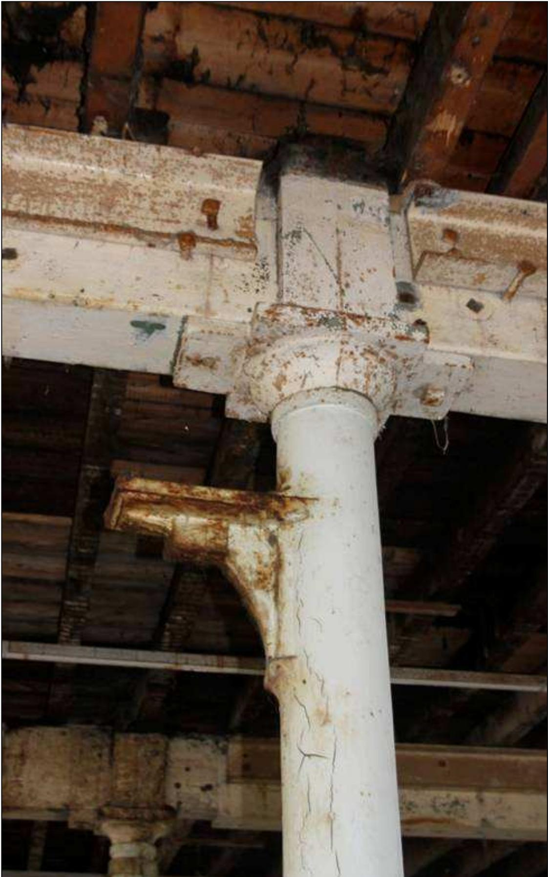
*Plate 18: Example of a line shaft hanging bracket*
