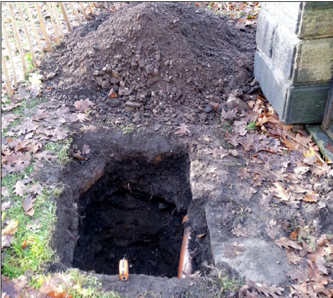
Plate 8: General view across Trial Pit 2
