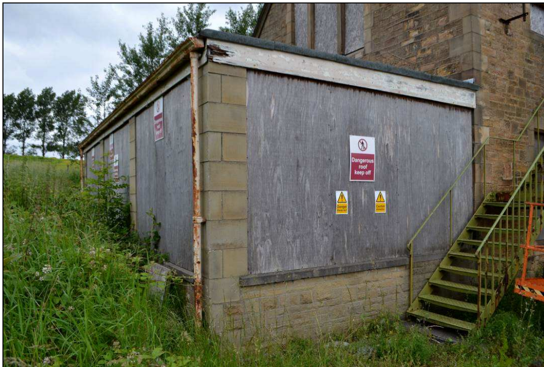
Plate 9: Southern extension, facing west
