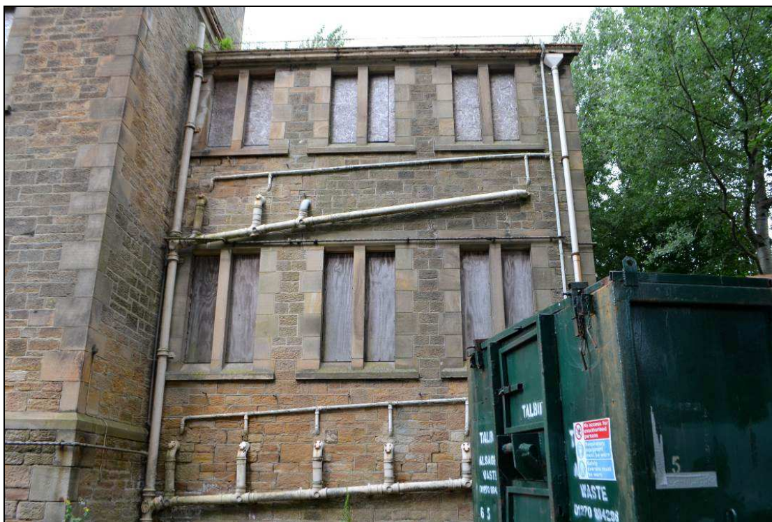
Plate 10: Eastern elevation of north-eastern wing, facing west
