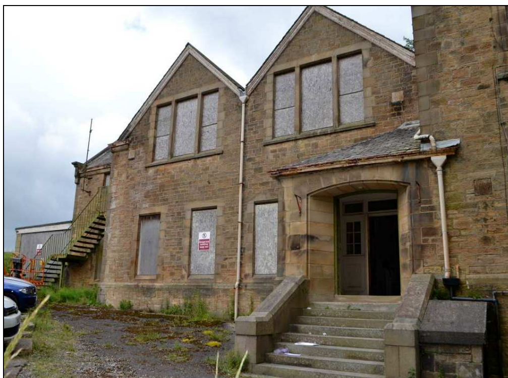
Plate 5: The stone steps leading up to the main entrance
