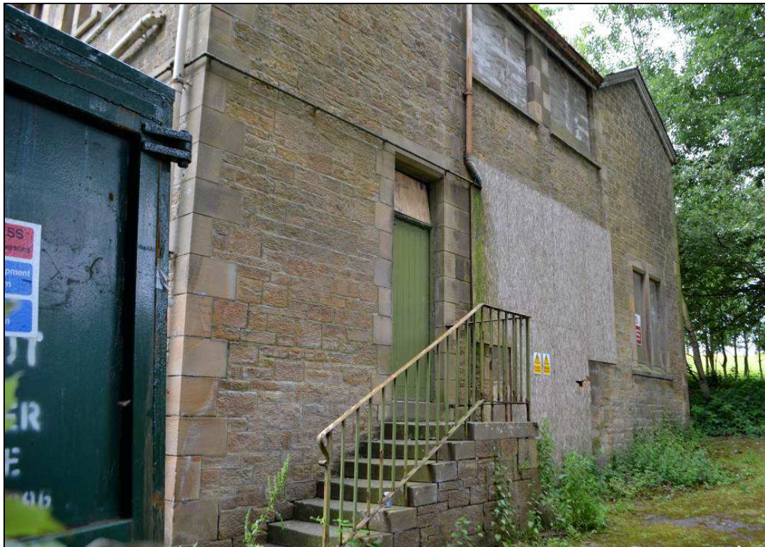
Plate 8: Northern elevation, facing south-west
