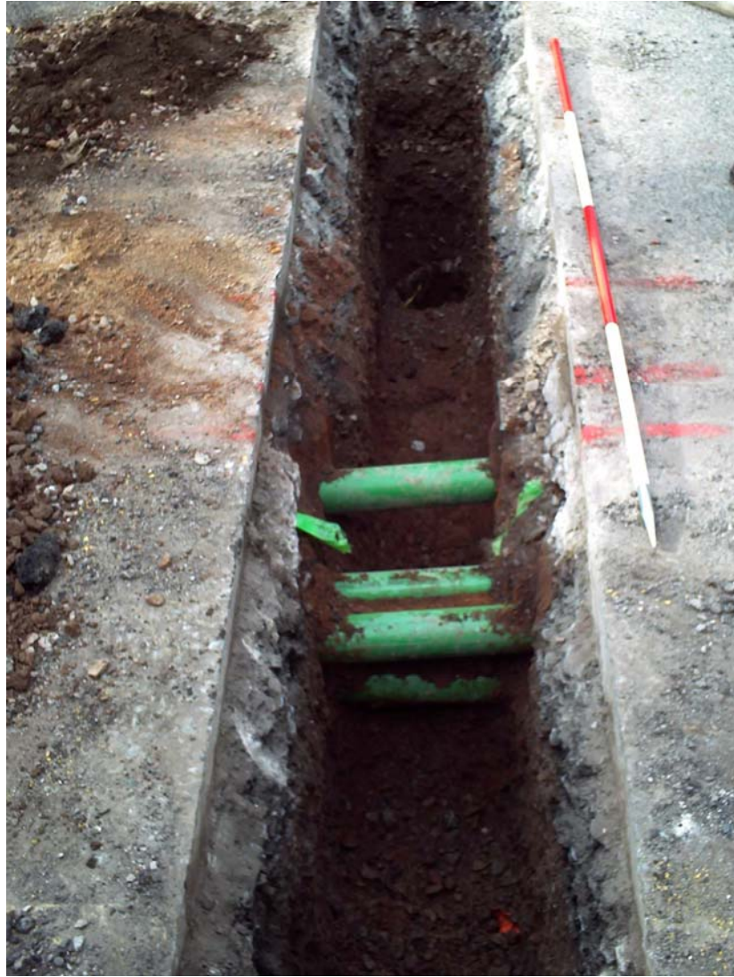
Plate 1: The trial trench facing west.
