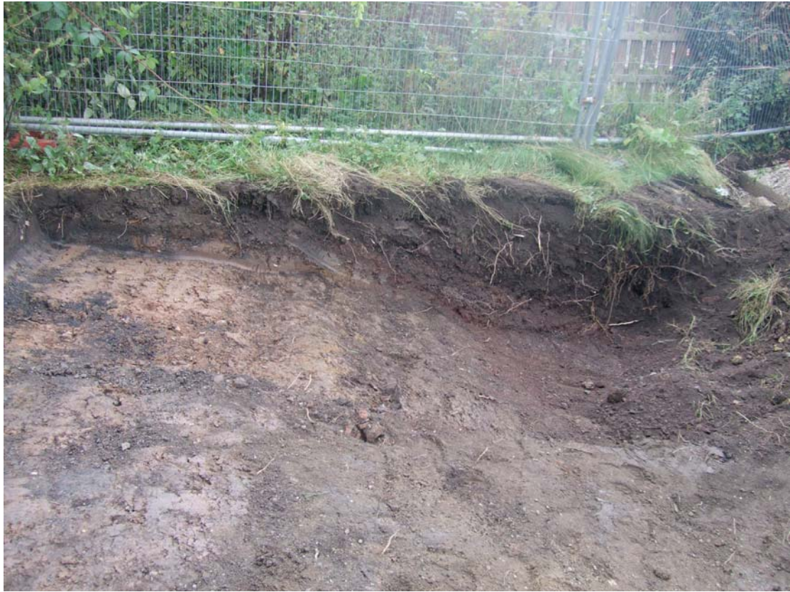
Plate 2: Detail shot of slightly deeper excavation at the northern end of the trench, showing the later levelling material (2) sealing the profile of the embankment (3)
