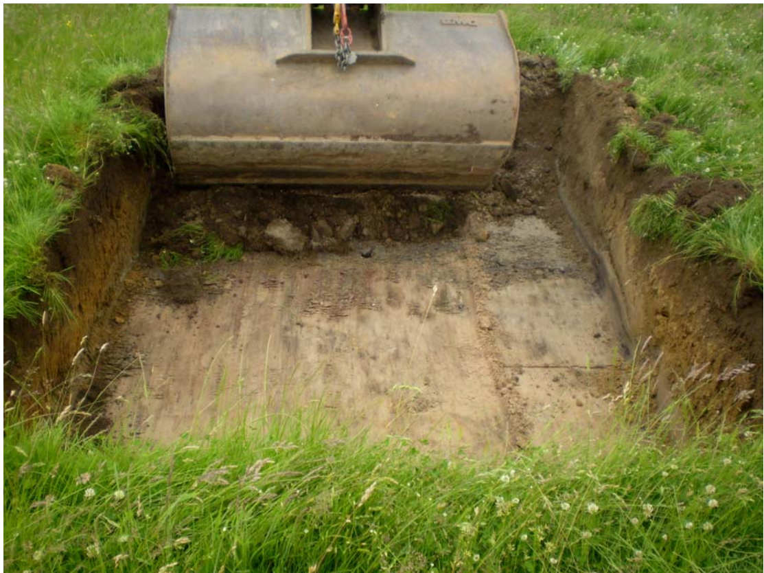
Plate 2: (Field 24) Excavation of directional drilling pit 24A
