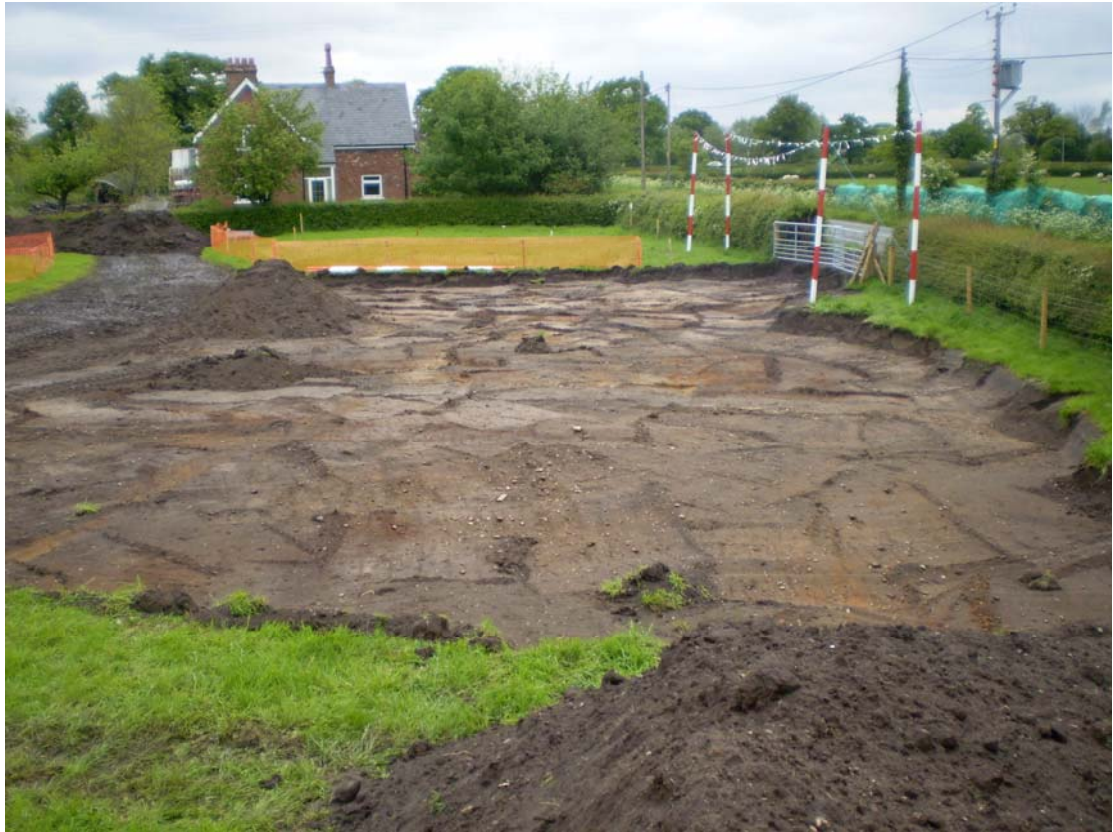
Plate 1: (Field 17) Area topsoil strip to create Delivery Zone E
