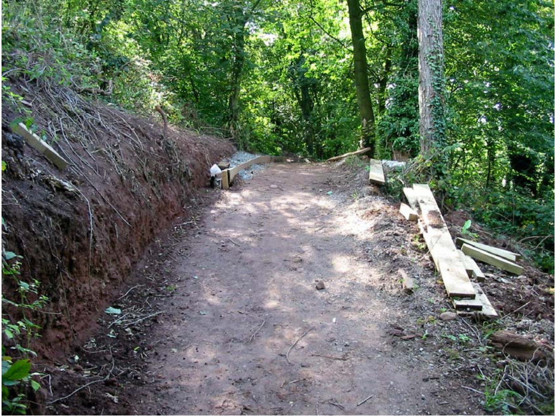
Plate 7: General shot of path after old surface removed
