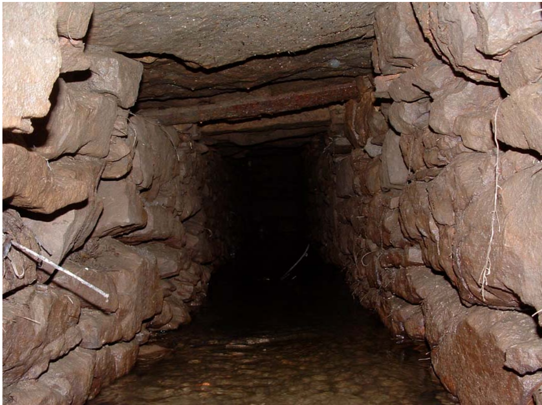
Plate 4: South-east-facing view inside culvert
