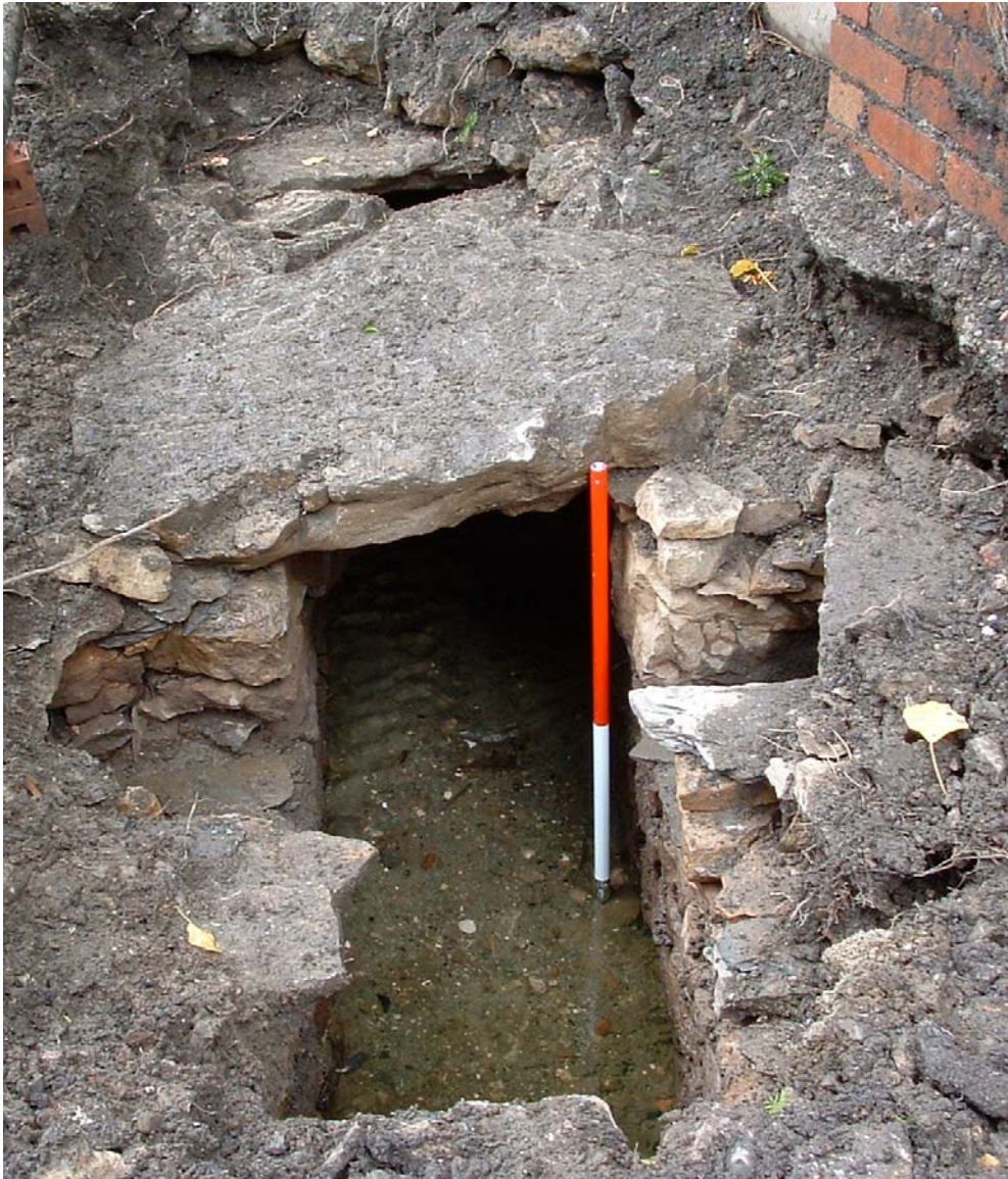
Plate 1: South-east-facing view of culvert
