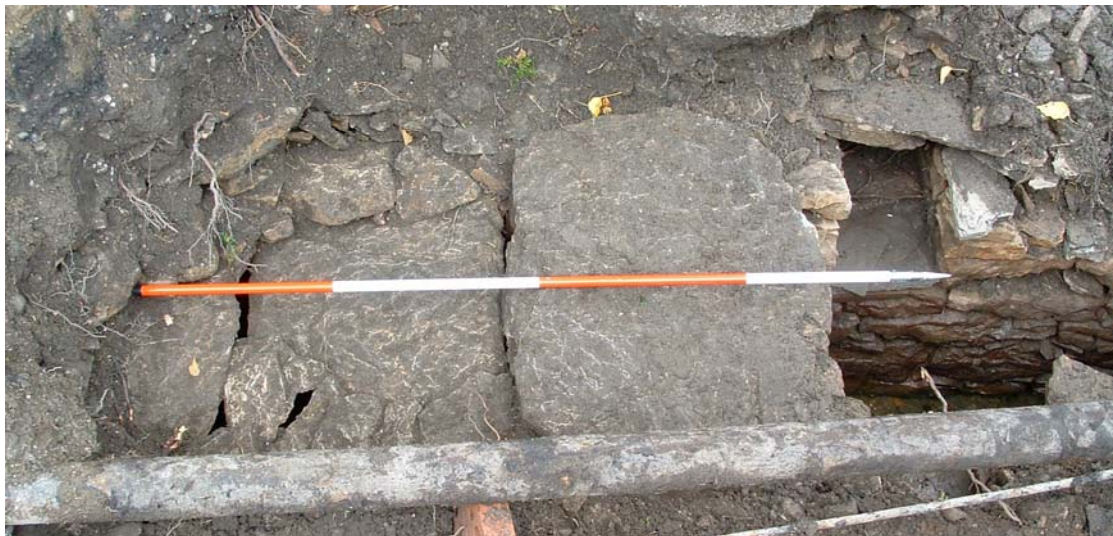
Plate 2: South-west-facing view of culvert
