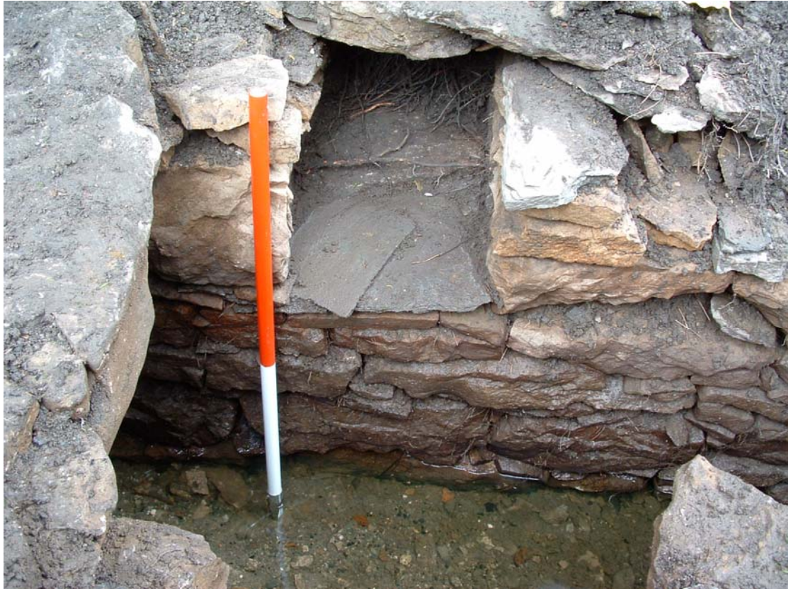
Plate 3: South-west-facing view of southern side culvert
