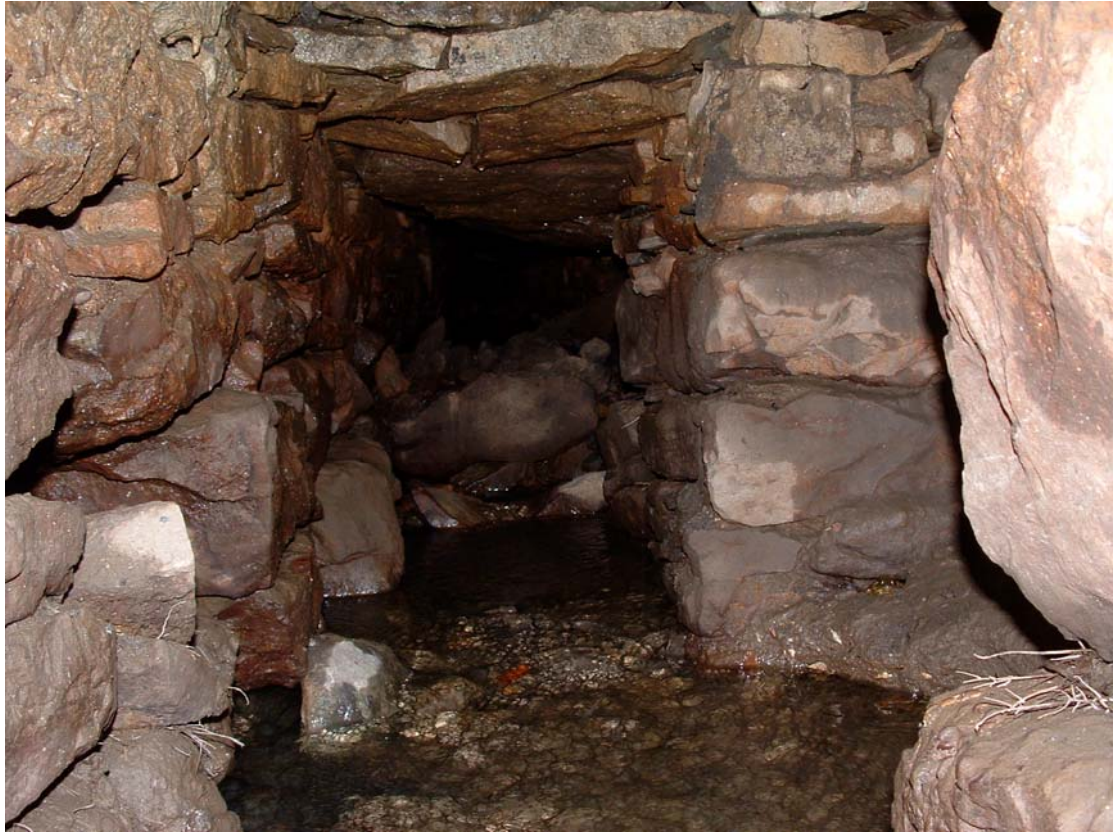
Plate 5: North-west-facing view inside culvert
