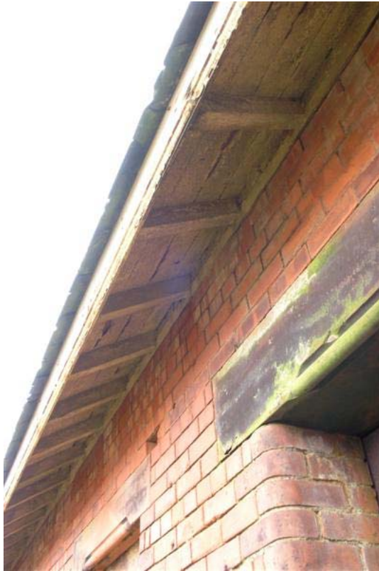
Plate 7: Projecting rafters below eaves
