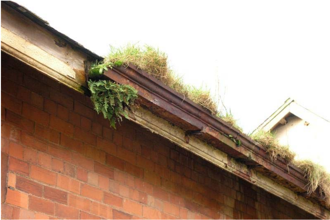
Plate 9: Cast iron gutter on east side
