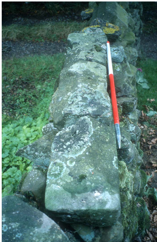
Plate 2: Detail of broken stone stoop in wall
