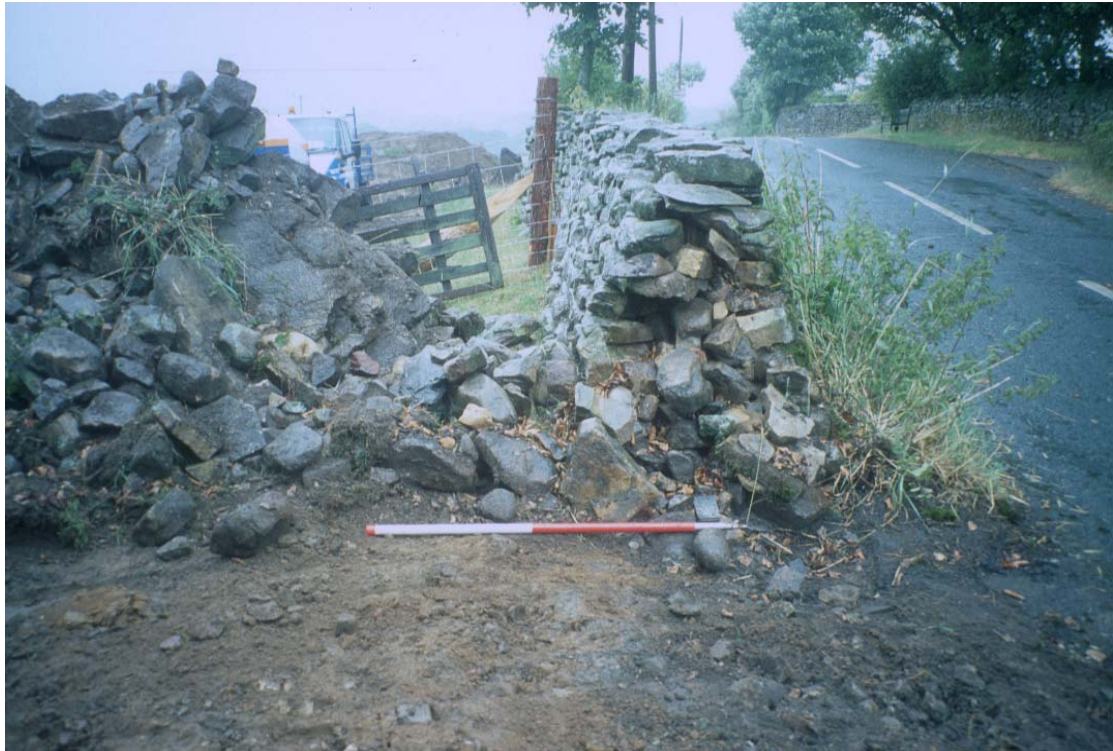
Plate 4: Section through drystone wall Field 1, facing north
