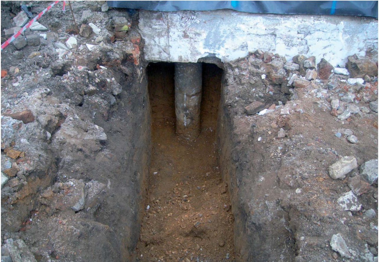
Plate 5: Underpinning trench, showing pile foundation
